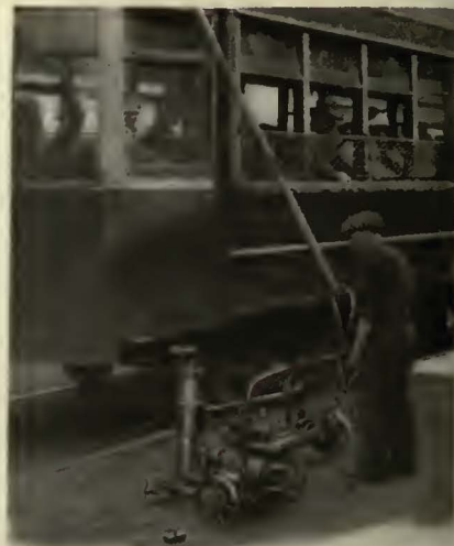
Grinding wheel arm swings aside to pass cars without removing trolley pole.
