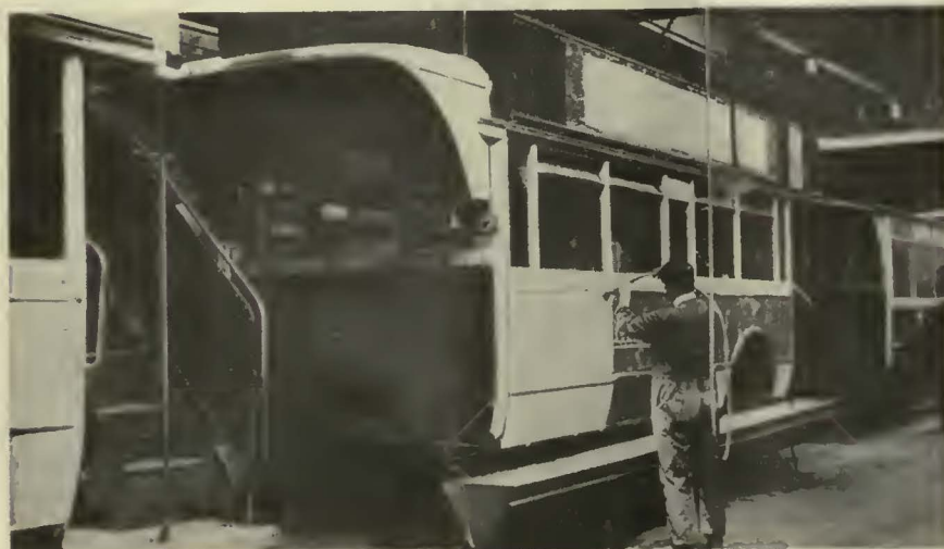
Bus bodies up to the waistline are painted by the flow method in the shops of the London General Omnibus Company. Only about one minute is required to paint each side. Paint is applied through a hose or by a can
