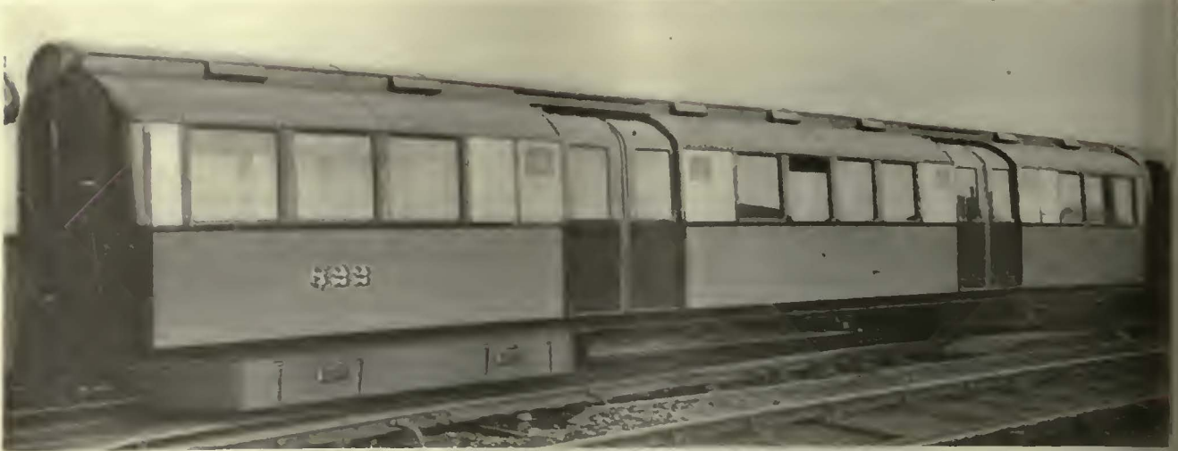
A "skirt" of ferrodo was built around the trucks of the London tube cars to confine the noise
