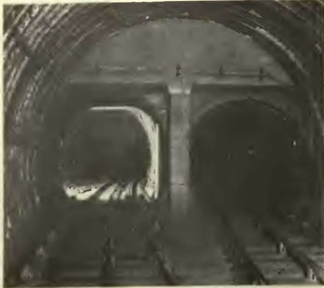
The London tubes are tubes in fact as well as in name. Larger diameters are used at junction and stations
