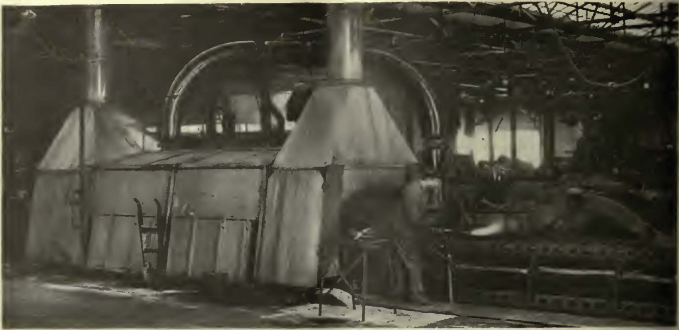
In London steaming is used for cleaning many of the large car and bus parts in the overhaul shop
