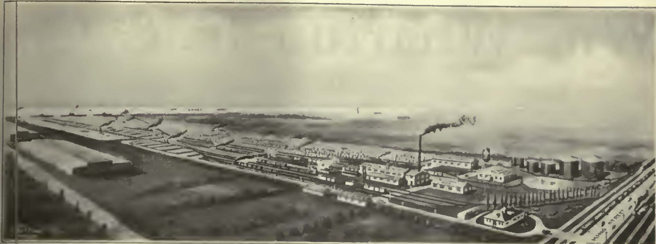
Bird's eye view of Plant and Storage yard.
