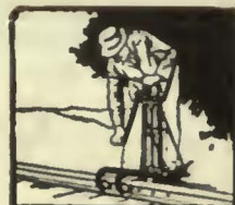
Track and Bonding Drill
