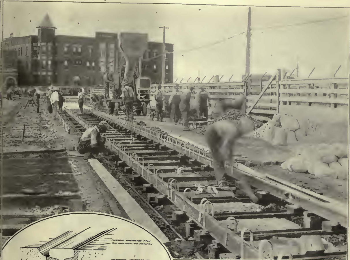
Installing Serviced Rail Filler, Sioux City, Iowa
