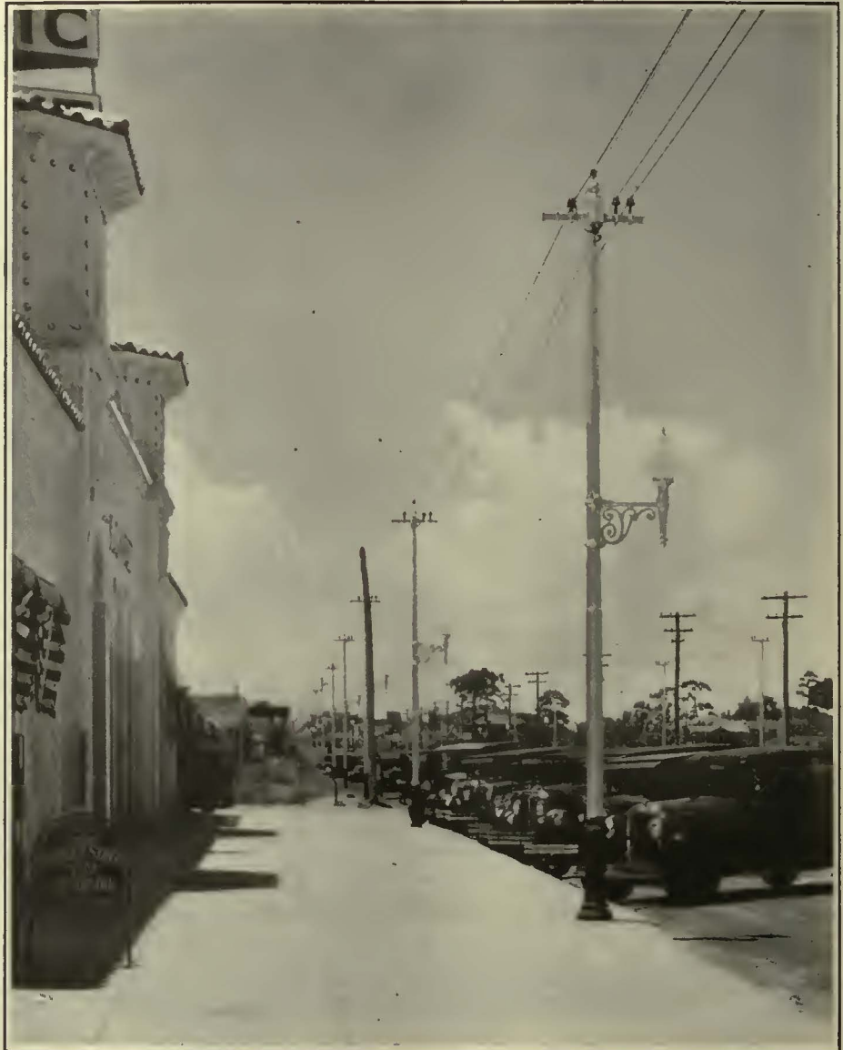
"Elreco" Combination Railway and Lighting Poles, St. Petersburg, Florida. Note contrast between new "Elreco" poles and old wooden poles about to be removed.
