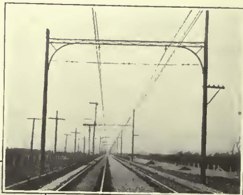
Bates-Truss Expanded Girders which are used over many miles of the “South Shore’s” right of way, relieve the wood poles of the steady strain of the span wires.
