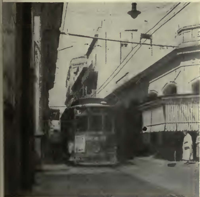
At Camaguey the local electric railway uses single overhead trolley wire. Span wires are often attached to buildings in these narrow streets
