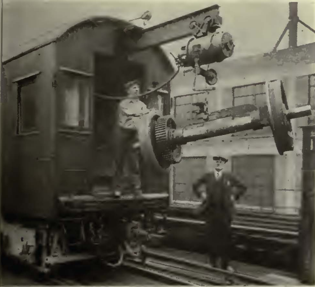
Lifting a pair of wheels by means of the air hoist
