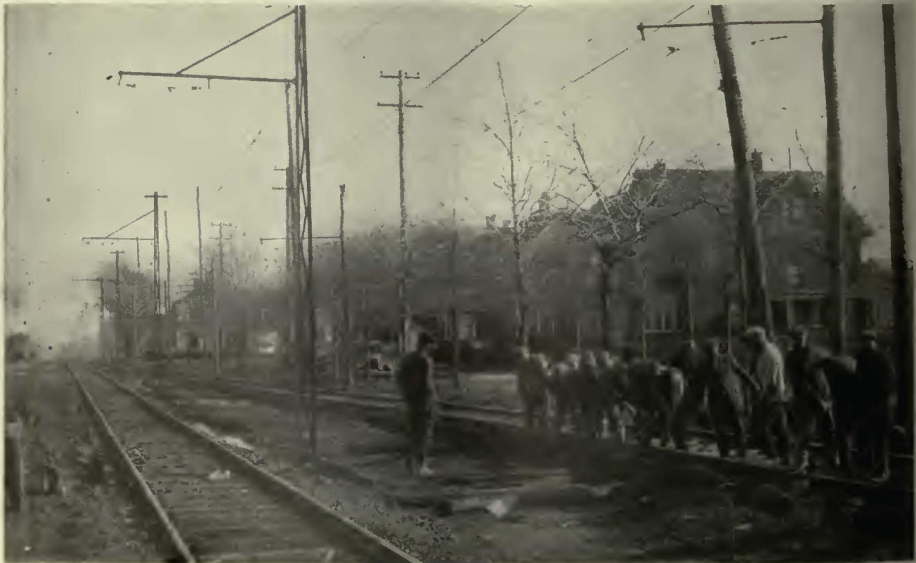
Erie Railway's tracks relocated on East Lake road without any service interruption. Temporary track being shifted to permanent location
