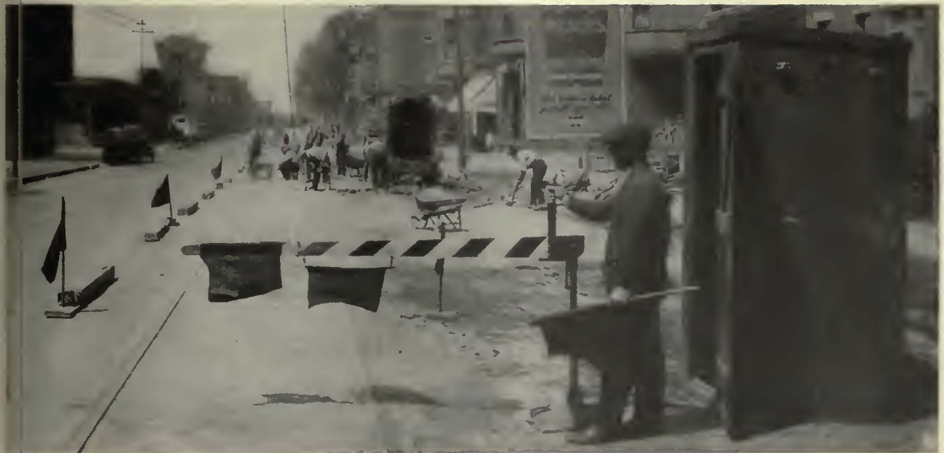
Precautions taken by Chicago Surface Lines to protect track workmen in the streets. The simple safety gate blocks the work area effectively
