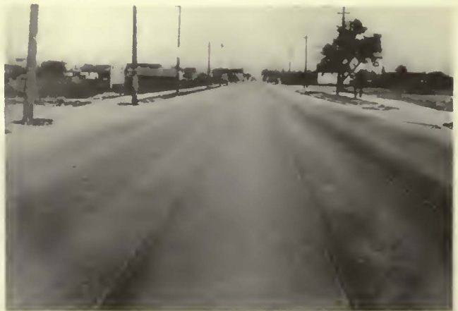
Modern type of concrete paving on Michigan Avenue at 126th Street in Chicago. The rail was installed in 1912 and 1913. Paving was placed in 1924
