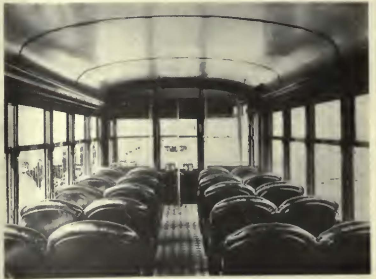
At left, view showing the observation type rear end with wide center window of Rockford cars. At right, interior view showing the one-level floor and the deep-cushioned individual type seats. Note the absence of dome ceiling lights
