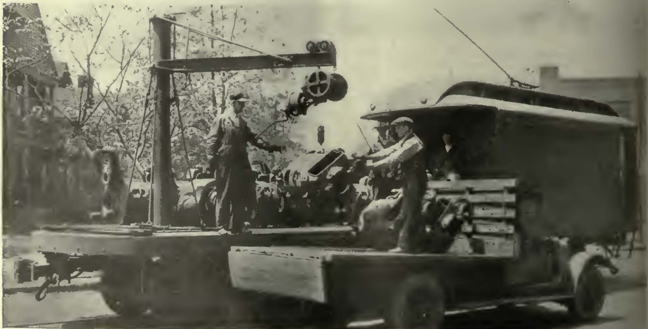
In transporting the motor to Cleveland small trucks and a supply car were used
