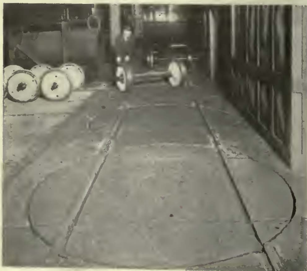
A feeder track with turntables connects the wheel storage tracks
