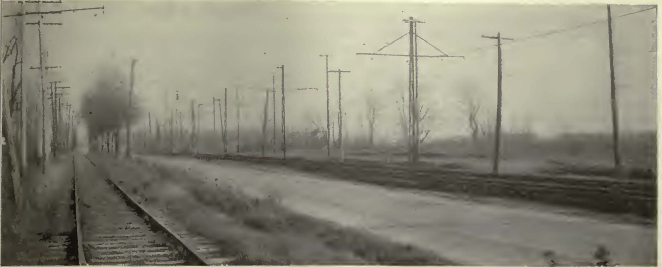
The new location of the tracks is on the private right-of-way in the center of the 120-ft. roadway, The old track at the left has been removed
