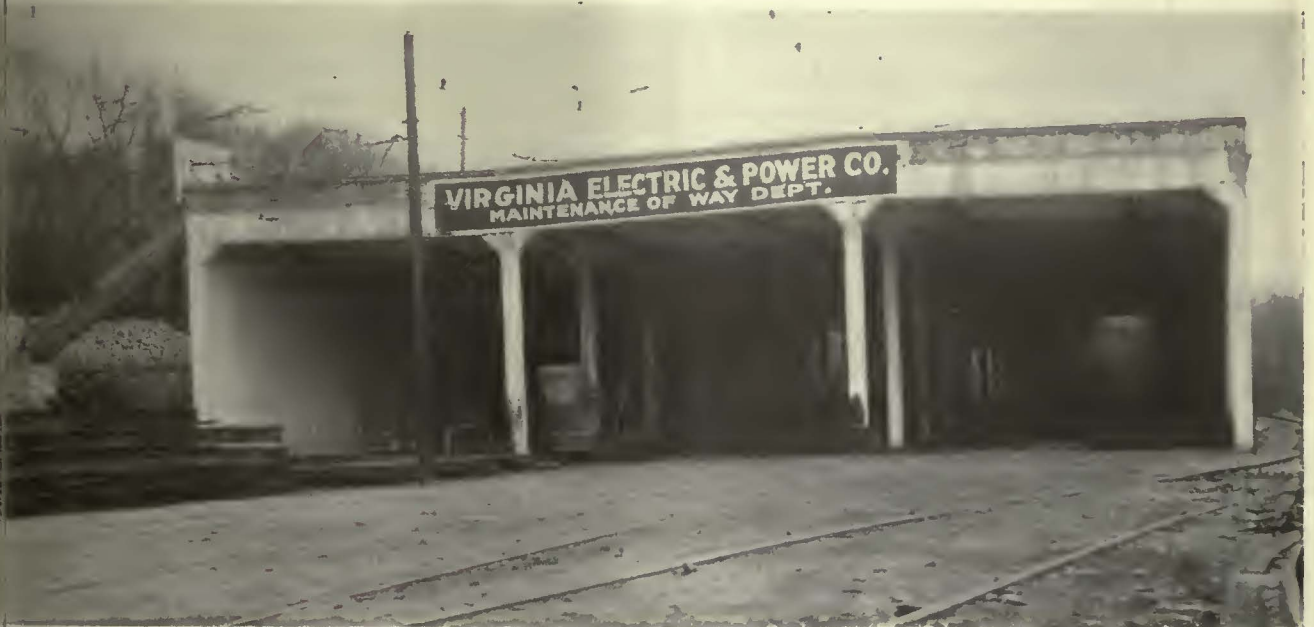
Plenty of room is provided for the storage of maintenance of way materials in this converted carhouse
