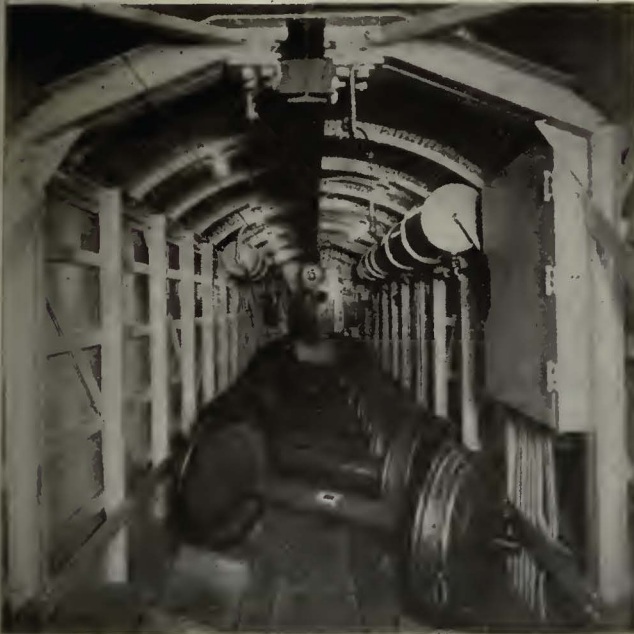
Interior of car showing air tanks on either side near the roof and supports for the I-beams of the air hoist
