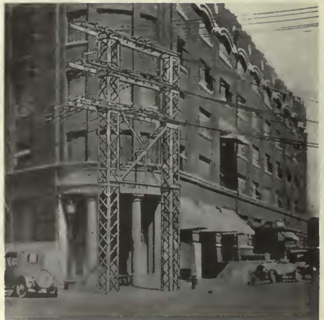
This tower replaced seven wooden poles in Fort Worth, Tex. It makes the power supply more reliable and improves the appearance of the street
