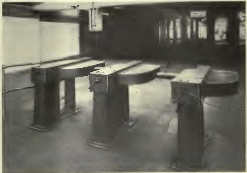
Battery of Perey non-electrical turnstiles installed in B.-M. T. subway station
