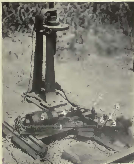
Northern Texas Traction develops derail for railroad crossings for use with one-man cars
