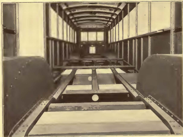
Three 7" steel channels act as sills, while deep stiff steel channels and angles comprise the floor beams. The T-shape pillars are also evident.
