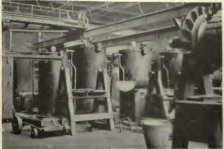
London County Council Tramways has fifteen impregnating tanks, each of which will hold an armature
