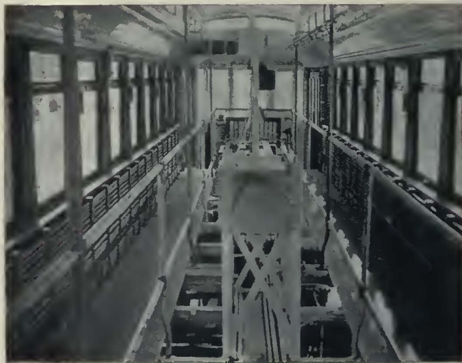
This old car has been fitted out for instruction purposes. The floor has been cut away to show the operation of the machinery. The wiring, air valves and other parts are also visible
