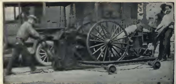
Reelocating Track Grinder
