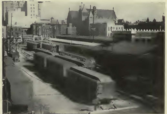
The passenger station and the adjoining flatroofed freight house are back of the transfer shed in this view
