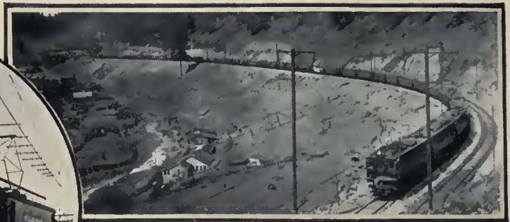
Operating Costs Reduced 45% on the Virginian Railway
