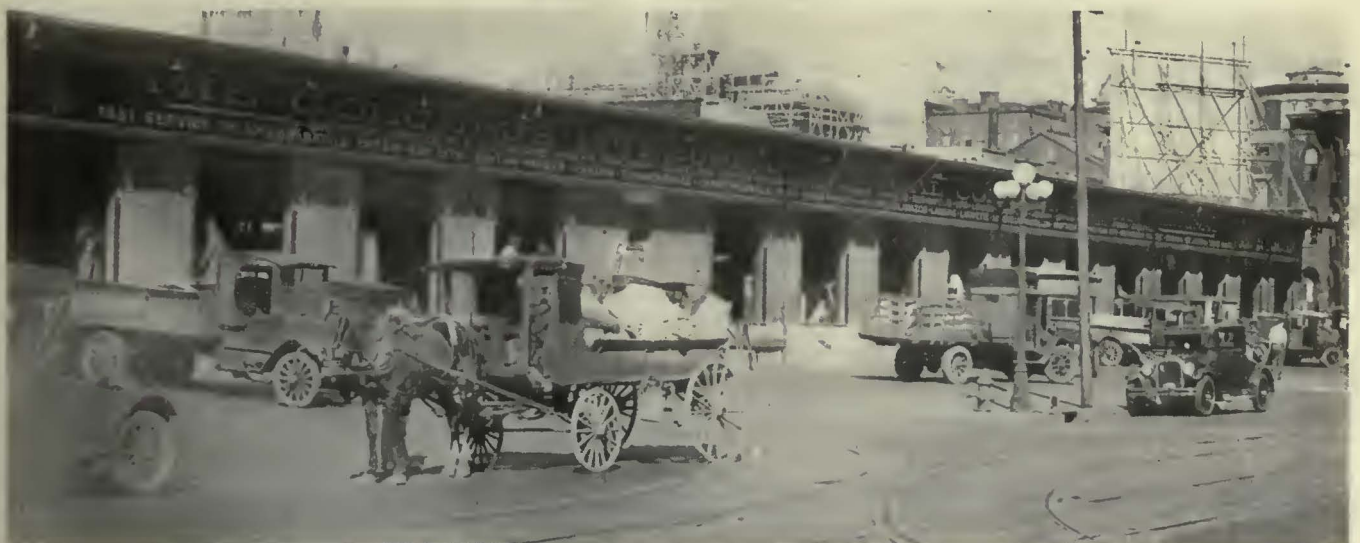
Seventeen service doors are provided in the present terminal for inbound and outbound freight
