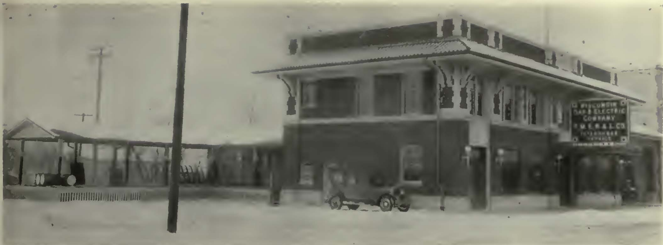
New terminal buildings at Burlington, East Troy and Watertown provide facilities for interchanging car and bus passengers under cover. This view of the Burlington station shows express platform at rear of building
