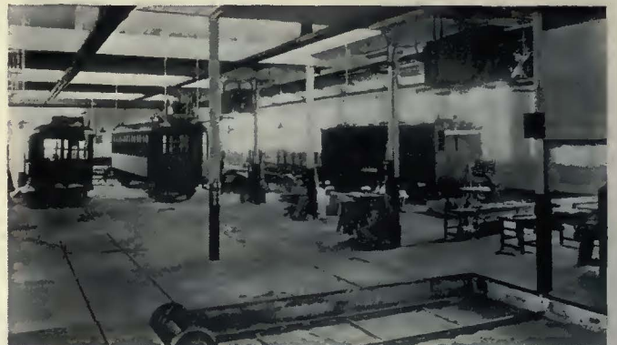
View of the woodworking shop from the transfer table
