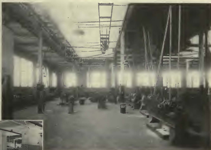
Machine shop, looking from the armature repair department
