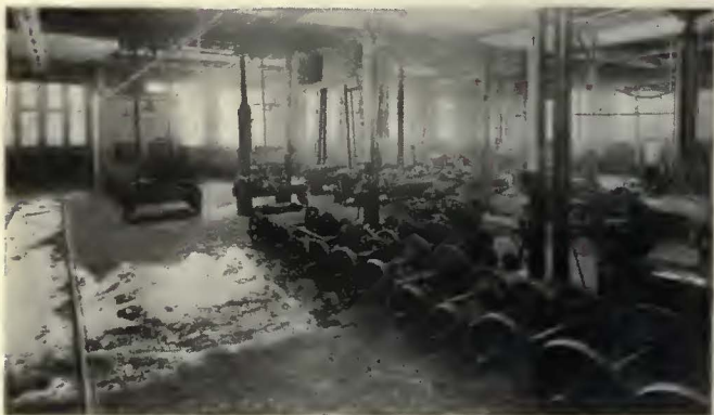
Overhauling and machine shop, looking from the transfer table
