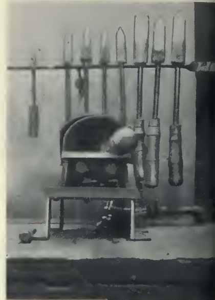
Rack used for soldering irons in the Woodside shops of the New York & Queens County Railway
