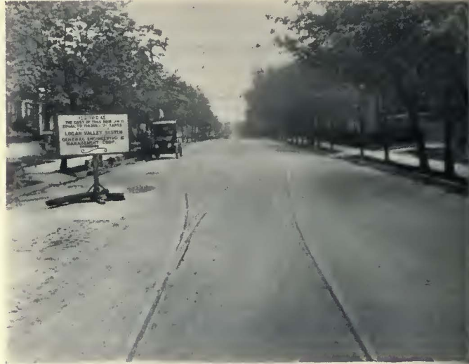
This view was taken 37 days after the previous one, with the new track completed and in service. The sign at the left of the street indicates one of the publicity methods adopted by the company
