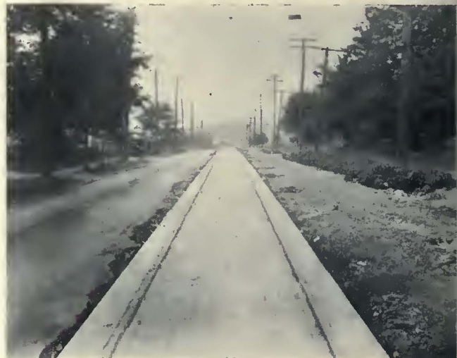
On some of the suburban lines the company has placed the track in paving in preparation for a later paving program of the city which may be carried out this year
