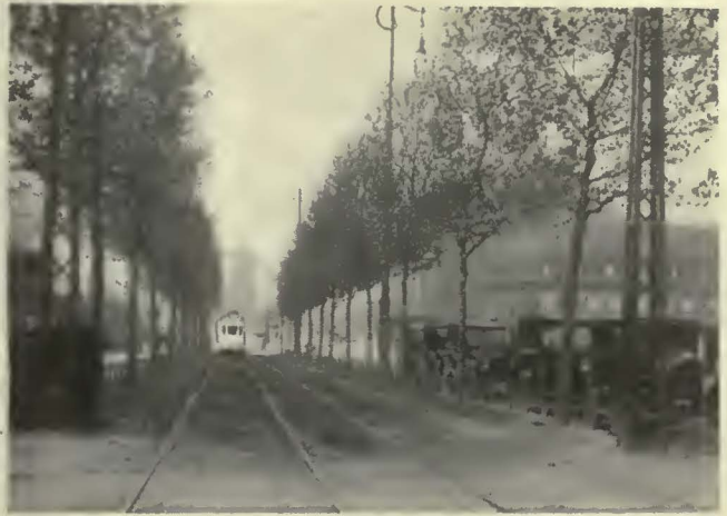
Track is often laid on reservations. The view at the left is from Berlin; that at the right from Dortmund
