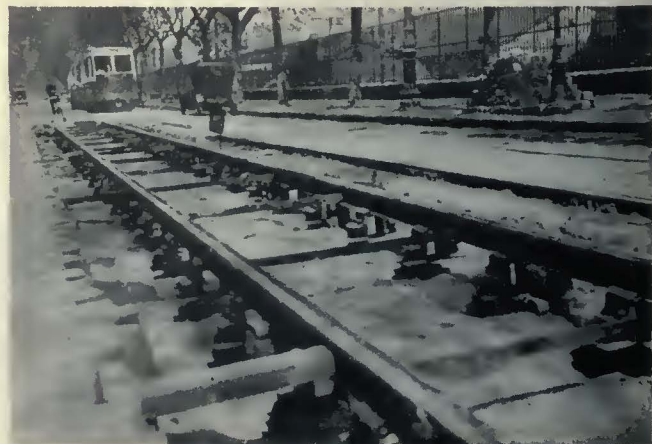
These two views show the method of laying track in Paris. It is first aligned, then mounted on wooden blocks, then the concrete is poured
