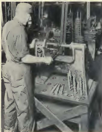
Method of using hydraulic jack as a horizontal press
