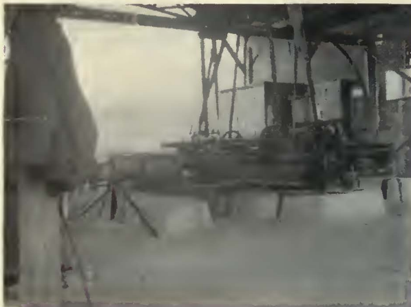
Rail-bending machines form part of the usual equipment of a track yard in Europe. The view at the left shows the rail bender at the Paris yards—The right-hand view shows the shelter housing the rail bender in the track yards of the Hamburg Street Railway. This shelter is directly in front of the company's large track storage house
