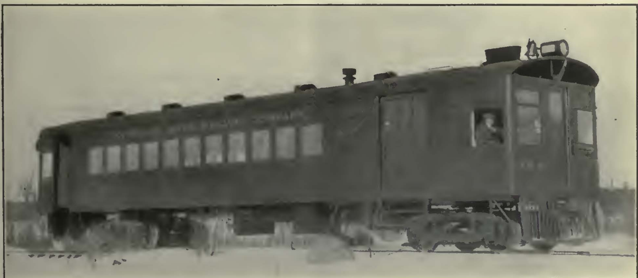
This gas-electric car is handling passenger traffic on an outlying line of the Winnipeg Electric Company's system
