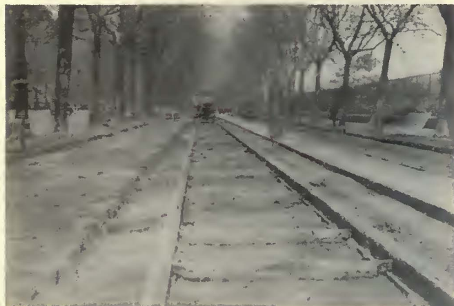
These two views show the method of laying track in Paris. It is first aligned, then mounted on wooden blocks, then the concrete is poured
