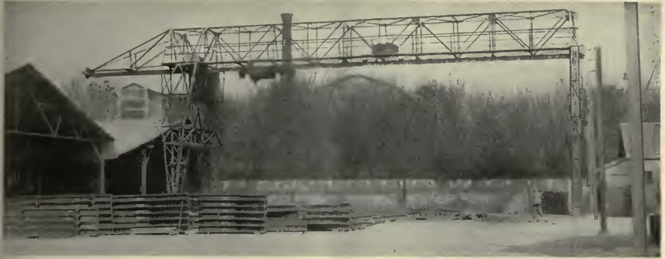
The track yards at Paris are equipped with traveling cranes and other modern machinery
