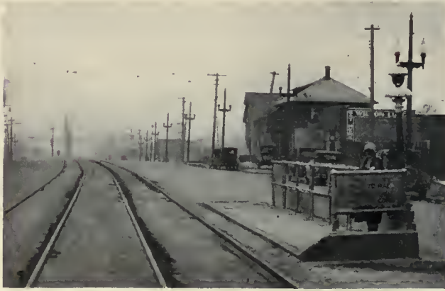
Safety zones and platforms were installed at all important street railway stops in the business district
