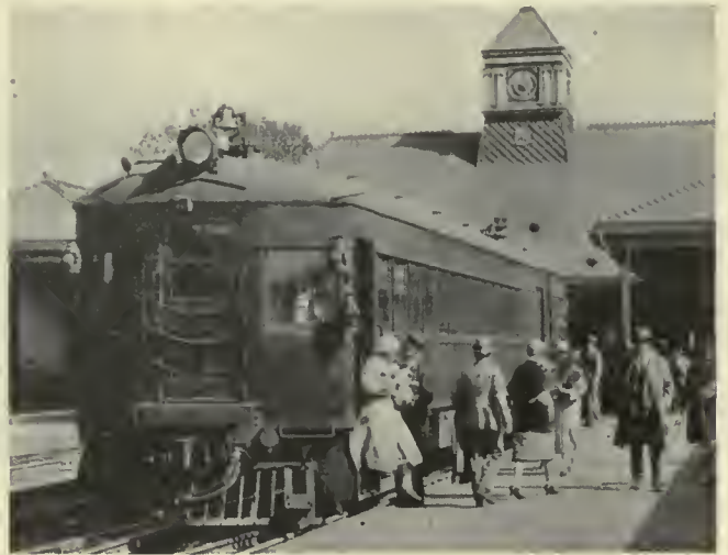
A 60-ft., 250-hp. electric car of the Philadelphia & Reading Railroad at the Trenton, N. J., station
