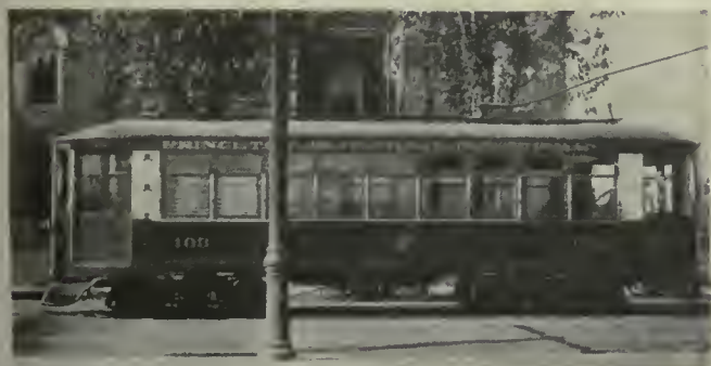
Light-weight interurban car of the Princeton Power Company which has operated continuously since 1917
