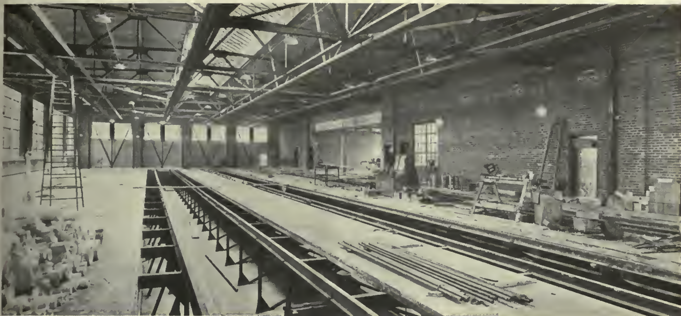
Four tracks extend the entire length of the carhouse, three of which have work pits accommodating a total of twelve cars
