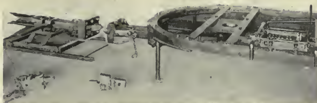
Fig. 3—Demonstration equipment for coupling cars
