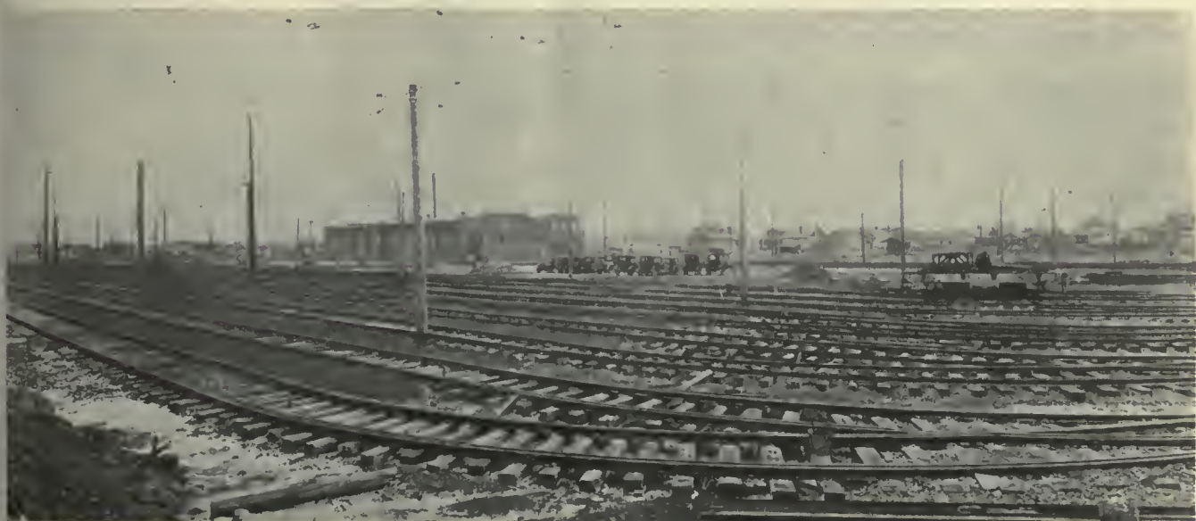
The new terminal for the northwestern section of Detroit has outside storage facilities for 250 cars
