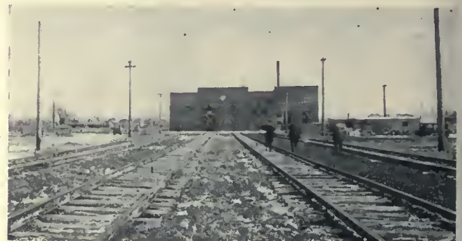
In addition to the repair shop the carhouse has ample office space, sleeping quarters and assembly rooms for the trainmen
