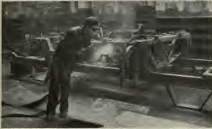
At left—Cutting off heads of rivets to loosen parts that require replacement. At right—Truck frames with parts marked in chalk for replacement and rivet heads cut off so as to loosen parts that are to be removed
