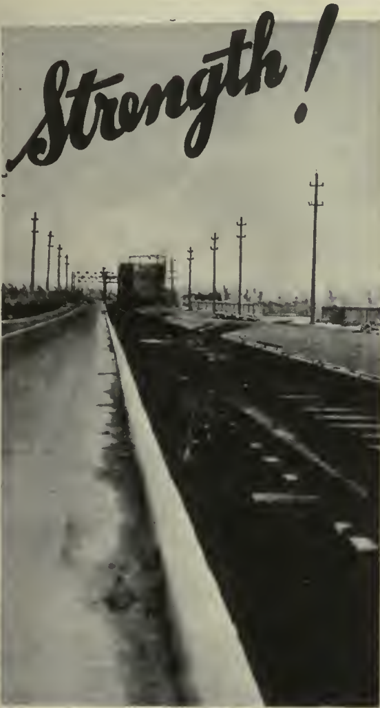
View of the Miami Causeway day following the Florida Hurricane. Observe all Elreco Poles are standing.
