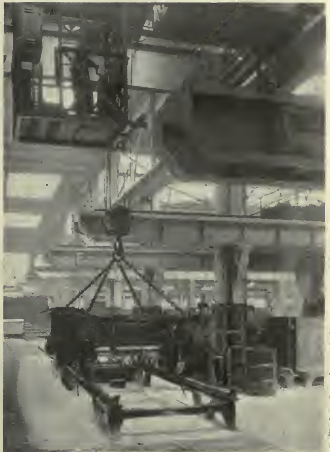
Dropping out wheels and journal boxes while the truck frame is lifted and carried by overhead crane to the cleaning room
