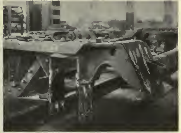
At left—Cutting off heads of rivets to loosen parts that require replacement. At right—Truck frames with parts marked in chalk for replacement and rivet heads cut off so as to loosen parts that are to be removed
