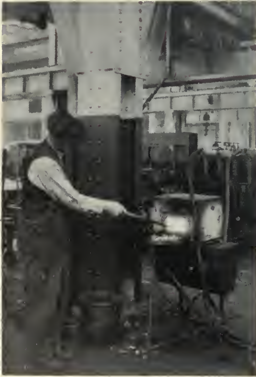
At left—Heating rivets in a portable fuel oil forge alongside the work At right—Riveting new manganese wear plates to truck pedestals
