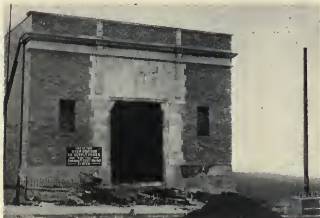
Elmwood substation, which will normally operate as one of three grounded-return stations, but is so located that in an emergency it can feed an ungrounded return or double trolley division
