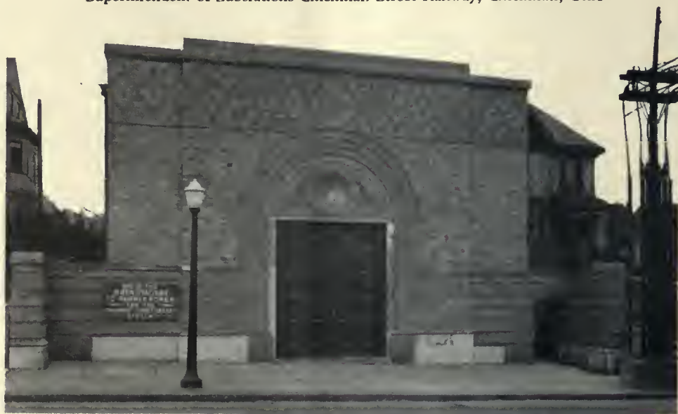
Colerain Avenue substation, one of the nine new 60-cycle stations built in Cincinnati
