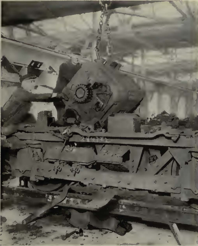
Workmen guide the motor so that the motor axle suspension seats properly as the motor is handled by an overhead crane
