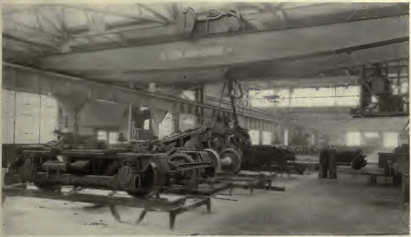
Installing a pair of wheels in a truck in the intermediate repair section of the Coney Island shops. Repair work is done with the trucks on stands, to raise them to a convenient height for the workmen
