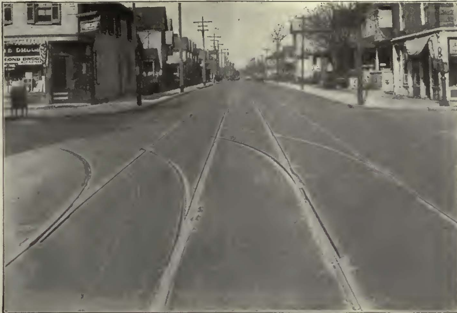
Looking west on Washington Street at the intersection of Cincinnati Street. Note the excellent condition of the tangentials and the smooth surface of the track area. Carey Elastite Track Insulation was used throughout.
