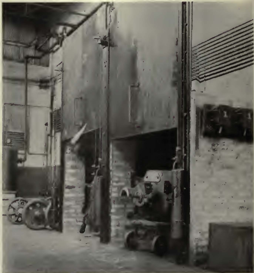
Bake ovens showing sliding doors, counterweights and motors being entered for preheating. The heater control switches can be seen on the brick wall
