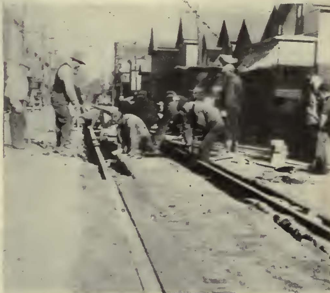
Changing and shimming the rail
