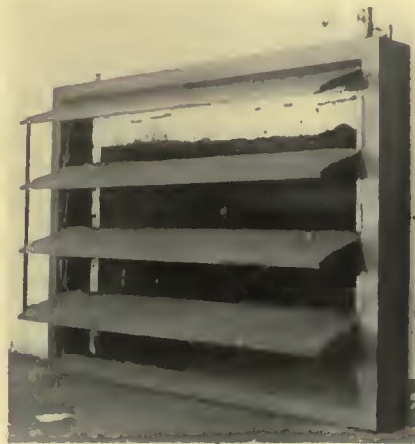
Fan shutter open in air chamber at Front Street substation of Toronto Transportation Commission
