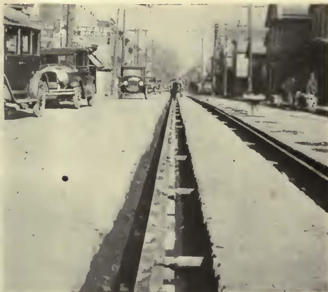
Replaced rail laid and lined
