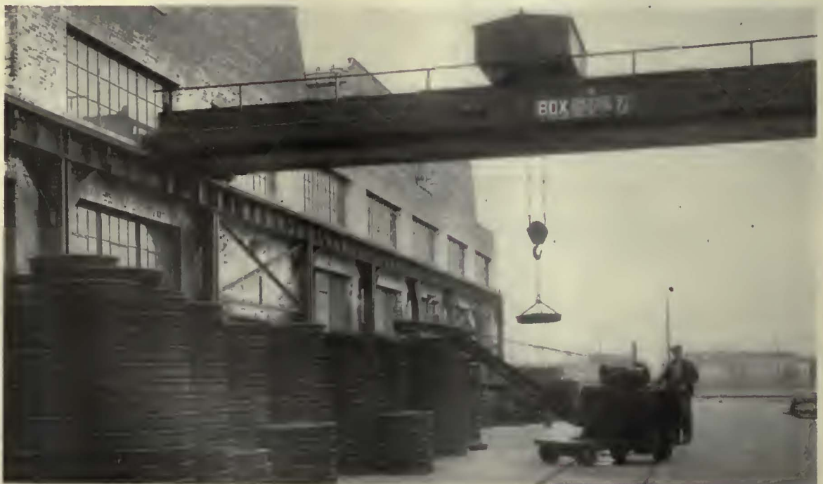
A convenient departmental storage for wheels and axles speeds up production. Material can be brought in on a car and unloaded by the overhead 7\frac{1}{2} -ton traveling crane. Wheels are loaded on small trucks and taken to the wheel and axle department by electric crane trucks
