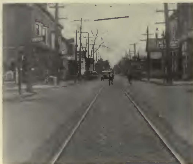
Completed track taken at the same point as the first picture
