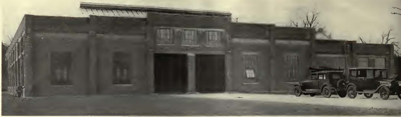
The new Grove Street garage. Space is available to extend the present unit in two directions
