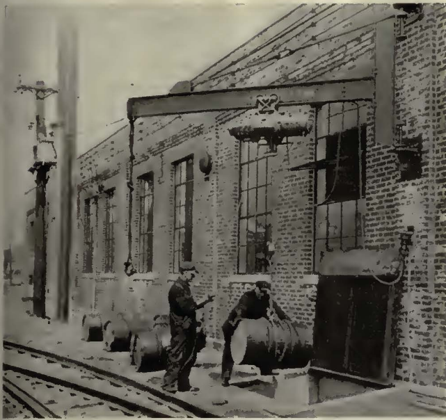
Bracket hoist on carhouse west wall for handling oil and wheels from spur track to pits leading to storage rooms in basement
