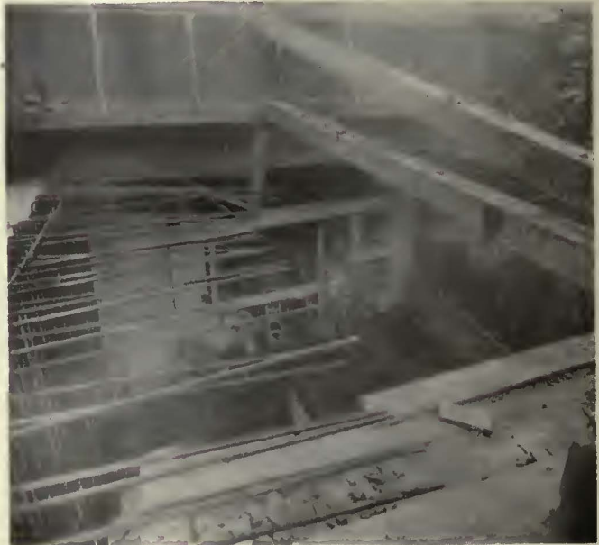
Building a culvert for Pittsburgh railways
