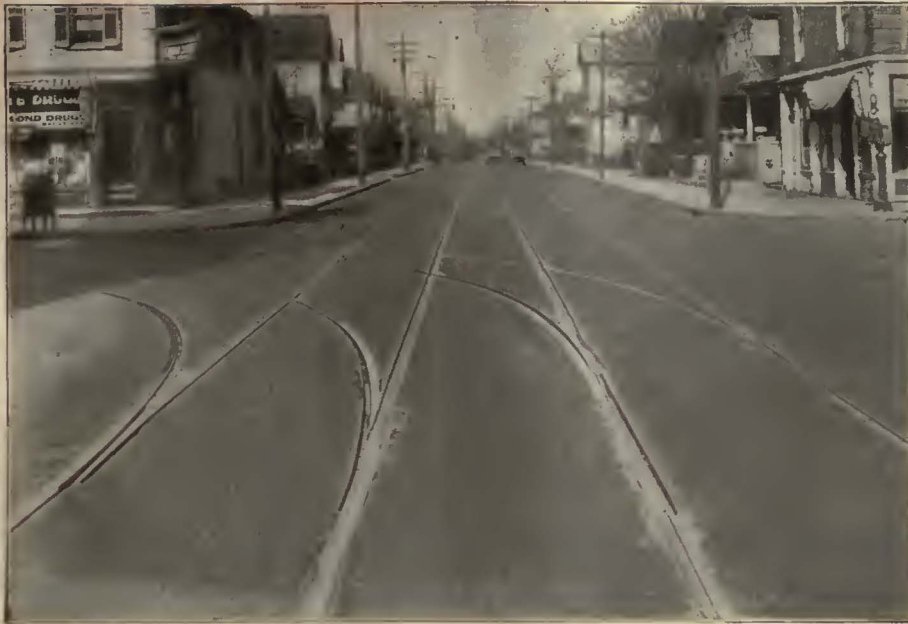
Looking west on Washington Street at the intersection of Cincinnati Street. Note the excellent condition of the tangentials and the smooth surface of the track area. Carey Elastite Track Insulation was used throughout.
