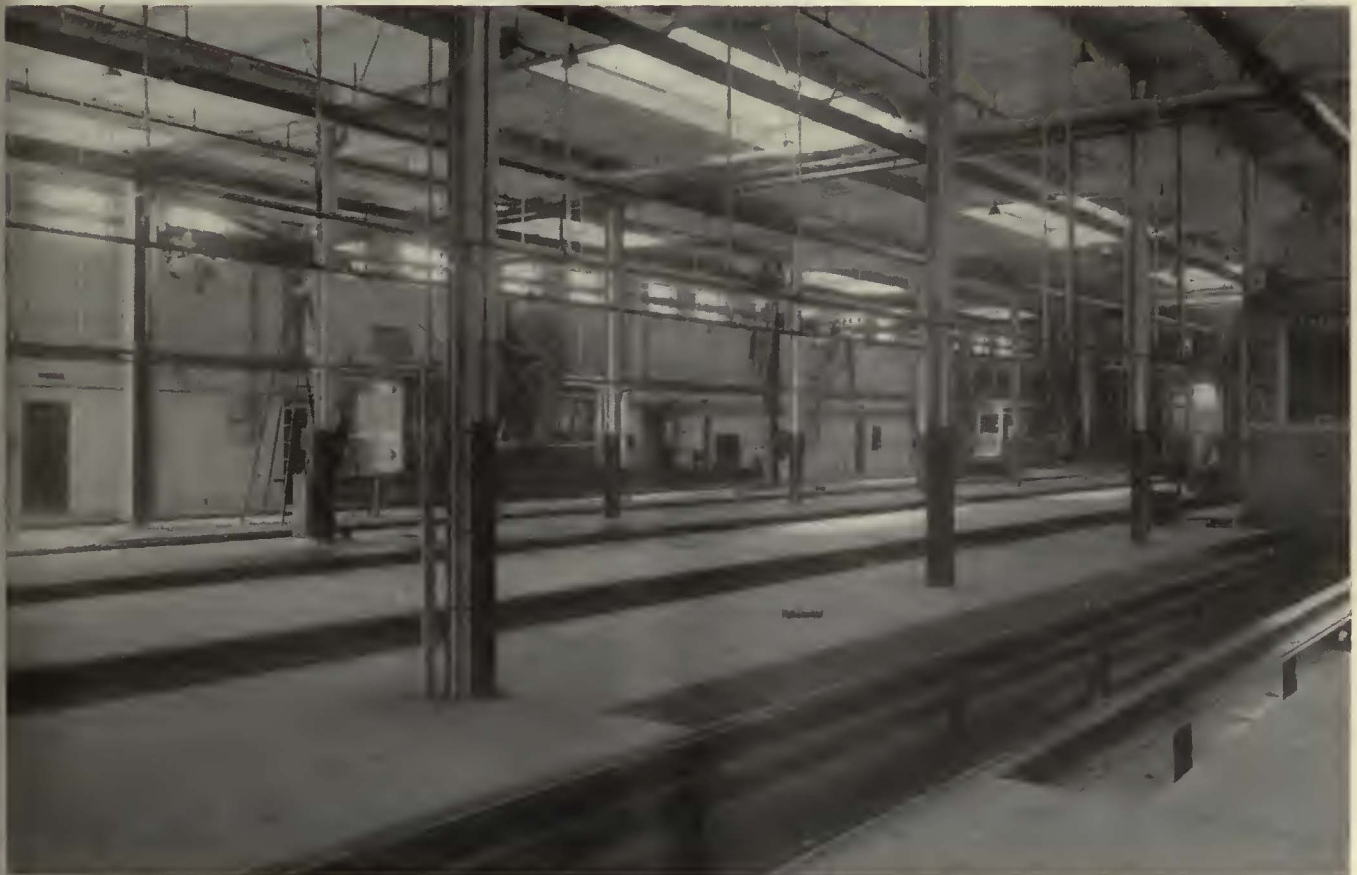
General interior view of Grove Street carhouse inspection bay. Note drop side inspection pit, Columbia car hoist and jib crane
