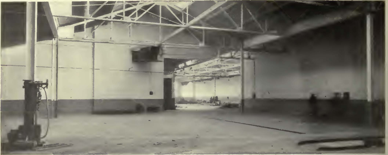
View of the bus garage looking toward the storage end. At the left of the doorway may be seen the ventilation hood and above the hood, the steel roof truss construction. Buses are serviced and repaired in the rear section of the garage
