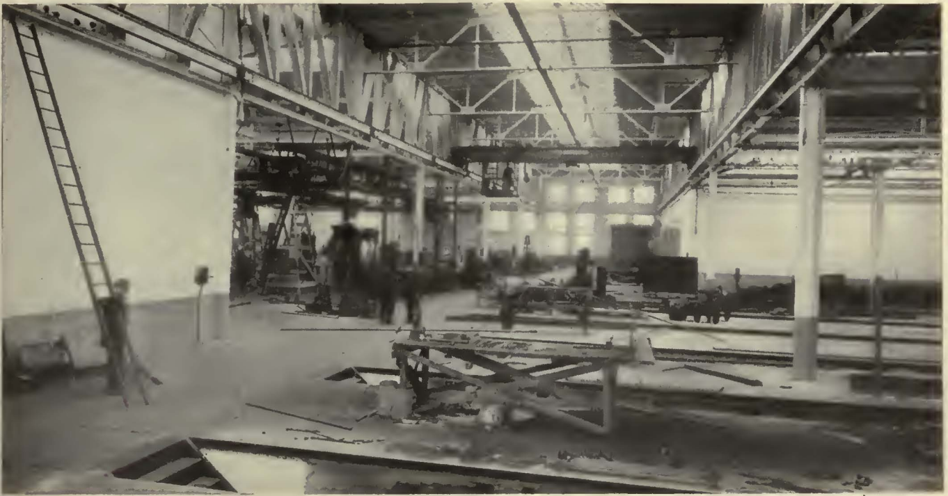
View of the pit room and the craneway. At the left of the crane are the armature repair and machine shops, and to the rear of these shops is the general storeroom
