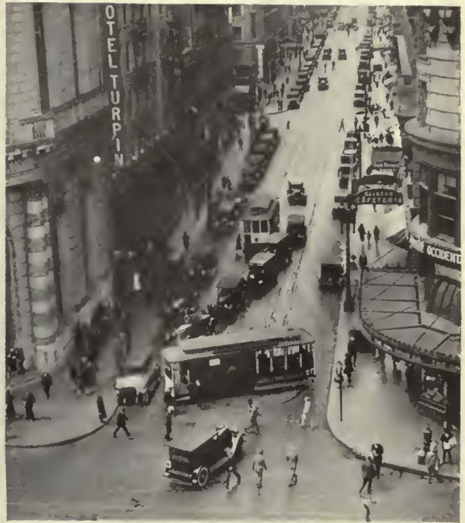
This practice of reversing cars on a turntable on one of the side streets debouching into Market Street blocks traffic
