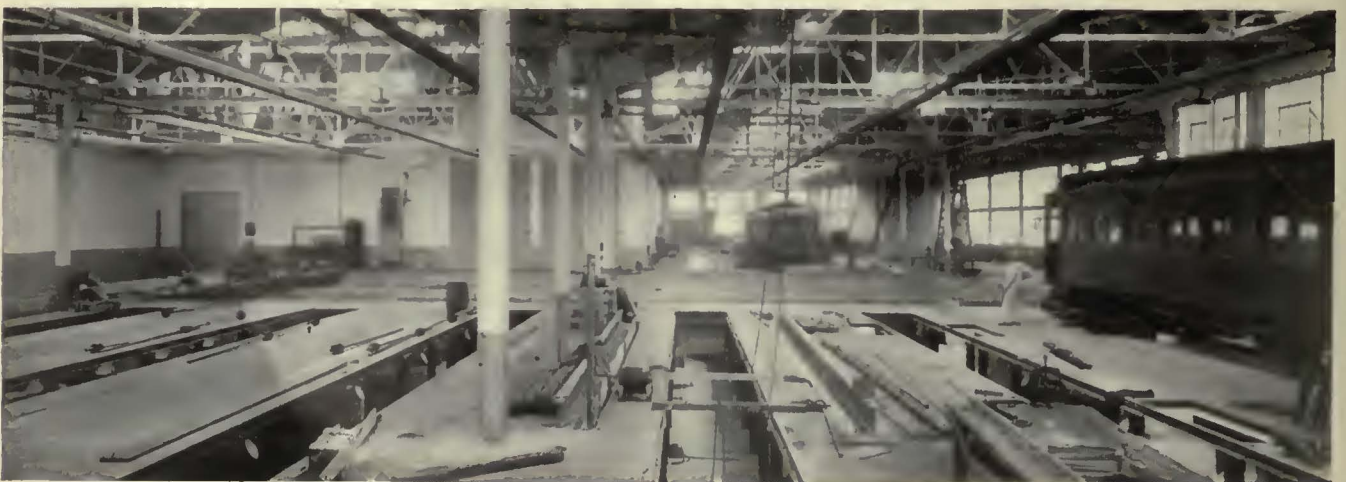
Another view of the pit room, looking toward the carpenter shop and the two closed doors of the paint shop. The transfer table can be seen at the left of its runway
