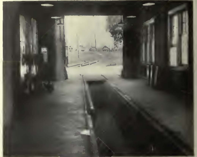
This 60-ft. track pit is so constructed that either a street car or a bus can be run over it
