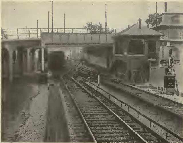
The interlocking tower of the complete yard signal system installed is shown at the right of this view
