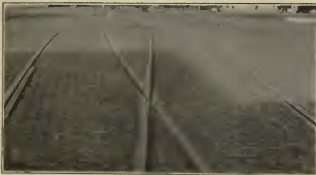
Showing frog installation, at Terre Haute, Ind.
