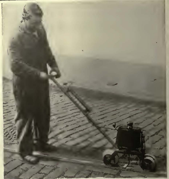
R. T. W. Track Oiler
