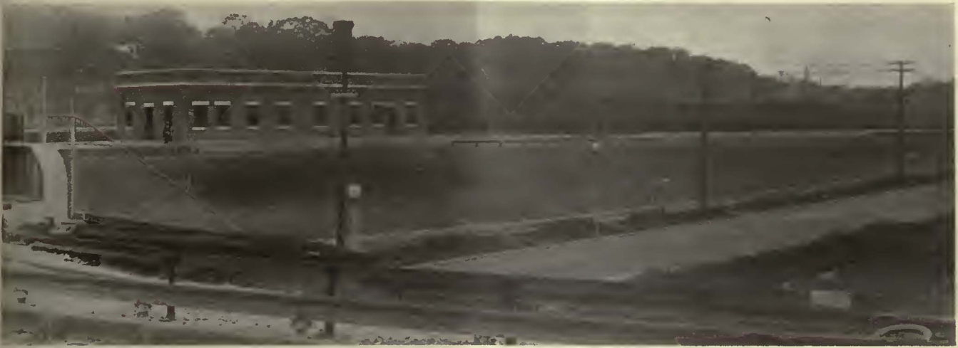
The yardmen's building, at the entrance to the yard, is used by the yardmen of the transportation department, the department of rolling stock and shops, and the trackwalkers, signal men and others of the maintenance department
