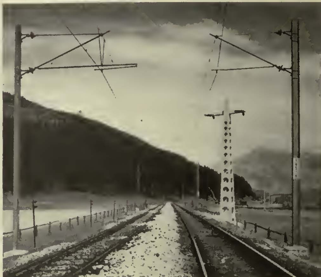
Note type of concrete tower used to carry high-tension transmission line over contact line at Kitzbühel between Wörgl and Saalfelden, Austrian State Railways
