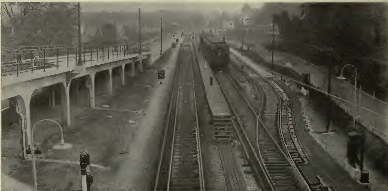
Looking south from Ashmont Station, showing the Codman Street yard in the background. The platform, shown in the center of this view, allows the trainmen to change ends quickly and facilitates the cleaning of cars
