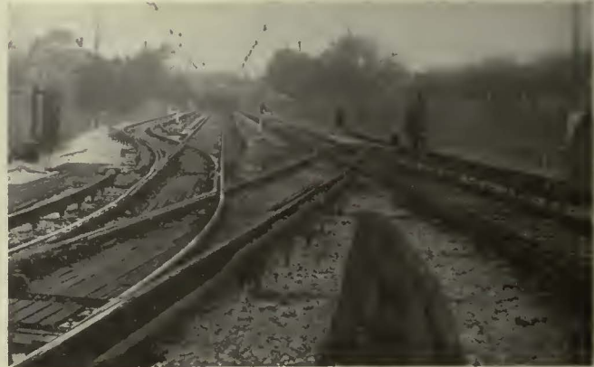
Looking north from the yard. The track at the extreme left is the relay track, used for trains which are to go back into service immediately. Note the wooden platforms for the trainmen and trackwalkers
