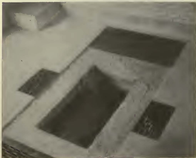
Converter pit and air inlet construction
