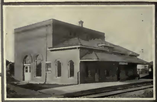
Columbus Grove Substation on the Lima-Toledo Railway
