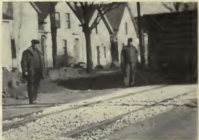
Stone for paving was unloaded from drop-bottom cars
