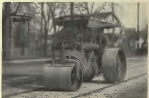
Each layer of Tarmac which was spread under pressure was rolled to within 4 in. of the inside of each rail
