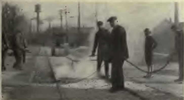
Each layer of Tarmac which was spread under pressure was rolled to within 4 in. of the inside of each rail
