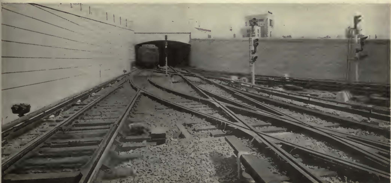
South portal at the terminal yard, showing the types of signals governing movements into the subway proper
