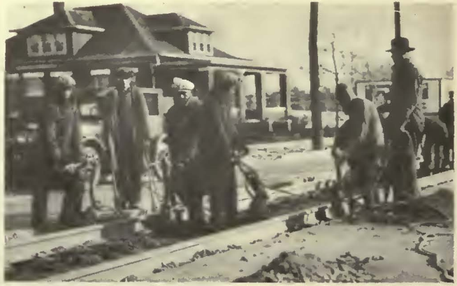
The ties were tamped by the use of electric tamping machines
