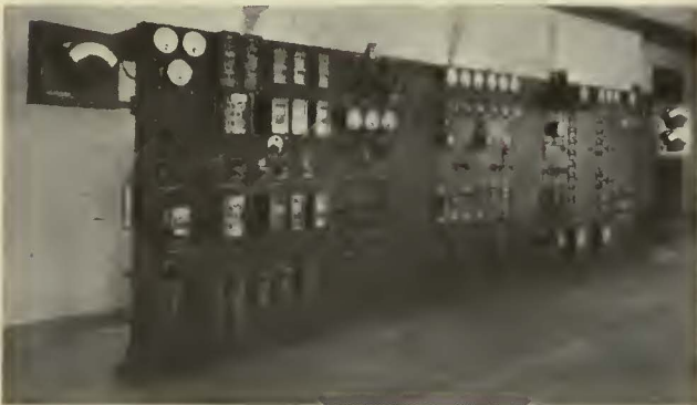
Basement of the Cumberland substation. An individual converter switchboard may be seen at the left and a battery of high-speed circuit breakers at the right
