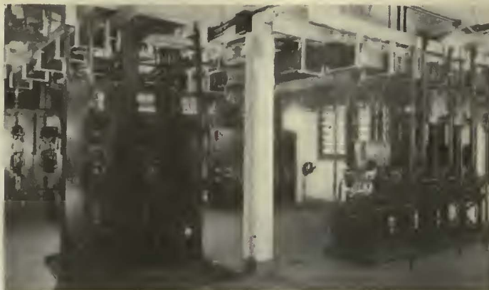
Basement of the Cumberland substation. An individual converter switchboard may be seen at the left and a battery of high-speed circuit breakers at the right
