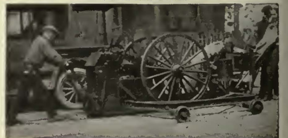
Reciprocating Track Grinder
