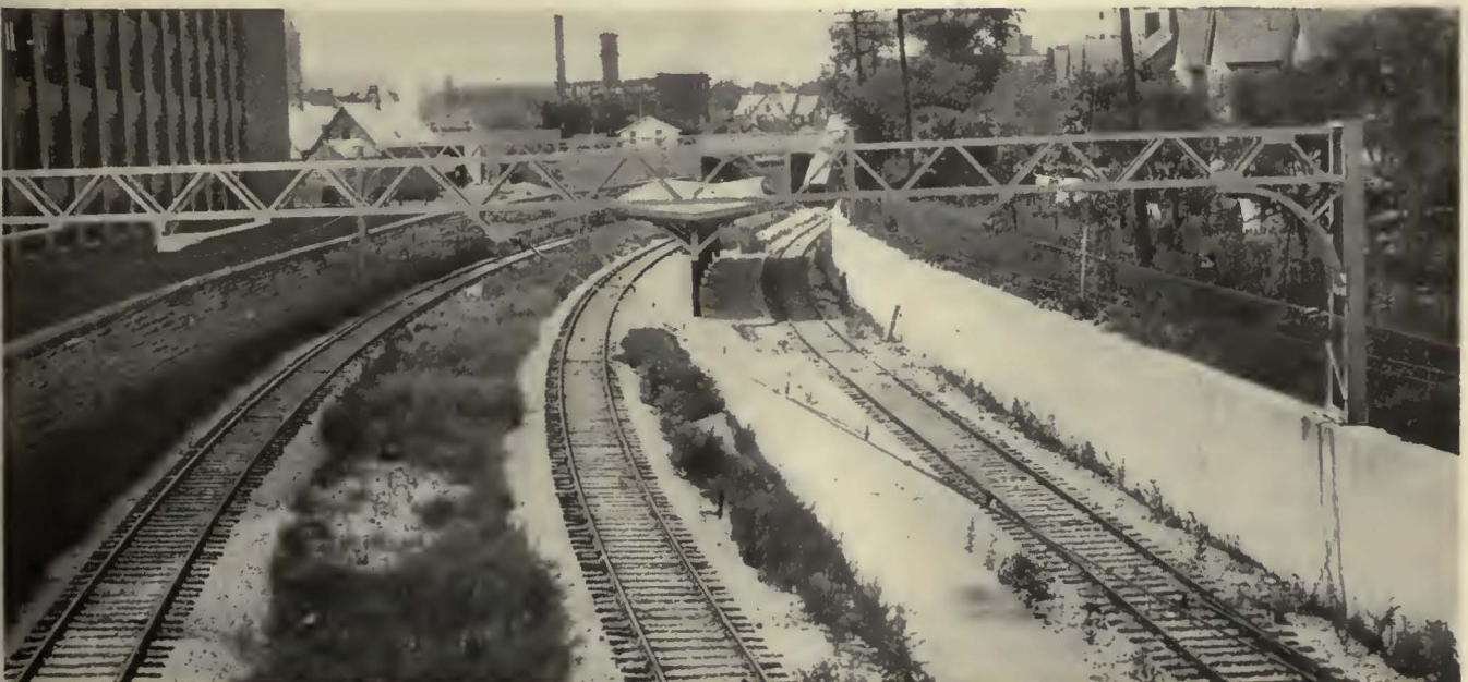
The presence of retaining walls materially decreased the cost of steel for supporting the spans
