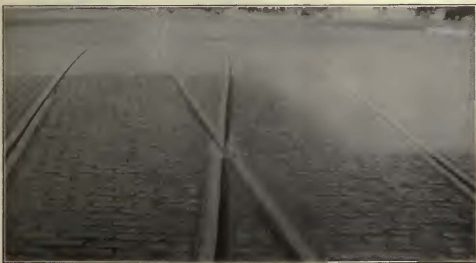
Showing frog installation, at Terre Haute, Ind.
