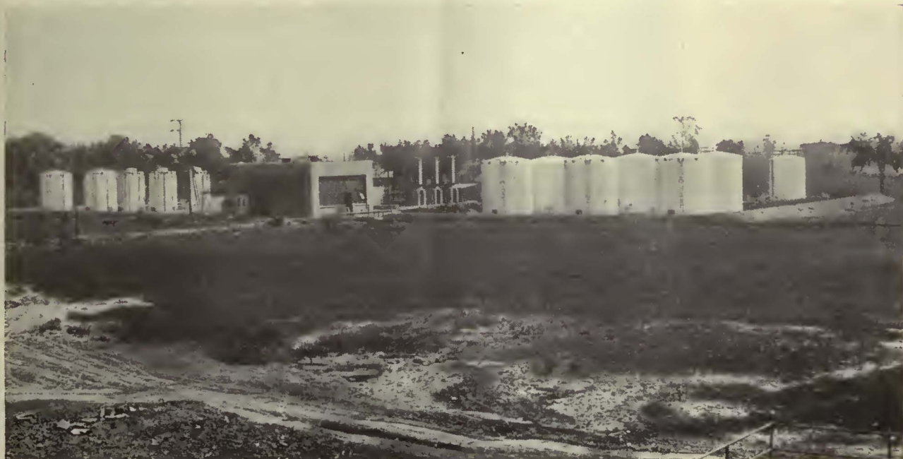
General view of pitch plant
