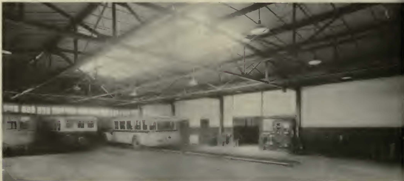
Main part of the garage where the buses are stored and serviced
