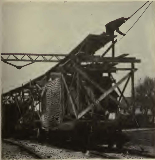
Staging on box and flat cars aided the linemen in connecting catenary hangers
