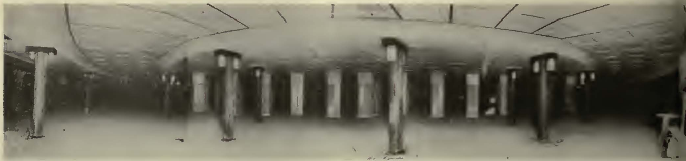
This large circulating area is only 2 ft. underneath one of the busiest traffic centers in London
