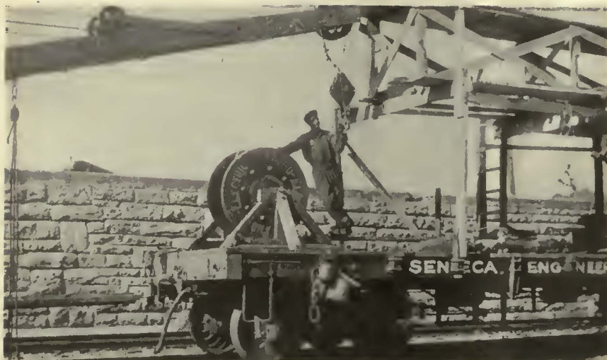
A locomotive crane made cable stringing comparatively easy
