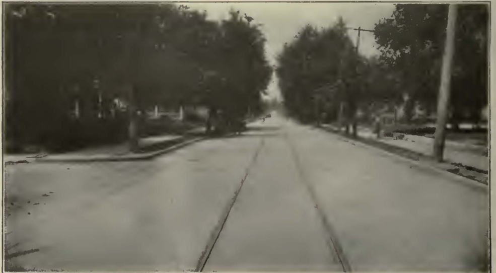
Used with concrete paving, at Richmond, Ind.
