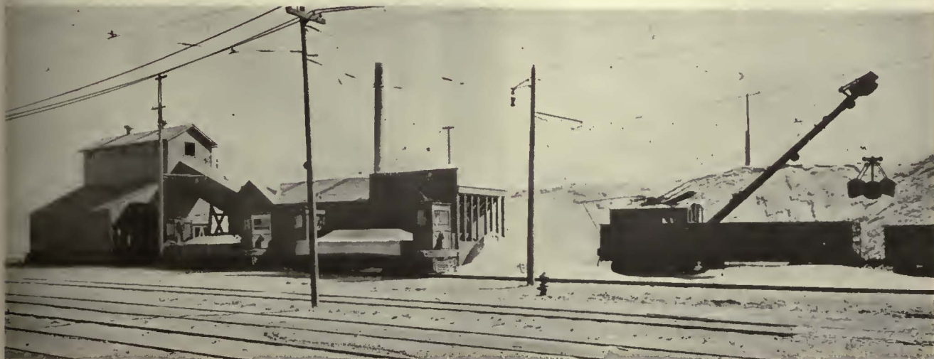
Sand-drying plant of the Chicago Surface lines. The wet sand storage is also shown in the background
