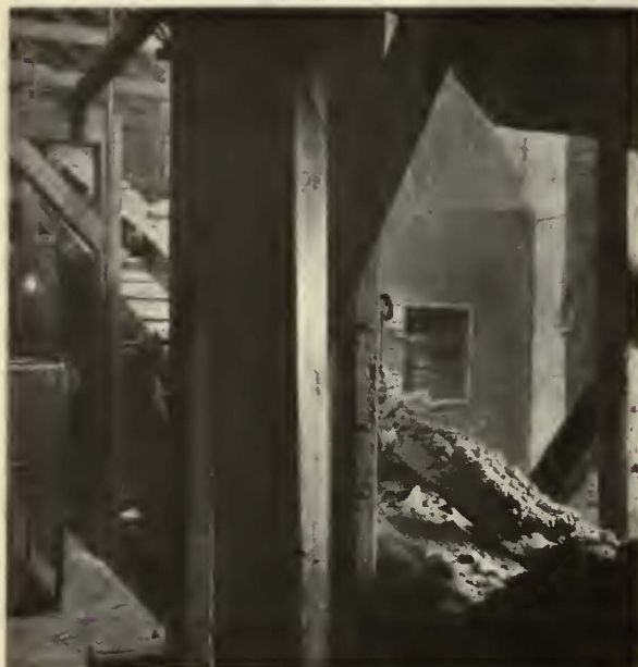
The wet sand is conveyed to the rotating drum, the stack end of which is equipped with a window giving the operator a clear vision of its interior
