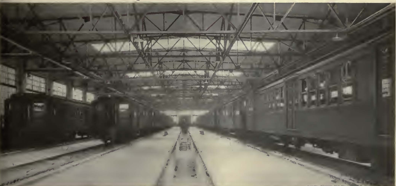
Five tracks extend the full length of the inspection shop, which is long enough to accommodate six-car trains. The tracks are spaced on 18-ft. centers, giving adequate room for the workmen
