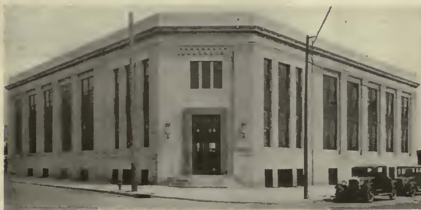
The administration building has quarters for the trainmen and operating staff of the system
