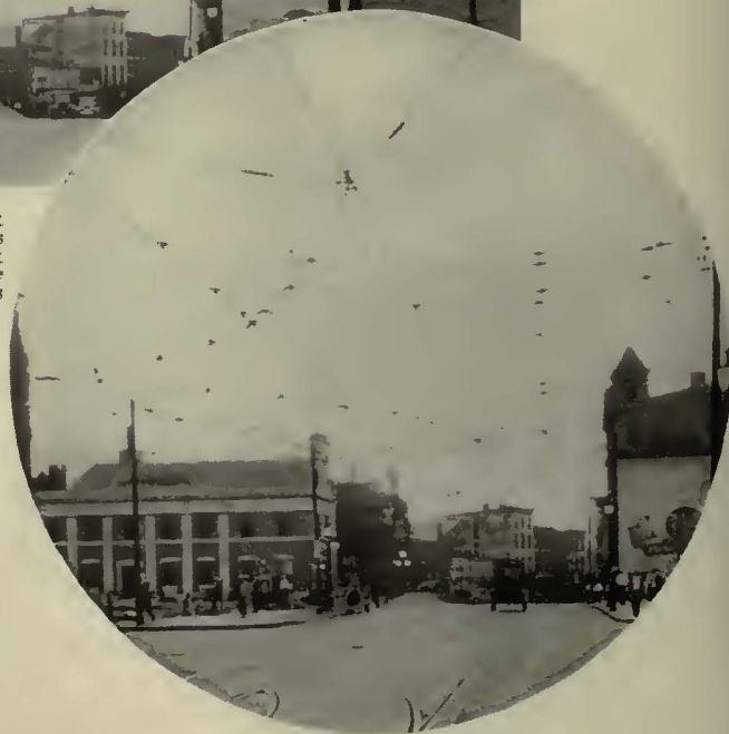
Hangers and ears have been reduced in number at Baltimore by elevating the curve pull-off wires so that they pass over the contact wires without the necessity of being attached thereto. The picture in the circle shows how well this has been done.
