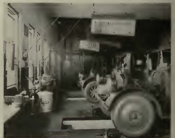
Ingenious method of raising hood for inspection at Milwaukee
