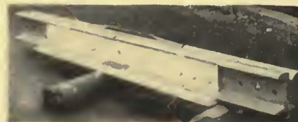
Type of construction used for expansion joint of girder grooved rail
