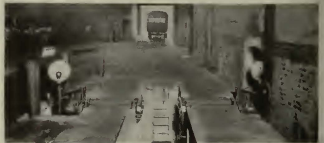
Brake tester and pit in the Charles Street garage of the United Railways & Electric Company of Baltimore
