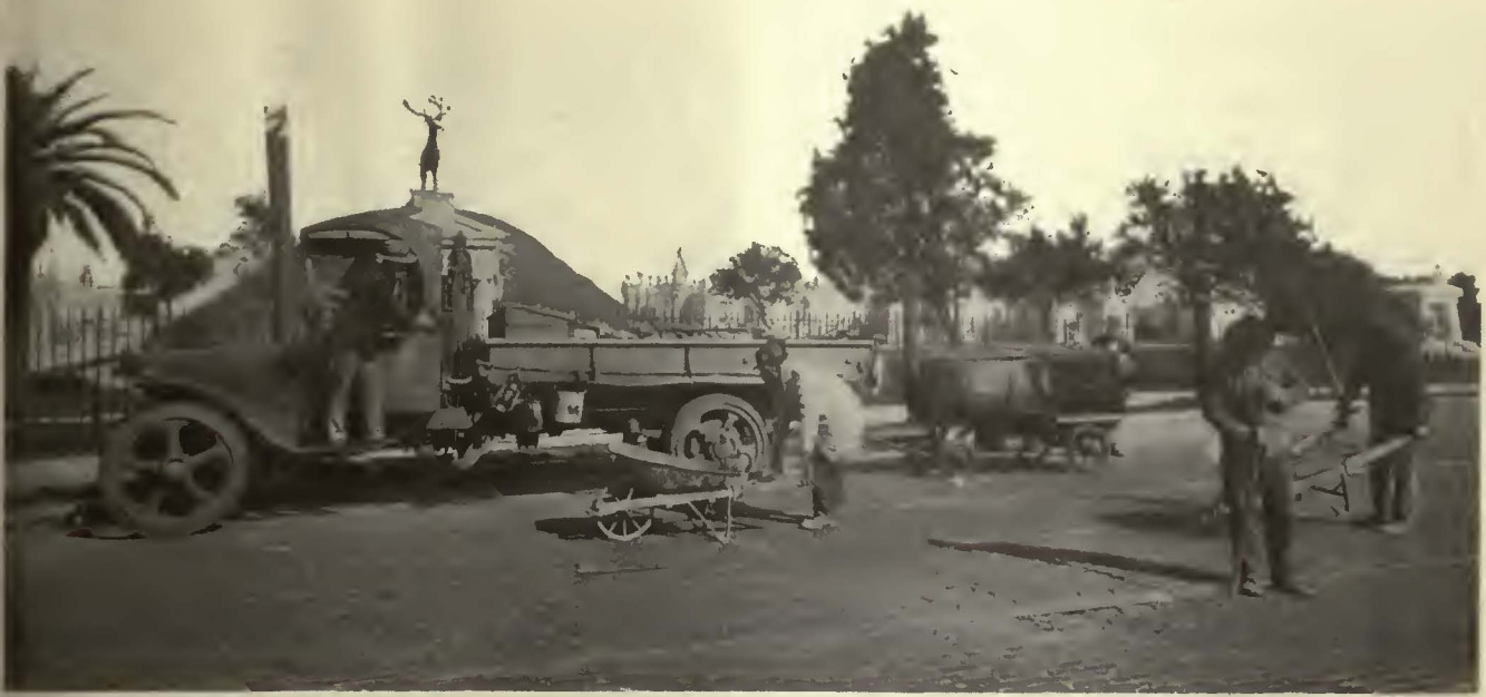
Field paving maintenance unit at work. Truck carries paving materials and hauls oil-burning combined tar kettle and sand drier
