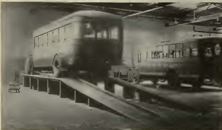
Ramps used instead of pits in one of the Public Service Co-ordinated Transport garages
