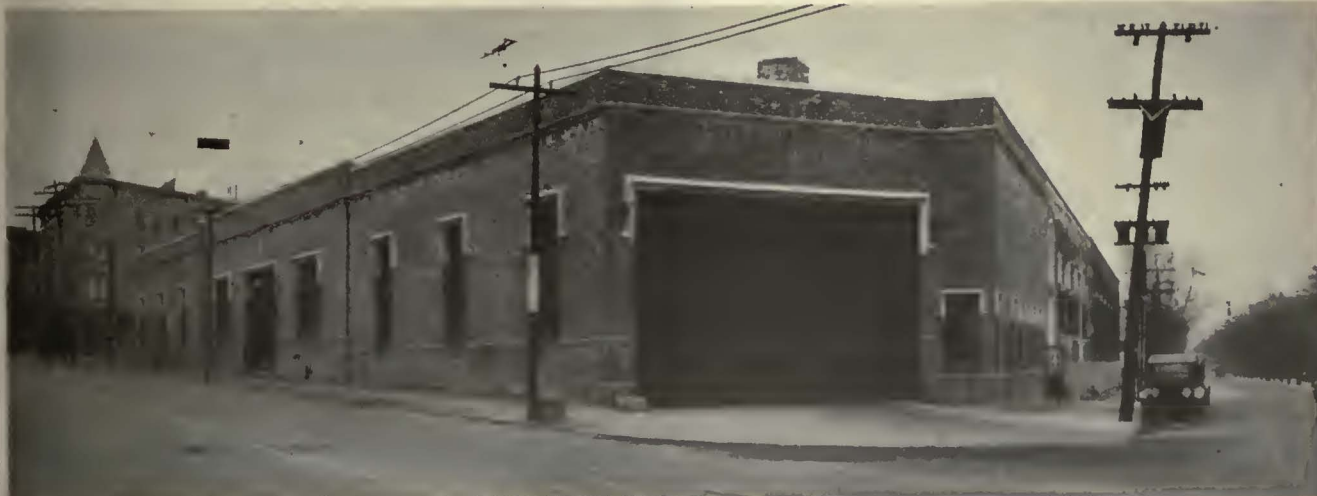
Recently built Lake Street garage of Public Service Co-ordinated Transport
