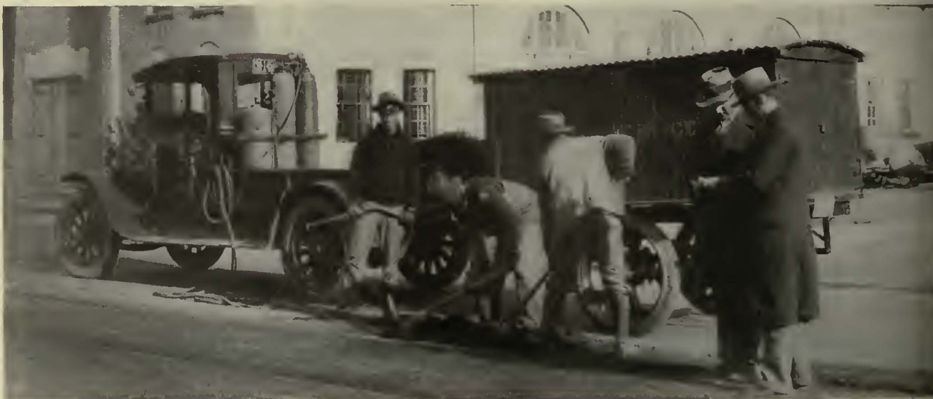
Field track maintenance unit at work. Foreman discussing features of work with supervisor
