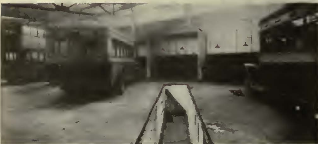
Pits in the new Frankford garage of the Philadelphia Rapid Transit Company are arranged at an angle of 45 deg. with the side walls
