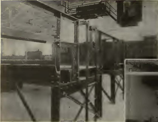
Pit construction in the Dorchester garage of the Boston Elevated Railway is of unusual design with exceptionally good ventilation and light
