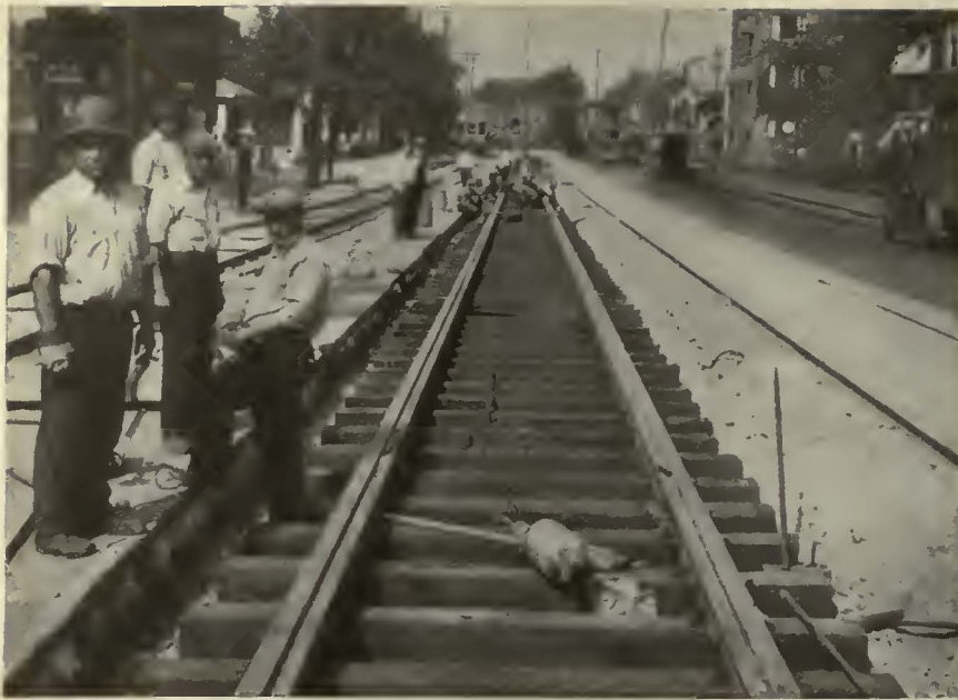
New track ready for surfacing gang
