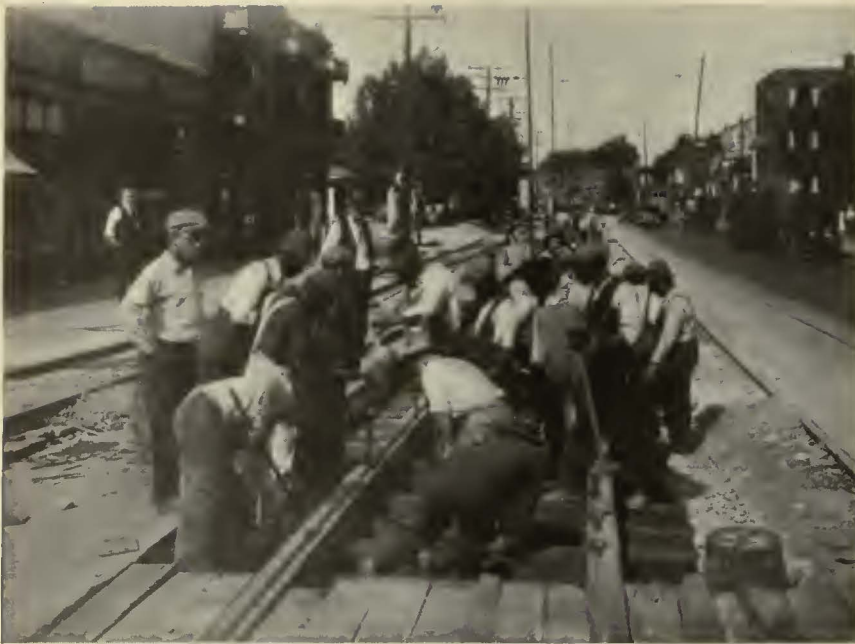
One track was completed and placed in operation, before work was begun on the other track
