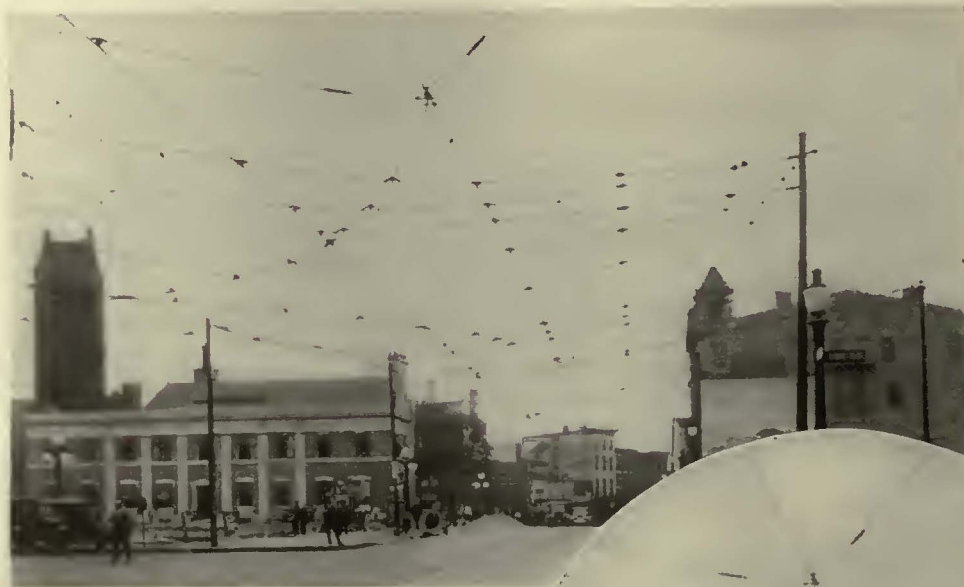
Hangers and ears have been reduced in number at Baltimore by elevating the curve pull-off wires so that they pass over the contact wires without the necessity of being attached thereto. The picture in the circle shows how well this has been done.
