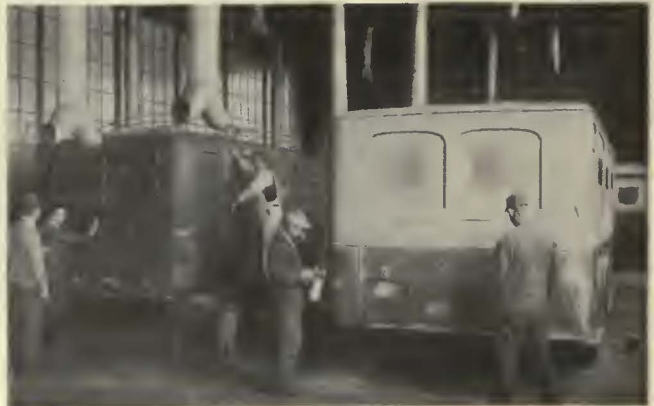
Spray painting at Hillcrest shops. "Bus" bodies are painted red, while "coaches" are painted in two-tone gray
