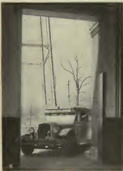
No. 1. Upper floor of Davenport garage, which has a clear space 66 ft. wide.
