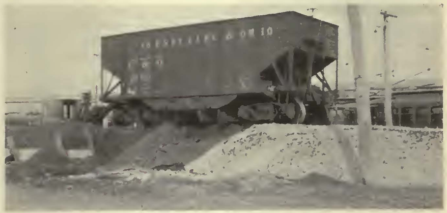
Unloading trestle reduces demurrage charges
