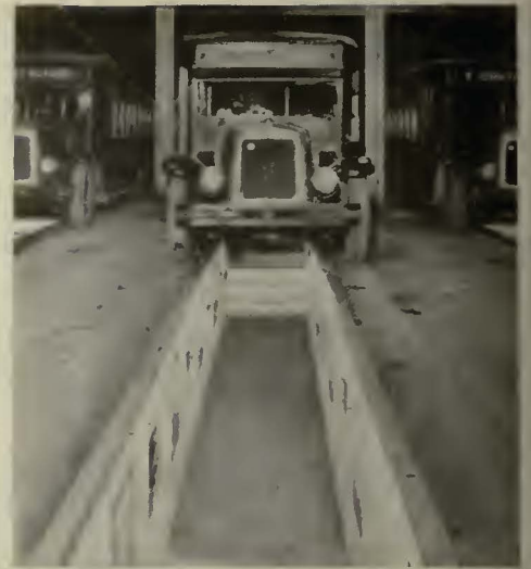
Convenient pit arrangement in bus garage of the New Orleans Public Service, Inc.
