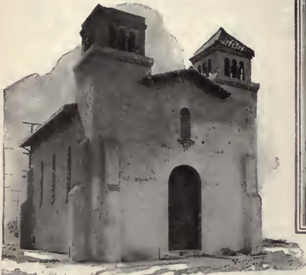
The substation building
