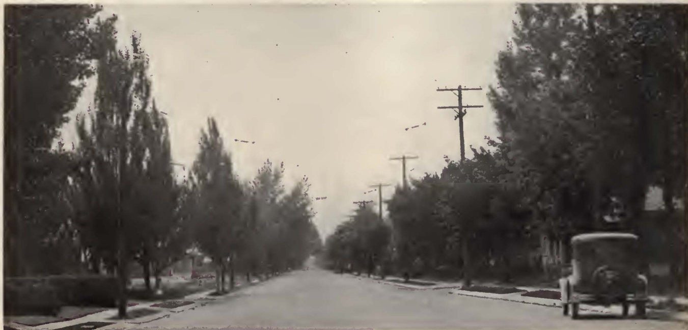
Trolley wires for the electric coaches, installed along the sides, are less conspicuous than wires over the center of the street
