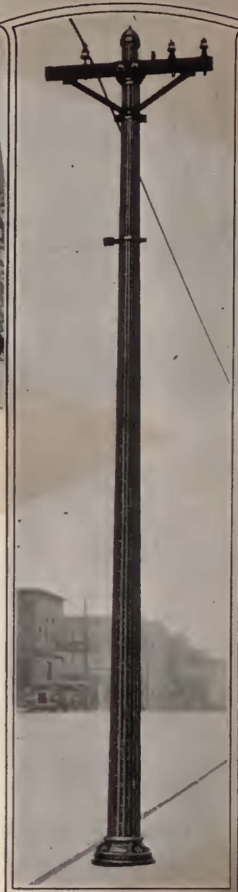
Union Metal Fluted Steel Poles used for trolley span wire support and distribution service, Joseph Campan Street, Detroit.
