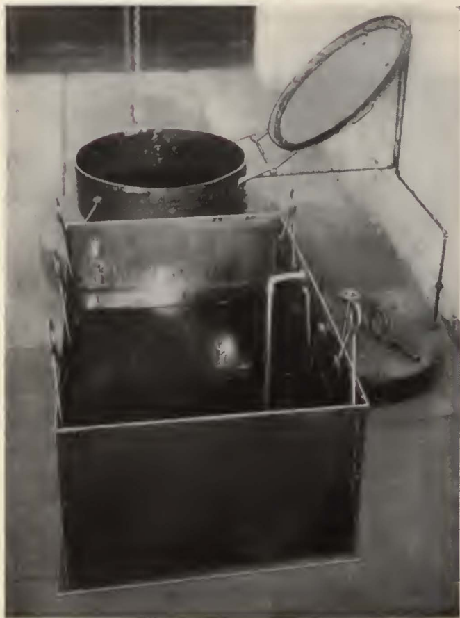
Rectangular varnish vat in shop of Des Moines City Railway will accommodate six G.E.247-I armatures at one time. Circular tank in rear is used for larger armatures. Between rectangular vat and the wall is a 17-in. diameter pressure tank, 45 in. deep, for storage of surplus varnish
