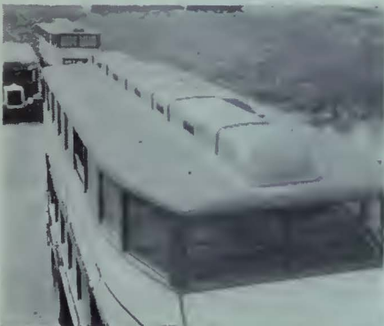
(Left) "Metal to metal contact won't do," said P. R. T. officials. "Top leaks have to be eliminated." And they were with Goodrich Rubber Seam Bands!
