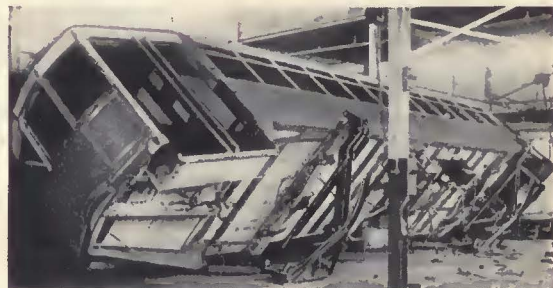
Trucks designed to permit turning over of car bodies in the shops of the Cincinnati Street Railway
