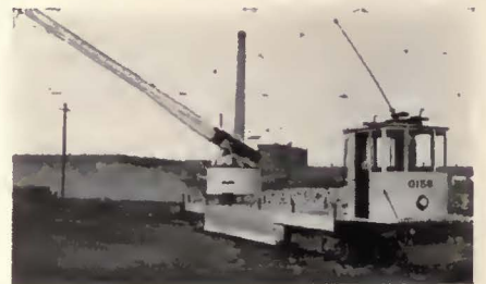
Differential Electric Locomotive Crane Car for Electric Railway Service
