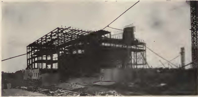
Progress Picture, Power Station
