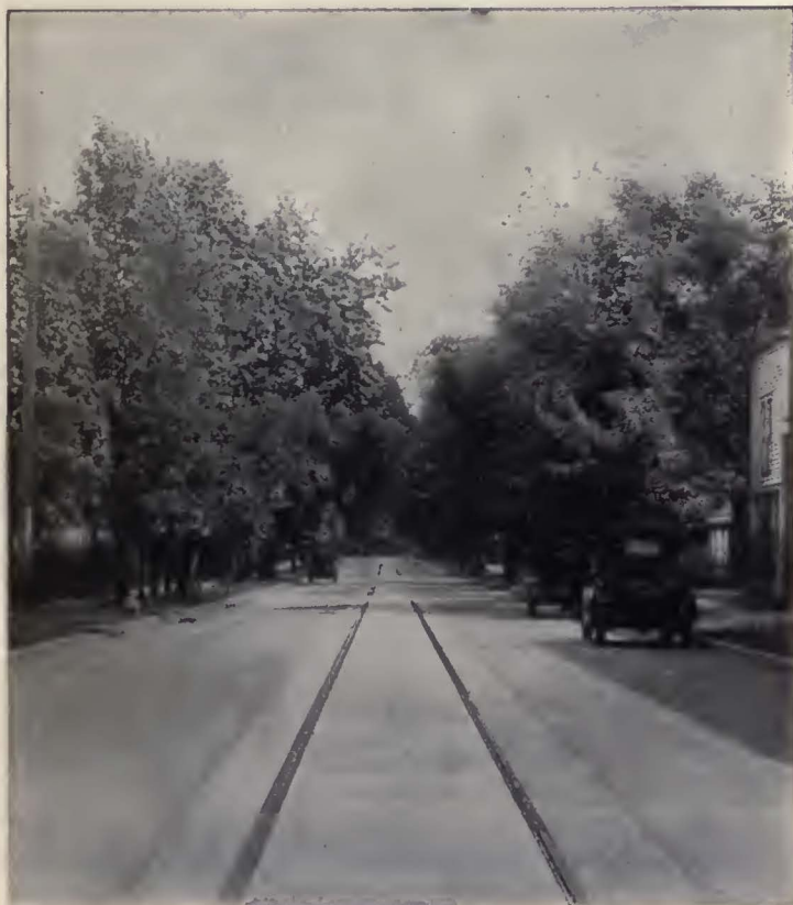
The completed installation—Carey Elastite System of Track Insulation, used in connection with a standard 85-pound A.S.C.E. T-Rail and a roadway of concrete.
