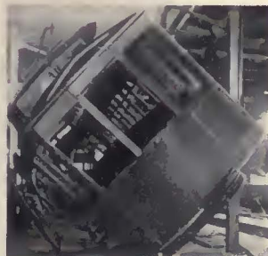
Trucks designed to permit turning over of car bodies in the shops of the Cincinnati Street Railway
