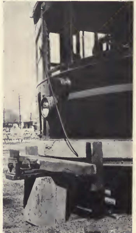
Jack for straightening bent bumpers
