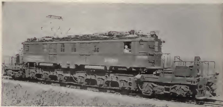
Electric locomotive to be used in the electrified zone of the Cleveland Union Terminal
