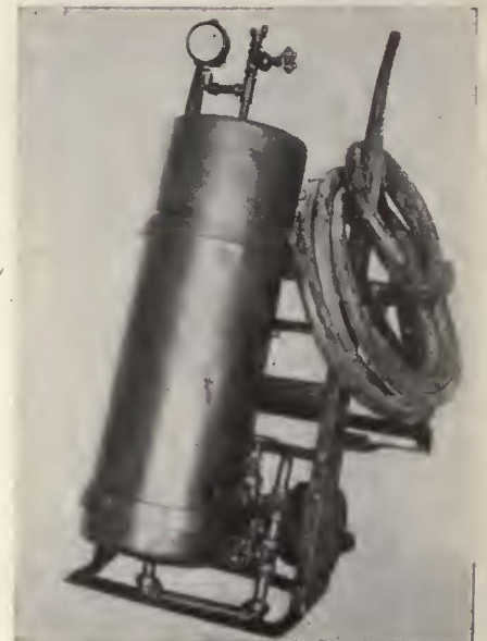
Portable flushing machine for bus engine cooling systems
