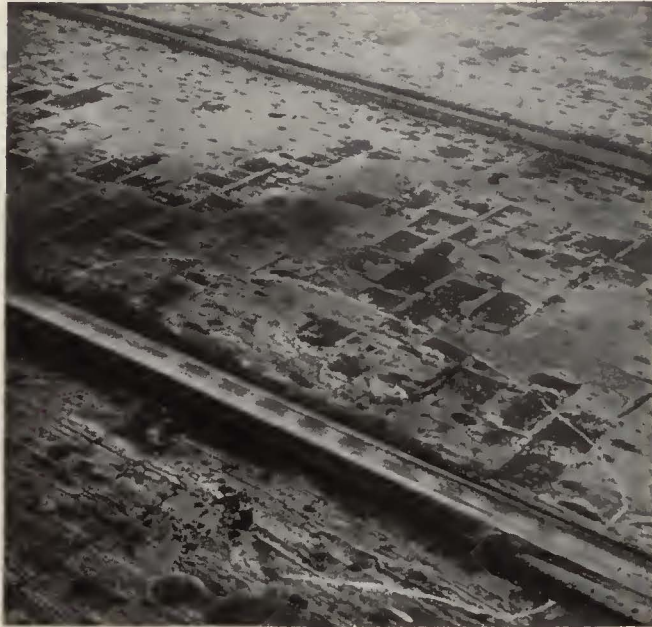
When cupping appears, the rail should be ground immediately; otherwise, the depressions develop into deeper ones and cause much damage
