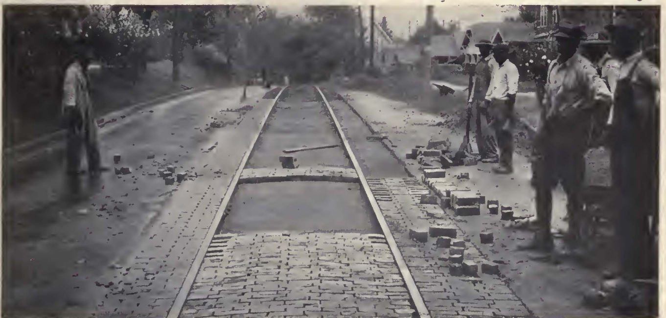
Though a sand cushion is necessary in a block pavement to take up the inequalities in the blocks and to distribute the load uniformly over the base, it need not be very deep
