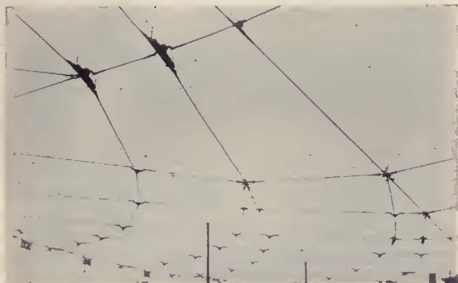
Overhead special work redesigned to permit of bow collection
