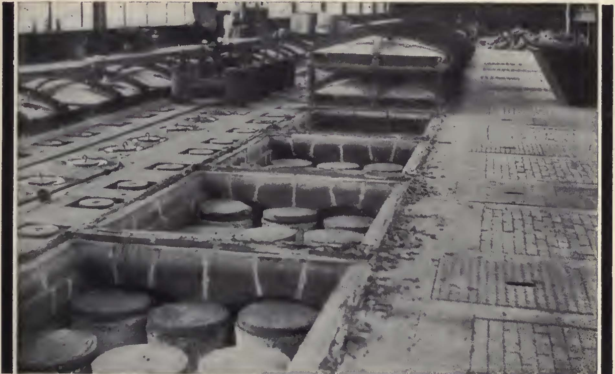
View of part of a ring furnace
