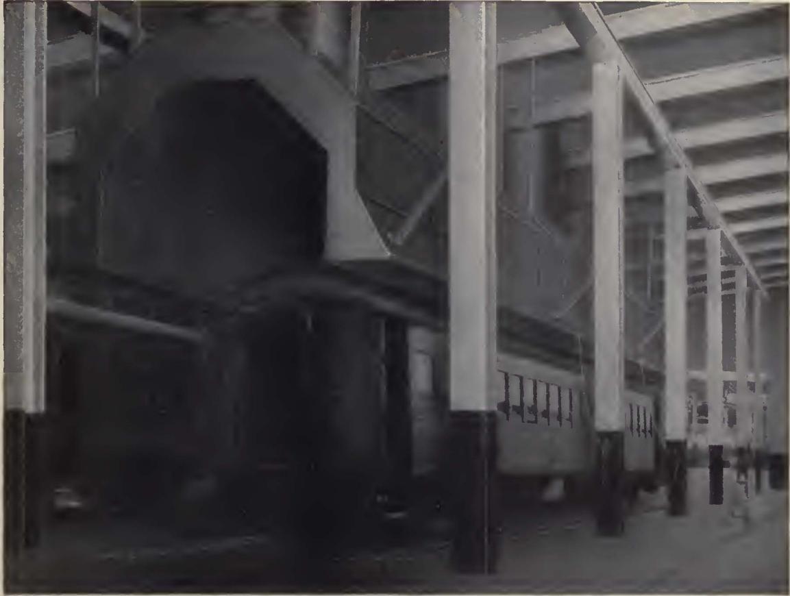
DeVilbiss Stationary Canopy Type Car Exhaust (Patent applied for)
