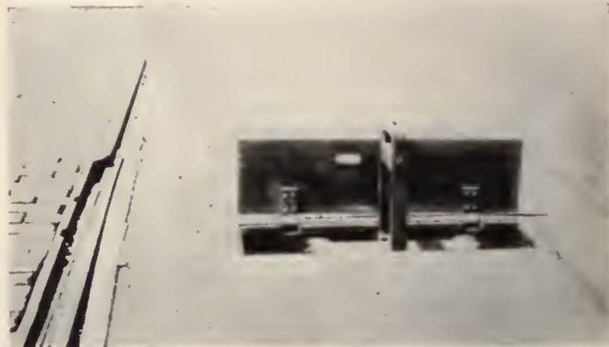
Oil-buffed spring tongue switch of the Chicago, South Shore & South Bend Railroad. Box open with manual control handle in neutral position
