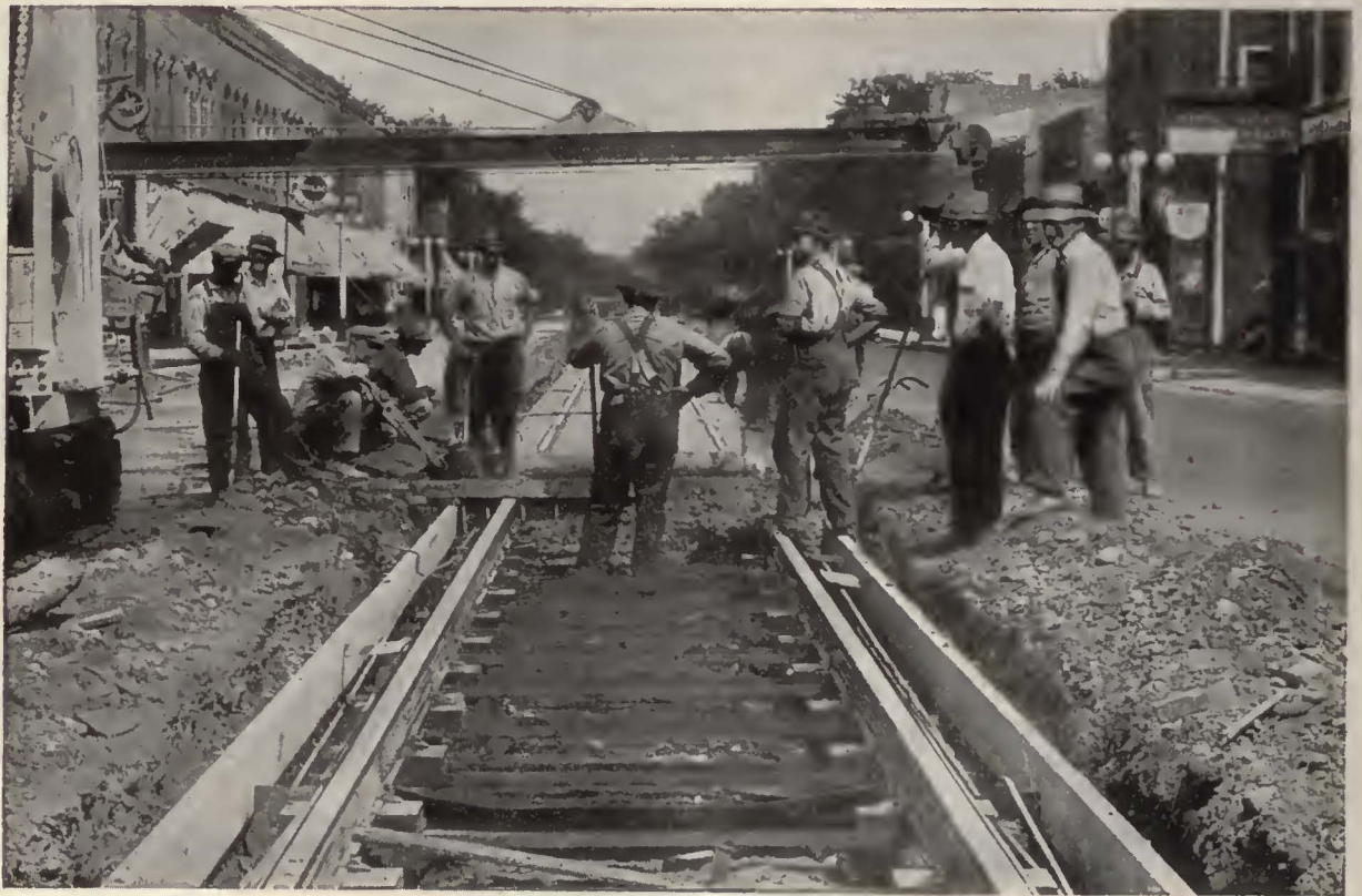
Showing the application of Carey Elastite System of Track Insulation on the Northern States Power Company's lines through Eau Claire, Wisconsin.
