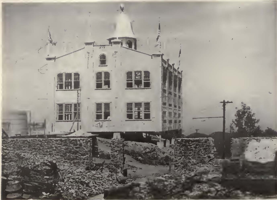
Fast work was done on temporary structure on Mount Tom
