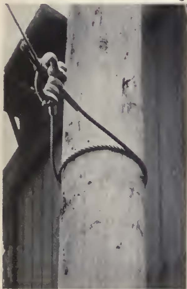
How dead-end sling is attached to post
