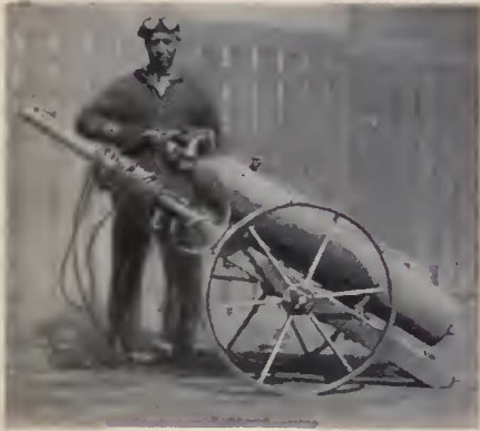
This truck for welding equipment is easy to move about and requires the services of only one man under the most unfavorable conditions
