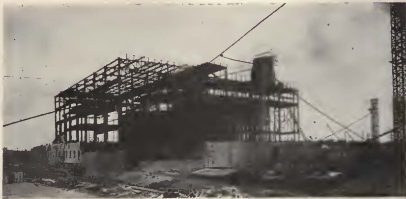
Progress Picture, Power Station
