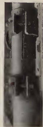
Economical method of reclaiming span-wire poles by reinforcing sleeves
