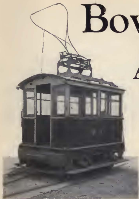
Original type of bow collector used for five years on Toronto shunters
