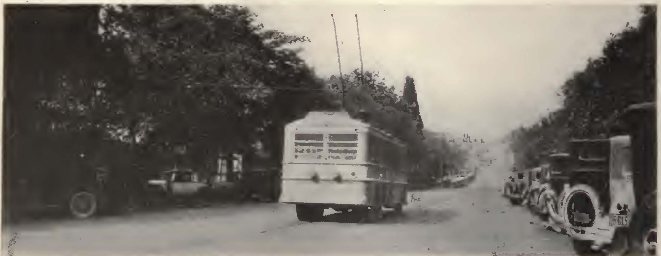
Trackless trolleys involve smaller capital cost than street cars and are cheaper to operate than are motor buses
