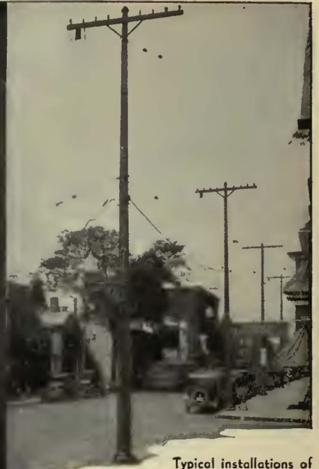
Typical installations of Union Metal Fluted Steel Poles
