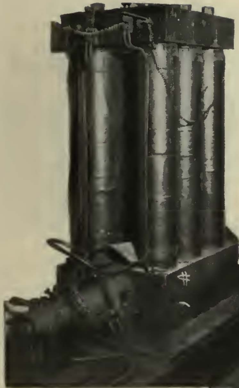
Above. An Edison 250-light type K generator in use from 1883 to 1928. Equipped with copper leaf brushes.
