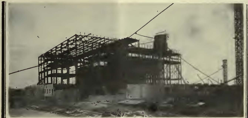
PROGRESS PICTURE, POWER STATION
