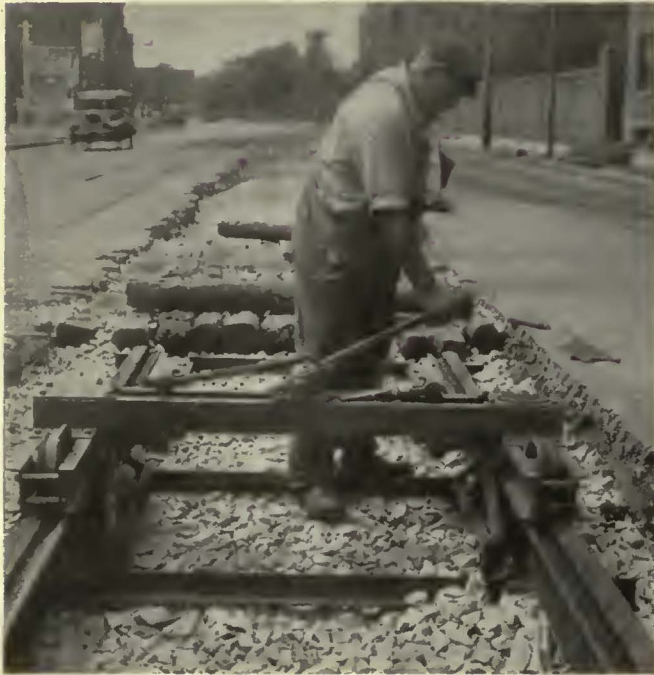
Seven-inch grooved girder rail was used with rolled-steel joint plates seam welded
