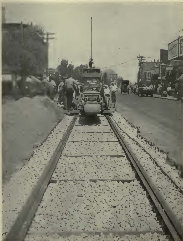
Mixing apparatus mounted on railway trucks was used for grouting
