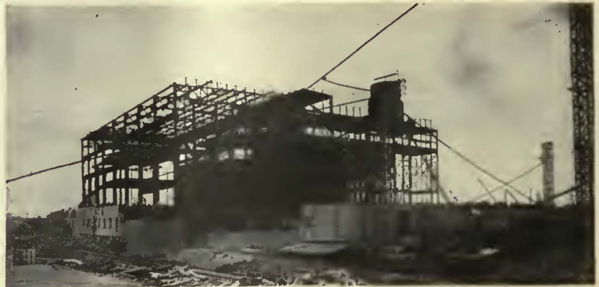
Progress Picture, Power Station
