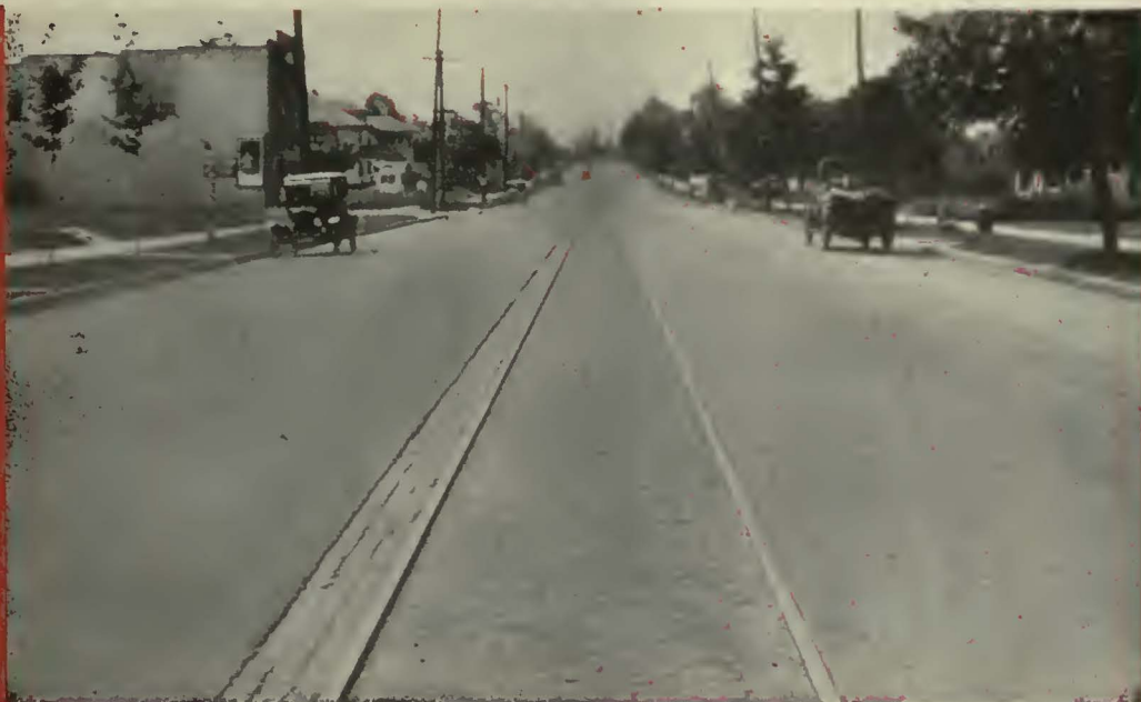
The track shown above is a continuation of the track shown in picture No. 1, opposite page. But in this section Dayton Ties were used. Note the unbroken pavement and absence of any sign of "VIBROLUTION."
