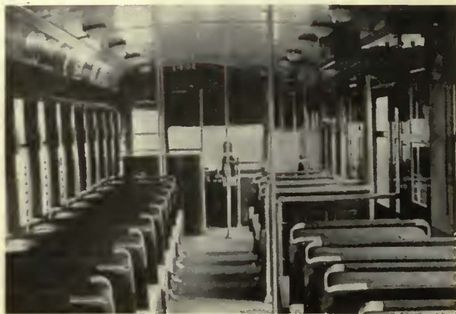
Front half of the car showing the arrangement of stanchions and the type of seats used
