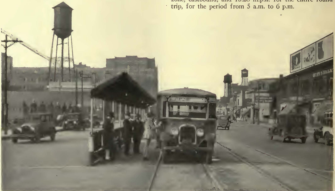
On Jefferson Avenue the local transfer buses run inside the safety zones at express stops. Between these stations they stop at the curb
