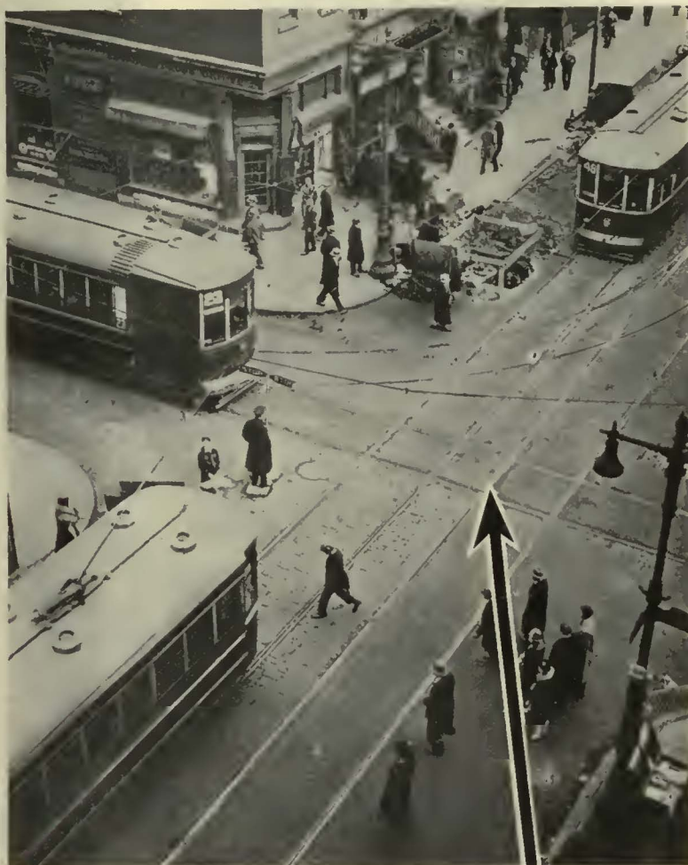
Bethlehem Silico-Manganese Weldable Crossing and turnout at 10th and Arch Sts., Philadelphia, Pa.
