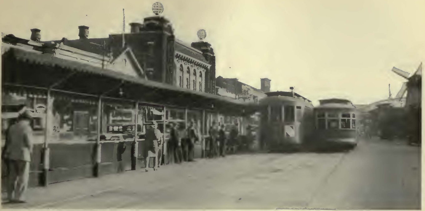
Train on the Jefferson Avenue line approaching a station. The safety zones are covered with awnings and are well protected
