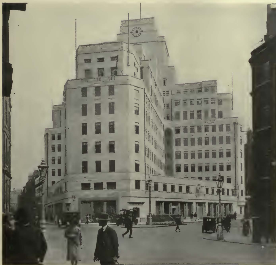
Impressive structure which houses London Underground officers and staff
