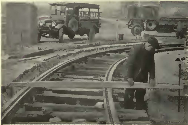
Long level board, designed by the Cleveland Railway to be handled by one man
