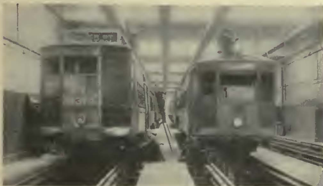
Many safety measures are in use in the Boston shops. This view shows the advantage of depressed pits with leg holes for inspection and repair work on trucks and motors
