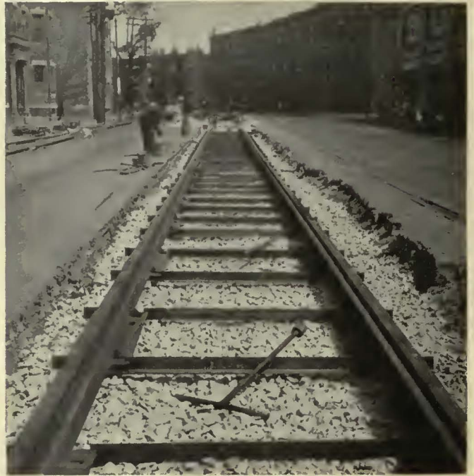
Seven-inch grooved girder rail was used with rolled-steel joint plates seam welded
