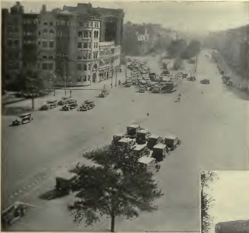
In Boston, traffic lanes are marked prominently at congested intersections
