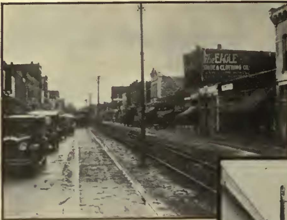
A typical "street of the past". Note the obsolete cluster-type lighting standards and the trolley poles extending down the center of the street.
