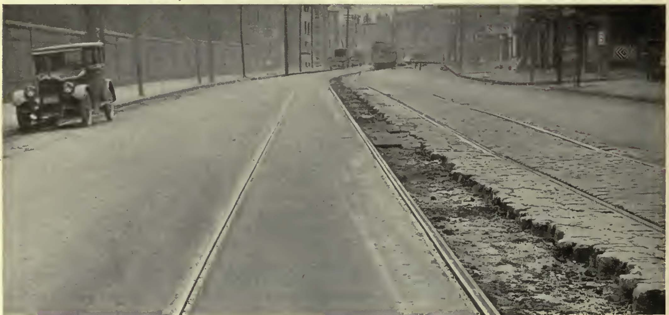
The paving surface consists of a 3-in. layer of sheet asphalt
