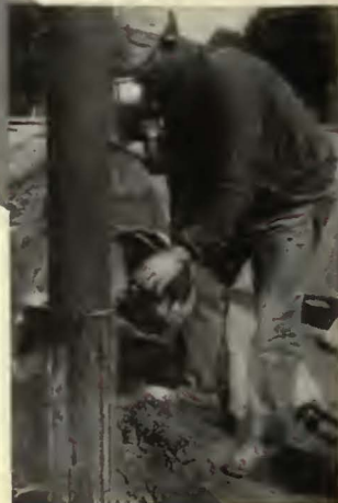
Pouring the cement. The entire space between pole and sleeve is filled.
