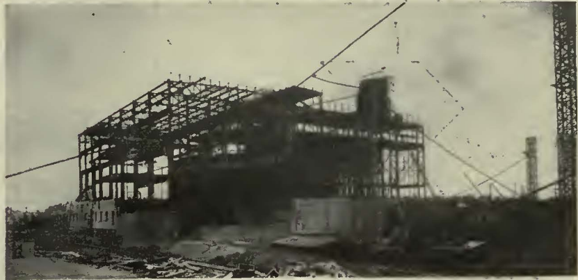
Progress Picture, Power Station
