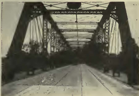
Spy Run Bridge, Ft. Wayne, Indiana, smooth-surfaced with Carey Elastite Asphalt Plank. Notice also that the rails are cushioned with Carey Elastite System of Track Insulation.
