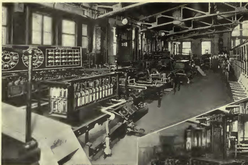
Interior of new instruction school in trainmen's room of 69th Street Terminal
