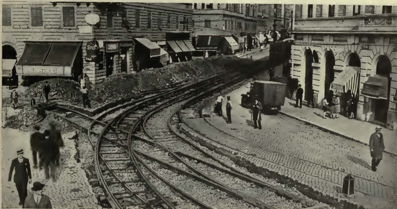
While new trackwork was installed service was continued uninterrupted over old track
