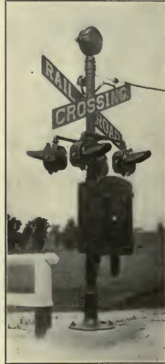
Nachod Signal on Interurban lines of the Milwaukee Electric Railway and Light Co.
