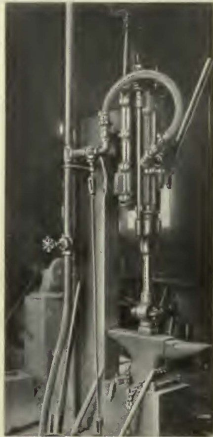
Air hammer made from an old rock drill speeds up blacksmith work in the track department of the Georgia Power Company
