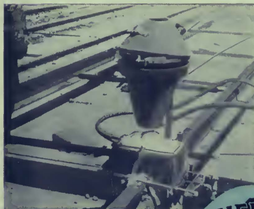
Thermit-welding Tee rail—after reaction has taken place, but before removing moulds.
