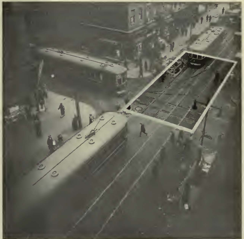
Bethlehem Silico-Manganese Crossing and Turnout installed at a busy traffic intersection in a large eastern city.
