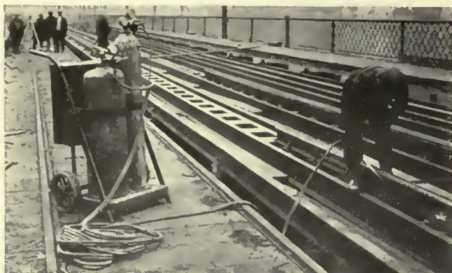
Portable truck for oxyacetylene burning outfit used by the Cleveland Railway
