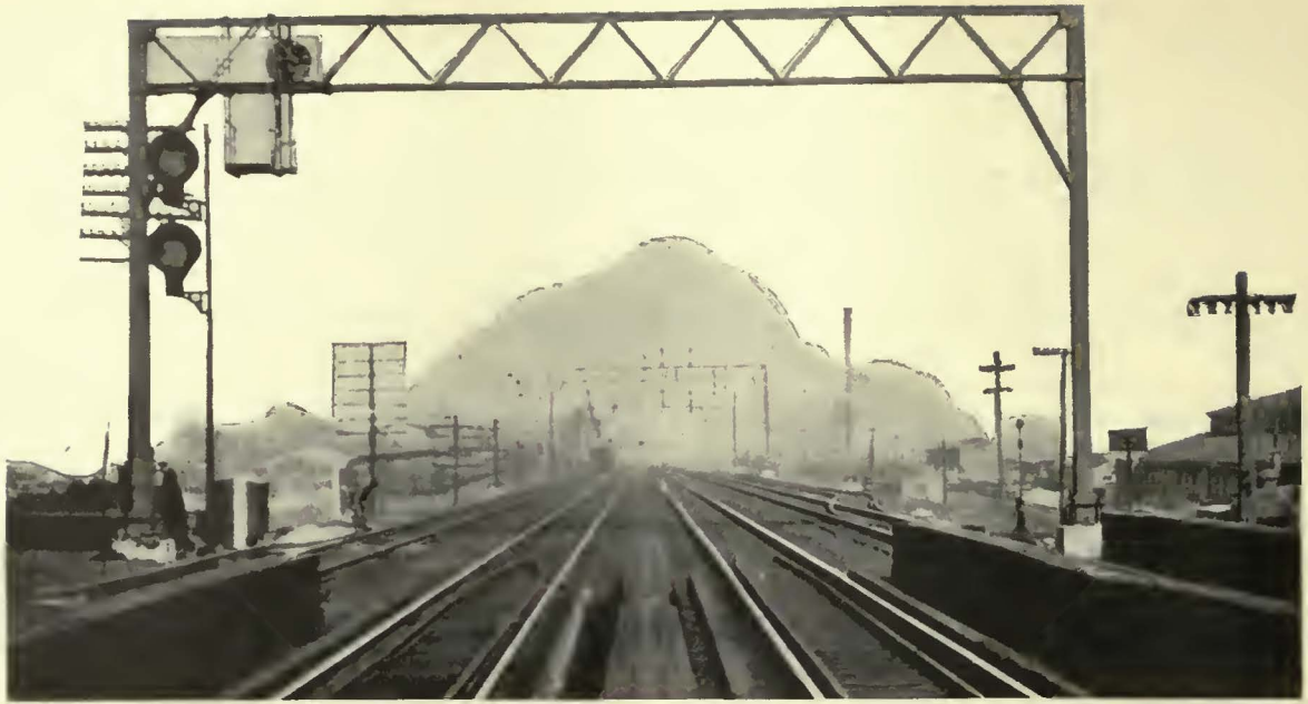
One of the four-track catenary and signal bridges. The old banjo signals seen on the mast near the left of the bridge will be removed and replaced by color light signals of the type shown supported from the bridge
