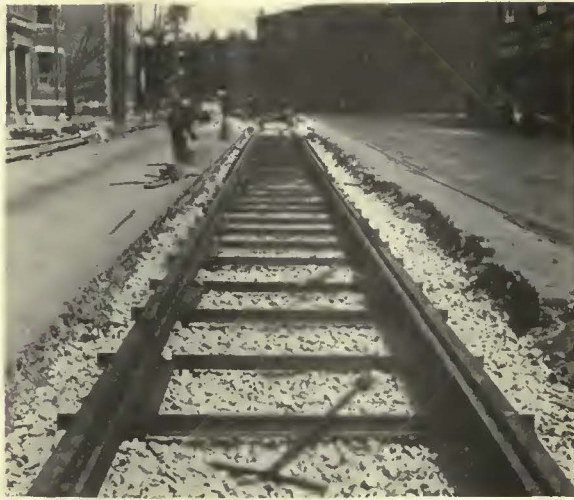
Monolithic concrete track recently built by the Boston Elevated Railway
