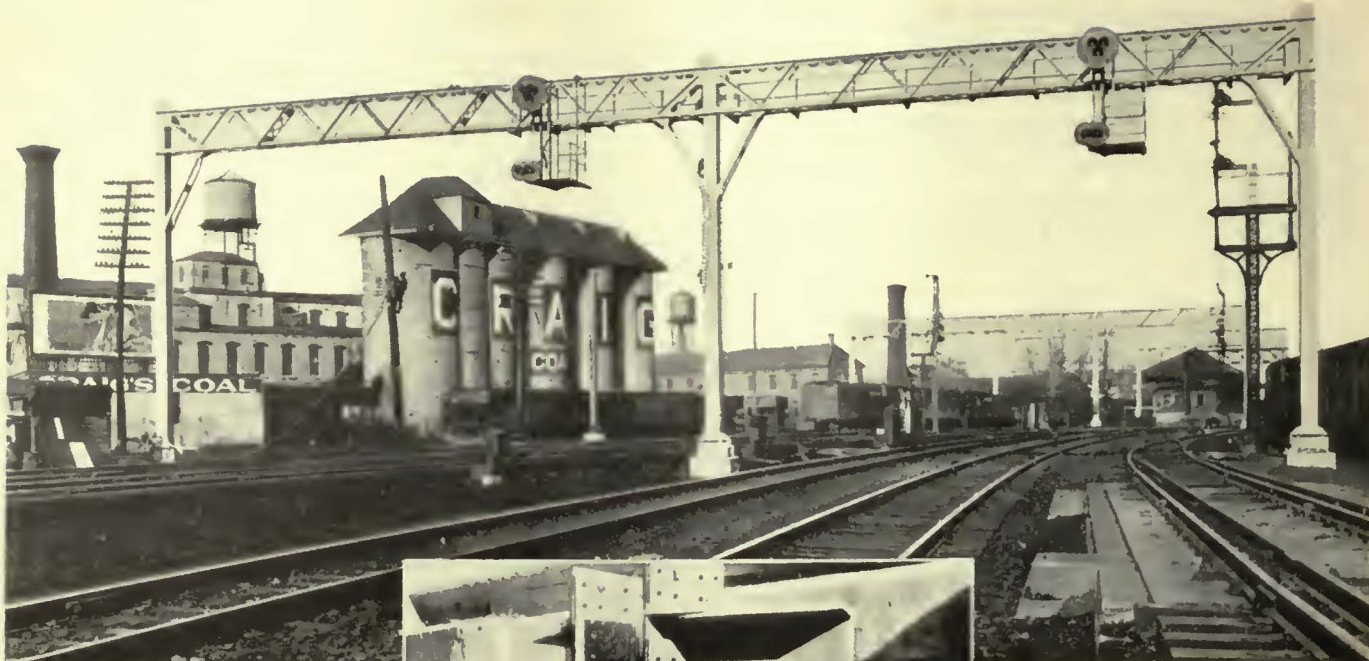
Catenary bridge with central supporting member, showing also the new signal installation
