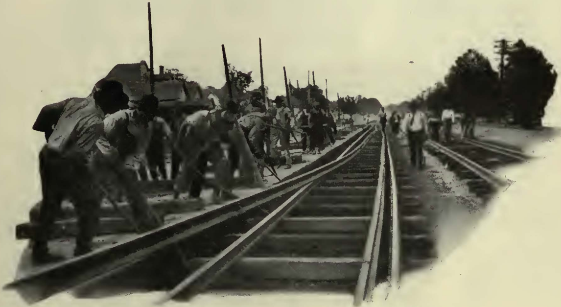
Snaking-in a long section of thermit-welded rail in Birmingham, Ala.
