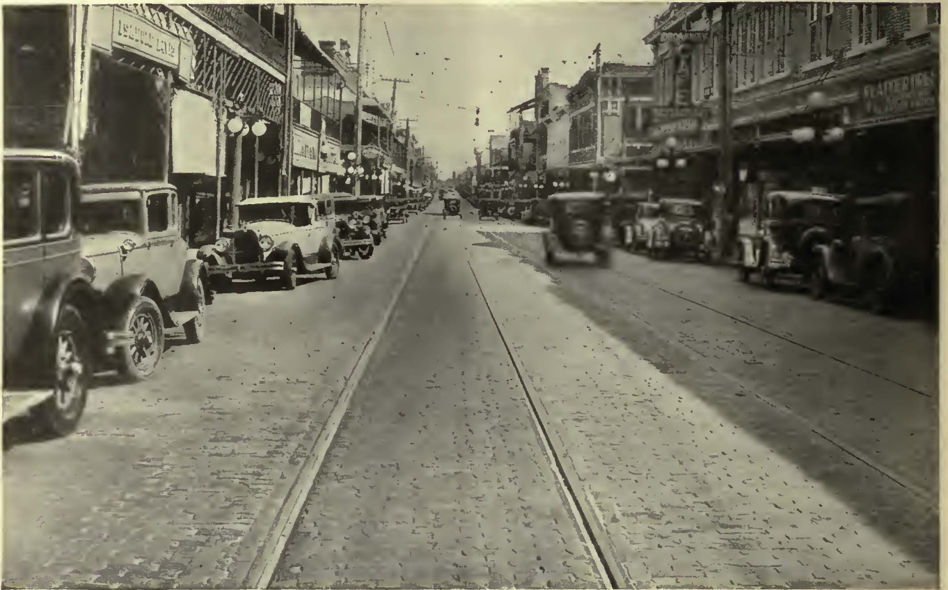
A view of The Tampa Electric Company's trackage on Seventh Avenue, Tampa, Florida. Note the excellent condition of the flangeways and the smooth expanse of brick pavement adjacent to the tracks.
