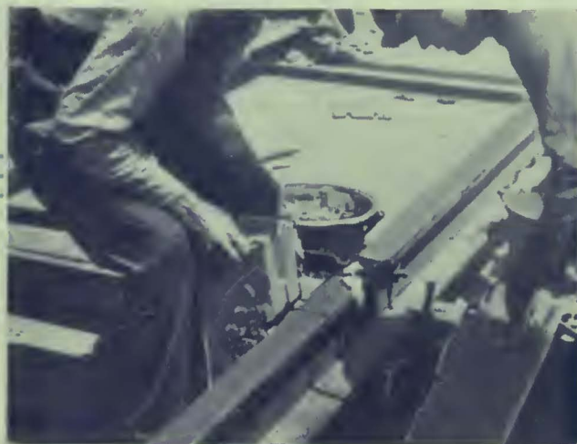
Thermit-welding Tee rail—workmen putting the moulds in place.
