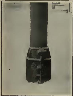
"C" Clamp Supporting Pole Corroded at Base
