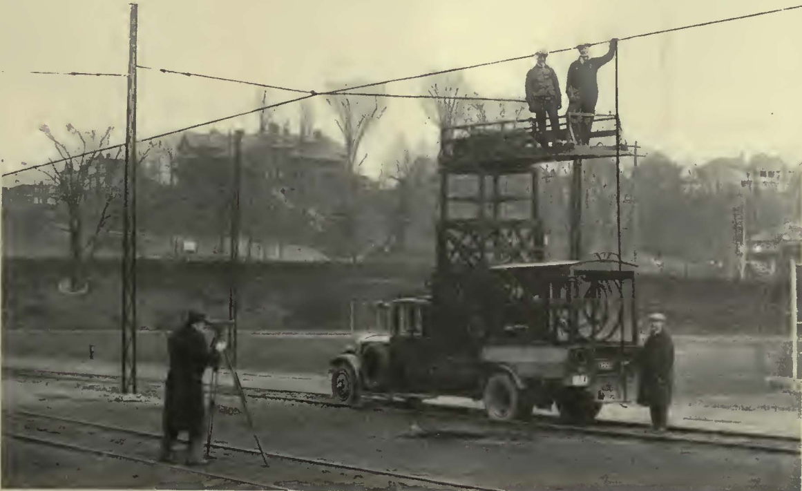
Checking up on tension of the trolley wire by measurement of the sag with a level
