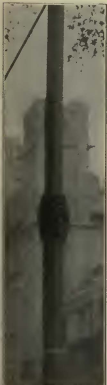
"A" Clamp Installation
