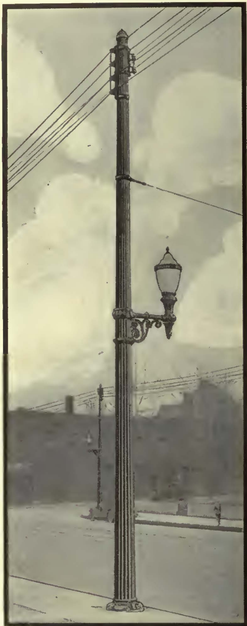
Union Metal Fluted Steel Poles installed on Market Street, Youngstown, O.
