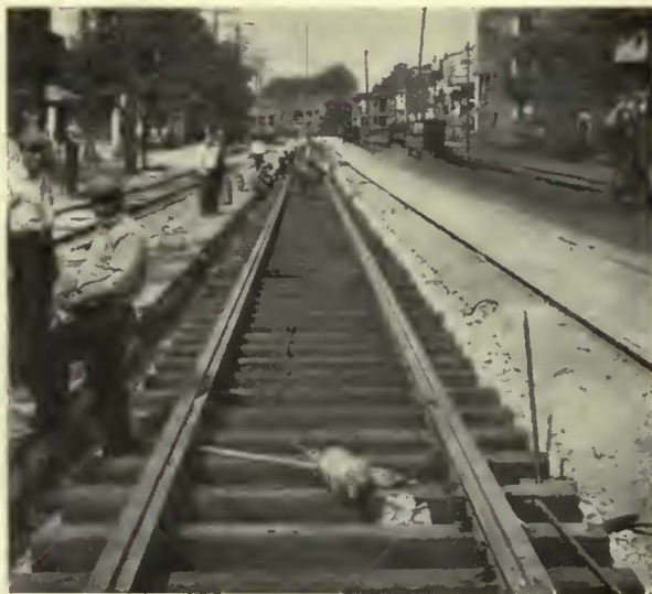
Pressure-treated creosoted wood ties are used in Cleveland
