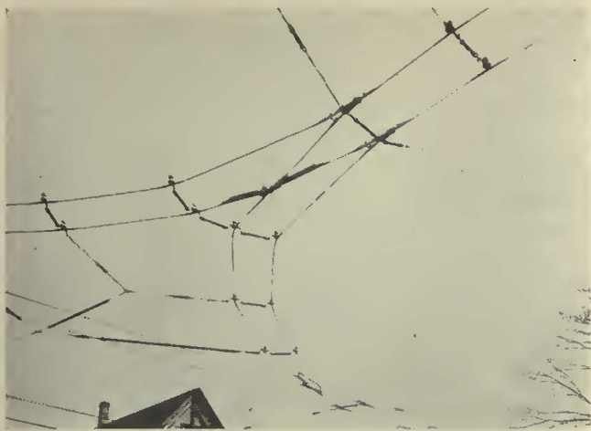
Special overhead "Y" construction at Harding and Diversey Streets
