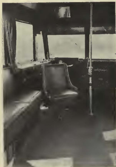
At the rear end of the car the operator's seat is swung around and made available for passenger use
