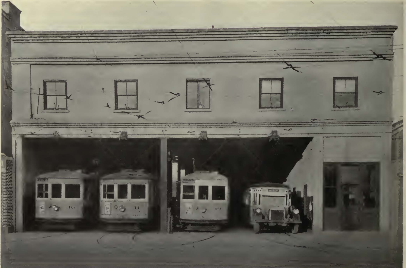
General offices, carhouse and garage are grouped in one building, centrally located on Main Street
