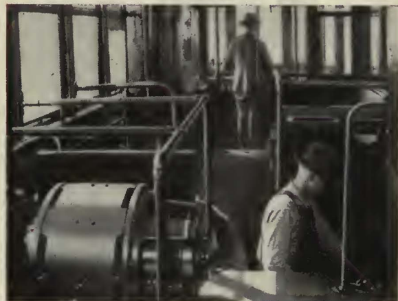
Interior view of Reciprocating Grinder Car.
