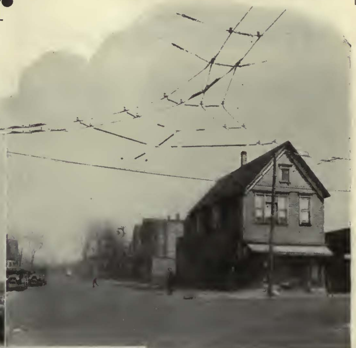
Special overhead construction at Diversey and Harding Avenues. O-B Spring Frogs, O-B Type DC Cross-overs, O-B Insulated Approaches and O-B Spring Lock Hangers were used.
