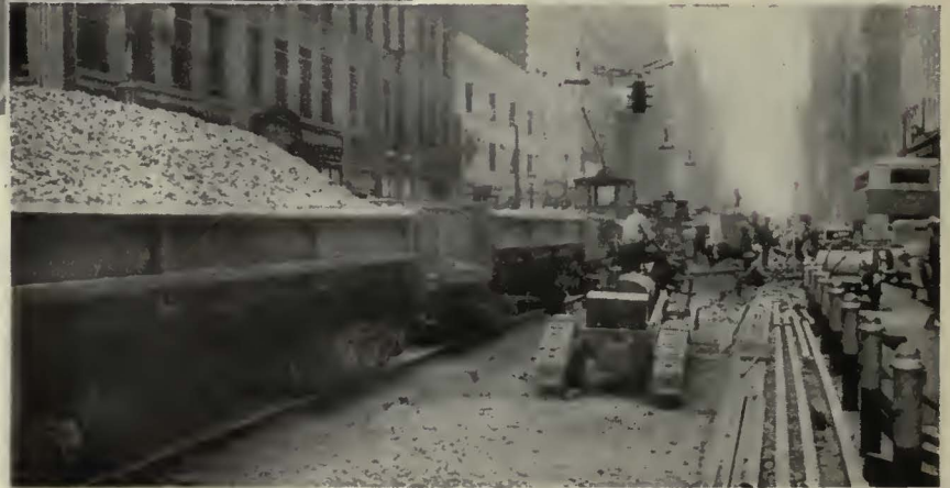
Concentration of mechanical equipment permitted speedy work
