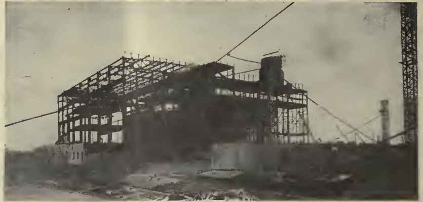
Progress Picture, Power Station
