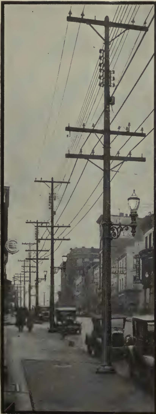
Heavily loaded Union Metal Poles serve Wheeling, W. Va.
