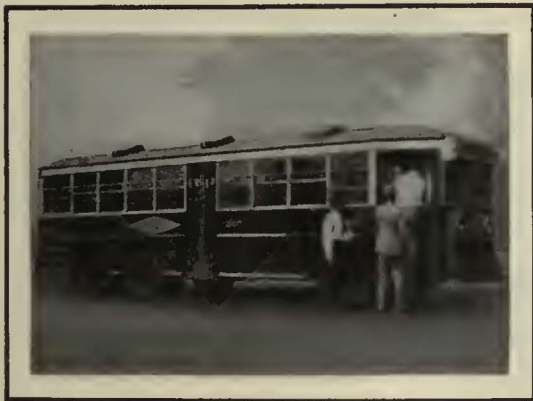
The Capitol District Transportation Company operates a fleet of 76 gas-electric buses in Troy and Albany, N. Y., where the routes are characterized by steep grades and heavy traffic. All the electric-drive equipment is of G-E design and manufacture.
