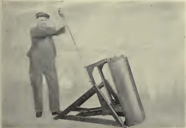
Tilting controller workbench used in shops of the Cincinnati Street Railway
