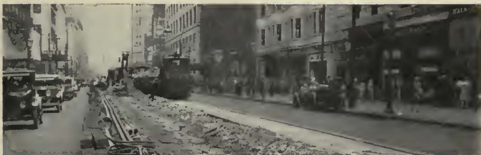
Electric shovel digging out the old track
