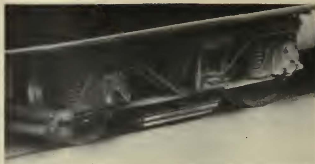
Installation of magnetic brakes between the wheels of a double truck, as used on the new Albany car
