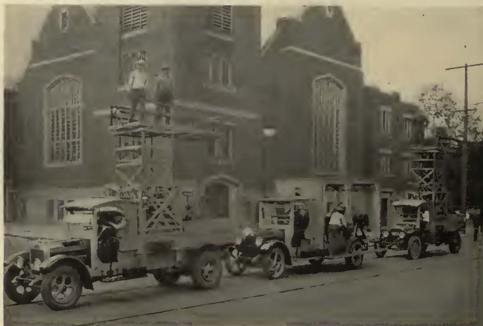
Removing old and stringing of new trolley wire in one operation
