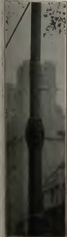
"A" Clamp Installation
