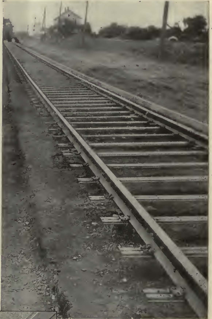
Reconstructed single-track structure with Bethlehem No. 3 Steel Ties.
