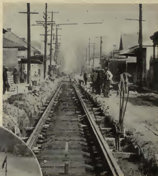
Combination steel and wood ties are used by numerous railways
