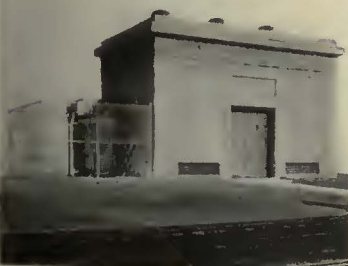
Pine automatic substation of the Northwestern Pacific
