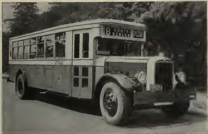
A G-E equipped gas-electric bus of the Public Service Coördinated Transport, Newark, N. J. The ability to increase schedule speeds has always been an outstanding advantage of gas-electric drive
