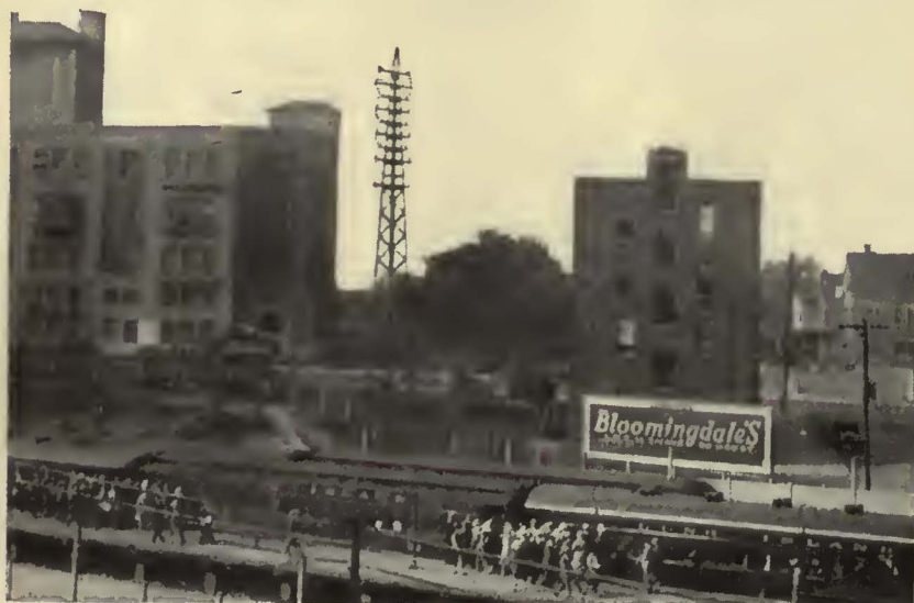
Woodside, one of the principal junction points on the Long Island Railroad, uses flush platforms
