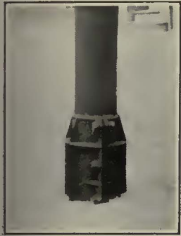
"C" Clamp Supporting Pole Corroded at Base
