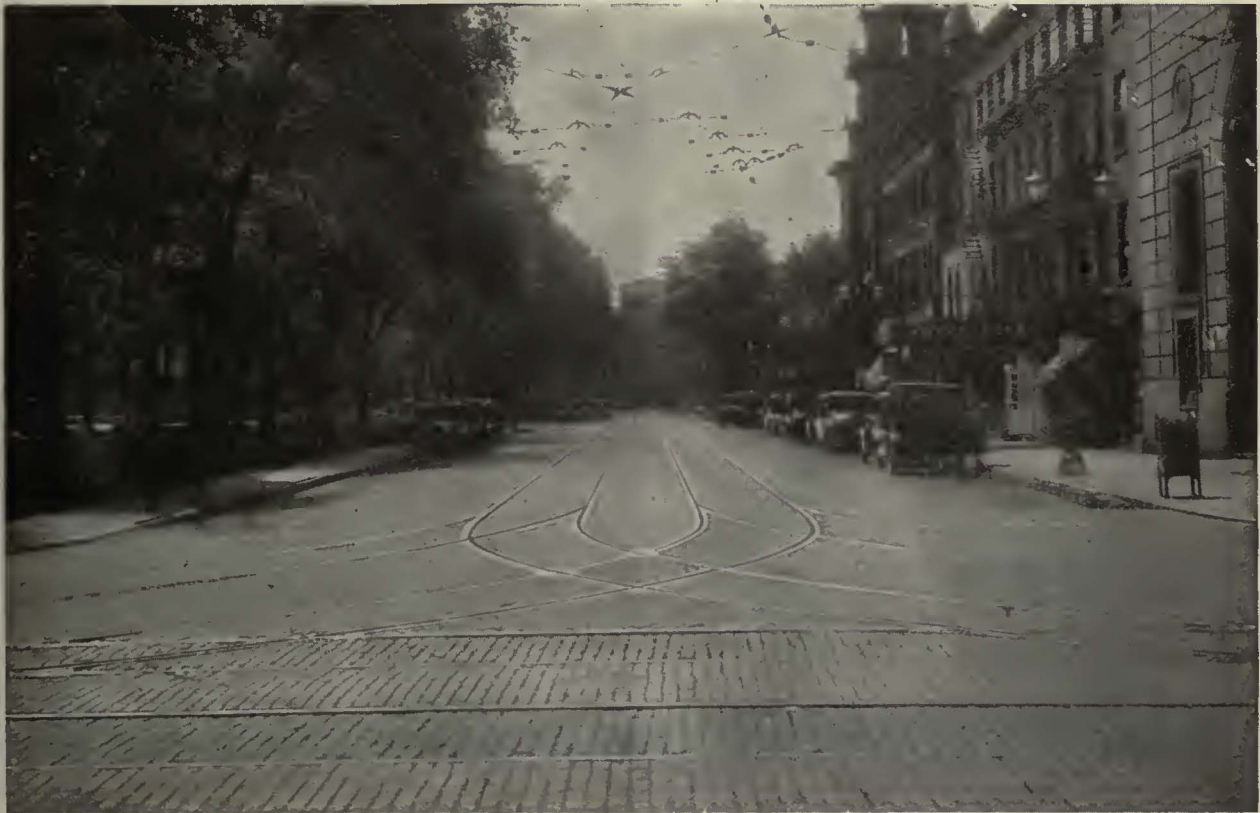
Looking south on Court Street, Elyria, Ohio. The track is protected with Carey Elastite System of Track Insulation, which forms a water-tight seal between the paving and the rail. Installation supervised by J. M. Powell, City Engineer.
