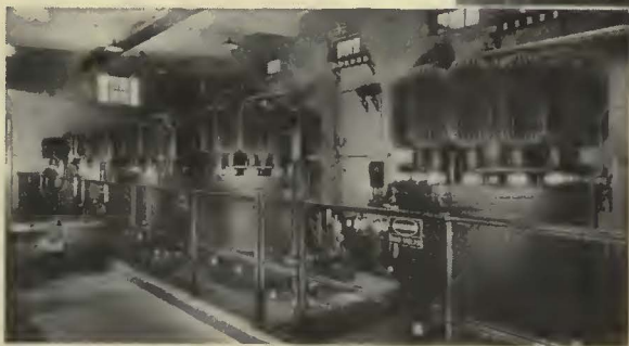
Mercury arc rectifier substation equipment for 600-volt d.c. service. Above—Installation of the Long Island Railroad at Hempstead. At left—Equipment of the Connecticut Company at Bridgeport
