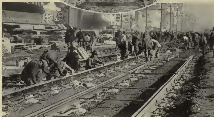
Experimental track built on rail seats without ties
