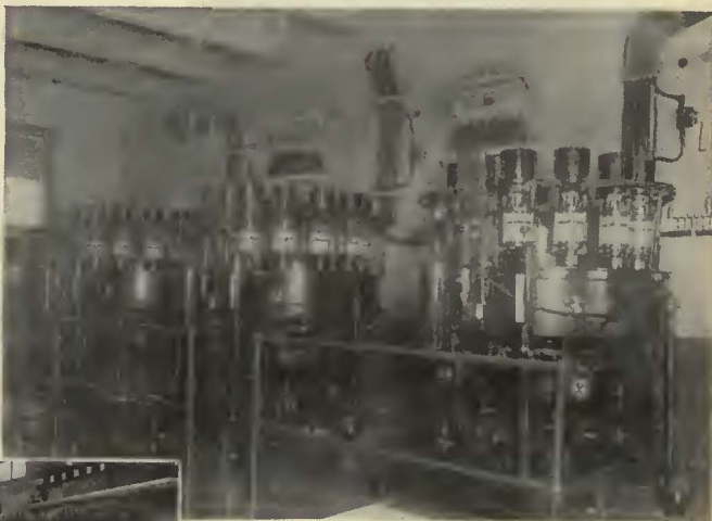
Mercury arc rectifier substation equipment for 600-volt d.c. service. Above—Installation of the Long Island Railroad at Hempstead. At left—Equipment of the Connecticut Company at Bridgeport
