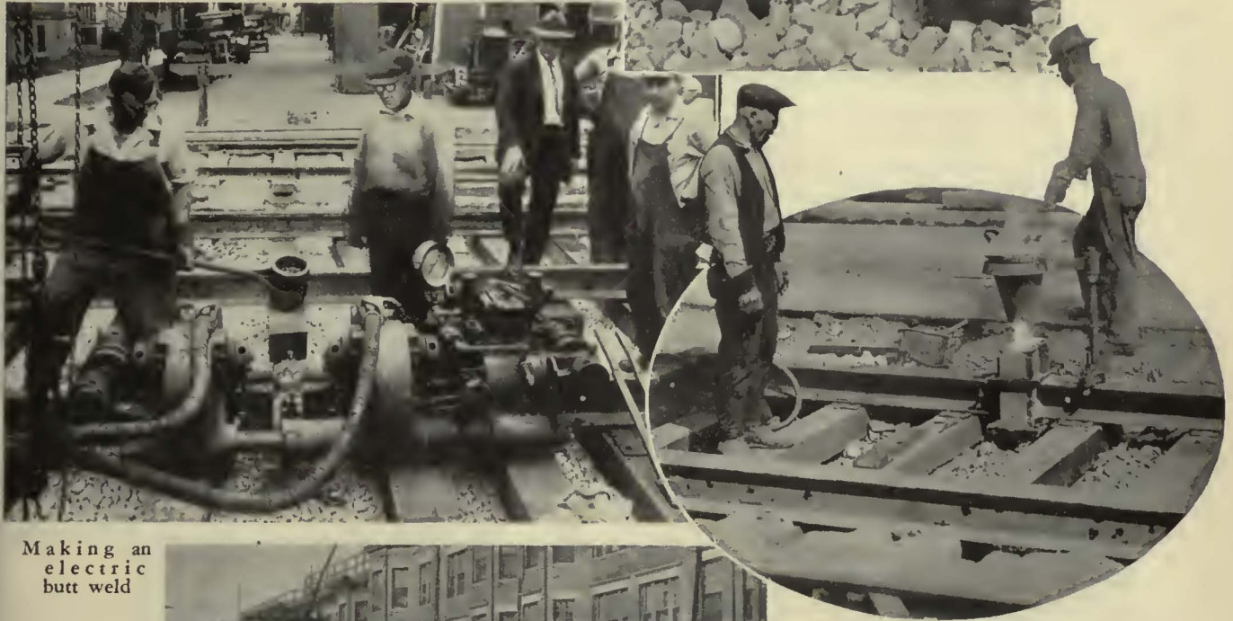
Thermit welded joints are widely used
