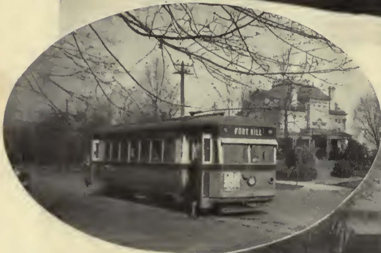
The square front of this Lynchburg car affords good vision for the operator and also makes possible the most efficient use of the available space
