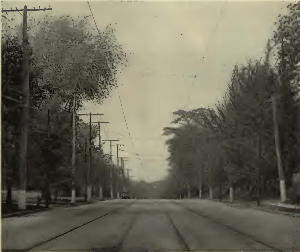
The rail has recently regained a considerable amount of its former popularity for use in street railway track with concrete paving
