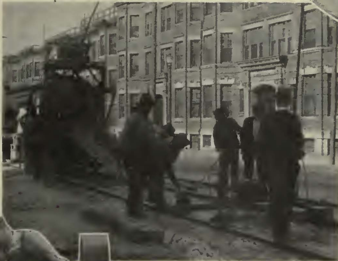
Vibrating track concrete to give added strength
