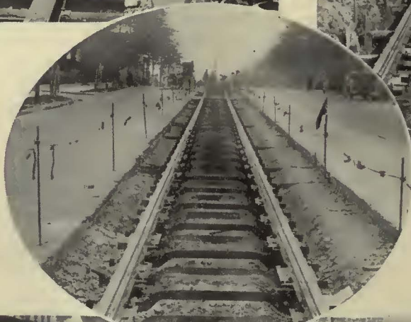
Grooved girder rail on wood ties is widely used in track construction
