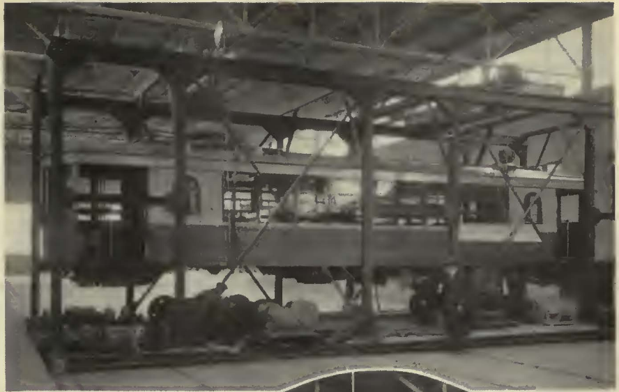
With the overhead hoist built into the transfer table structure two men can exchange shift trucks for overhauled motor trucks
