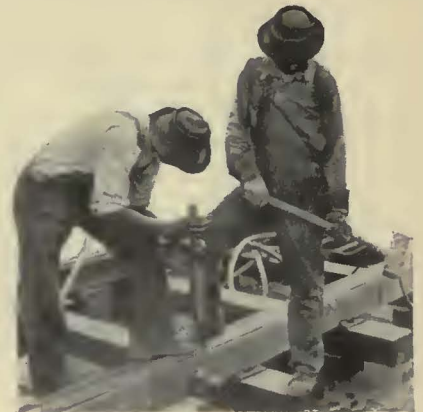
Reciprocal rail grinder mounted on car
