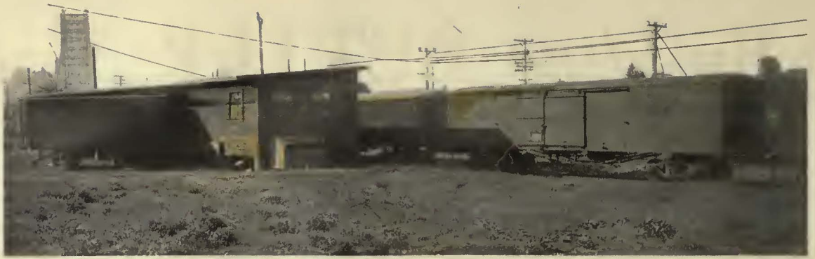
Fig. 13—Railway truck line transfer station of the Lake Shore Electric Railway, Toledo, with a "spot" capacity of four cars
