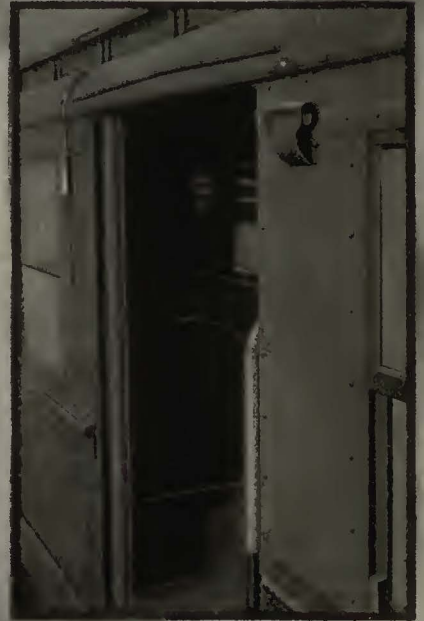
Door detail showing signal light and safety buffer
