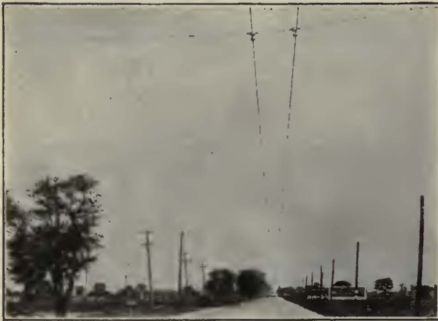
Overhead construction for Trolley Bus service on Plymouth Road, in the northwest portion of Detroit. A combination of O-B Spring Lock Hangers and O-B Type B Hangers, with O-B Marathon Ears, support the overhead.
