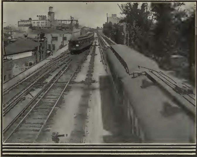
A view of the right-of-way of the Chicago Rapid Transit Co., Chicago. This property is an extensive user of Una Rail Bonds.
