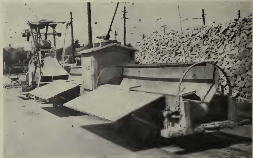
Belt conveyor used by Cleveland Railway for loading concrete mixer saves 53 per cent in labor
