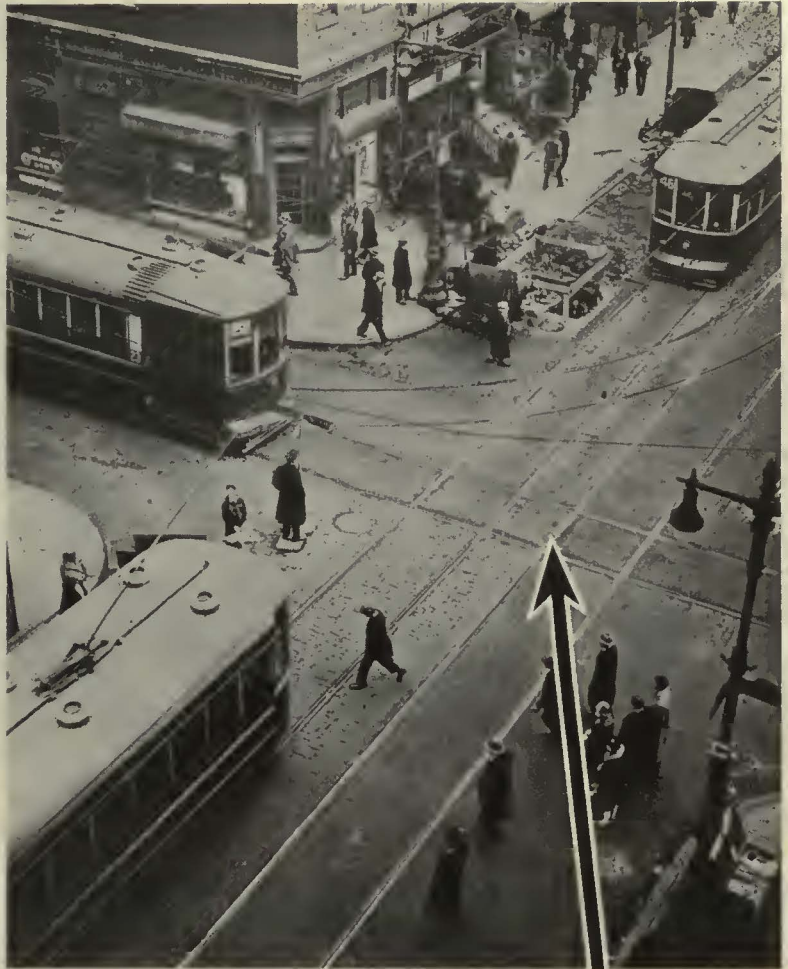
Bethlehem Silico-Manganese Weldable Crossing and turnout at 10th and Arch Sts., Philadelphia, Pa.
