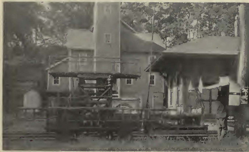
In the yards and on the branch lines gas rail tower cars are used
