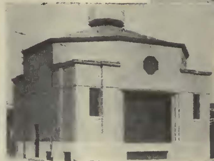
Below—Exterior view of the Turner substation.
