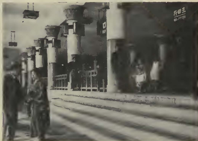
White Tile, Electric Direction Signs and Modern Lighting Fixtures Are Features of the Kobe-Arima Railway Station
