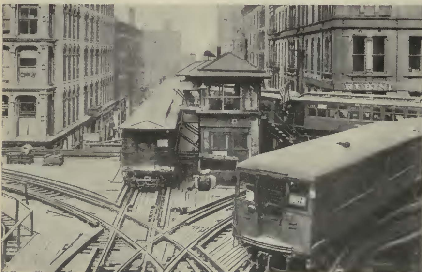
This intersection at Lake and Wells Streets, the northwest corner of the Loop, is said to be the busiest railroad crossing in the world. In the maximum hour, 224 trains of 1,244 cars pass through it
