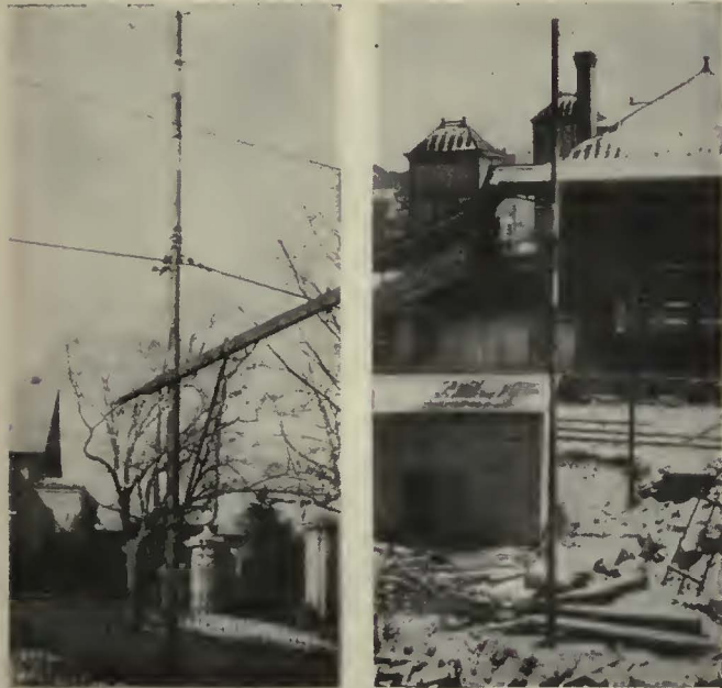
At left—Pole lengthened by splicing to support horizontal arm for attaching trolley wires on Webster Avenue. At right—Extra long pole made by splicing two ordinary poles together with reinforcing clamp
