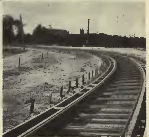
Keystone No. 9 Steel Ties used in construction of curve.
