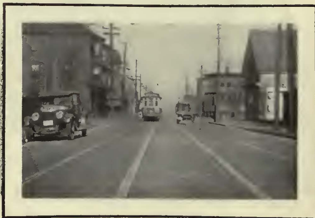
Many of the double track lines in Providence operate along narrow streets. This is Eddy St., 34 ft. between curbs where track was laid in 1930.
