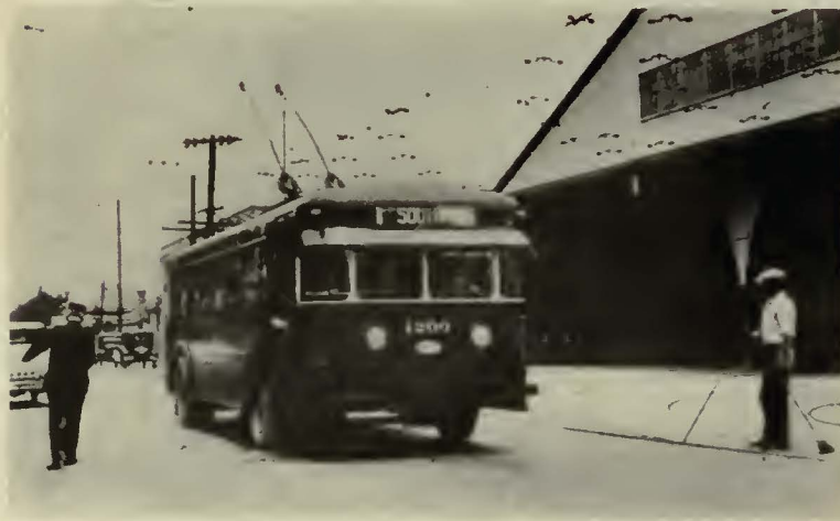
New Orleans trolley bus in front of the Carrollton shops, where the vehicles are maintained
