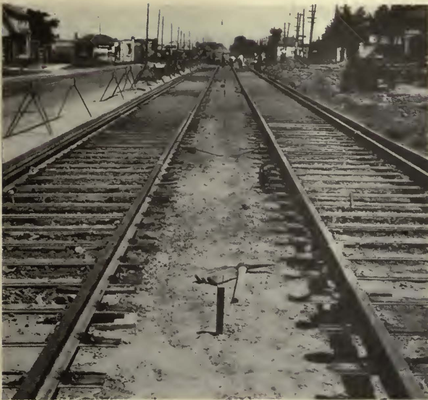
Double track construction with Bethlehem No. 3 Steel Ties.
