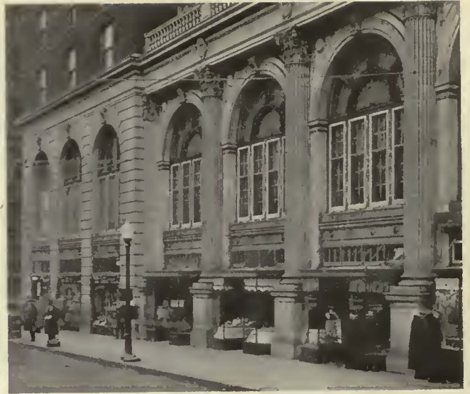
Section of East Fifth Street where span wires are attached directly to the walls of the Hotel Gibson
