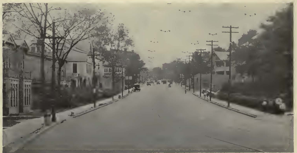
Improved appearance of Reading Road after installation of joint poles and elimination of those no longer needed
