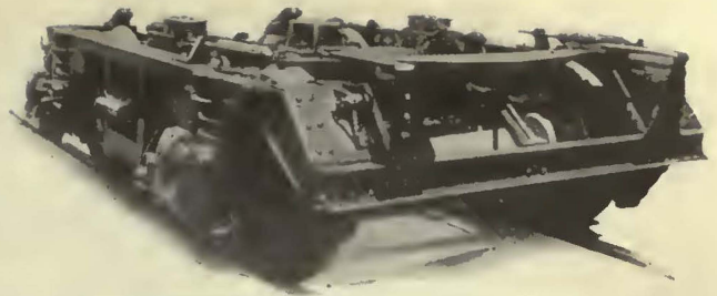
Each car has one trailer truck of the type shown. All wheels have clasp brakes
