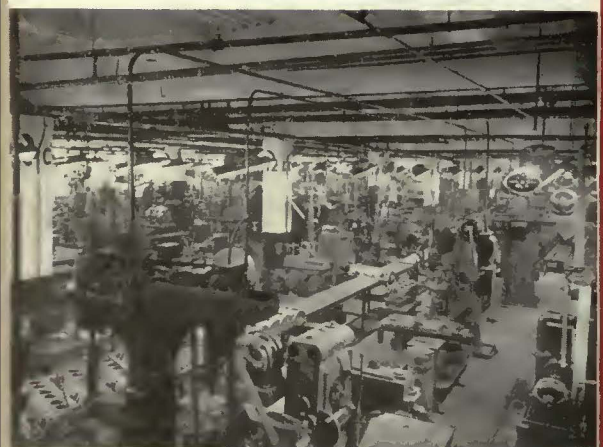
The plant is completely equipped with all modern labor-saving and material handling devices. Work in process progresses directly and automatically from one production or assembly line to the next.
