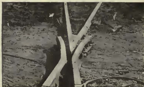
Same frog after being welded with TIMANG Manganese Welding Rod in the track.
