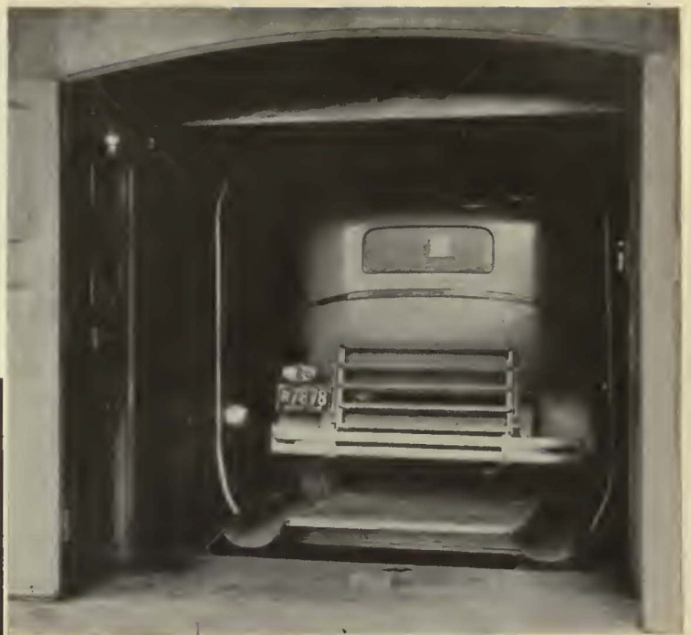
Above—Individual cradles and an automatic control are features of this new method of storing automobiles
