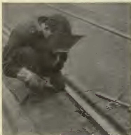
O-B Titon Bonds require only a one-inch space alongside the rail for application.
