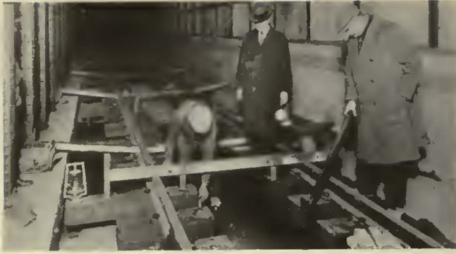
Leveling and spacing ties
