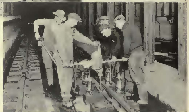
Jacking up the rails for placing ties and tie plates
