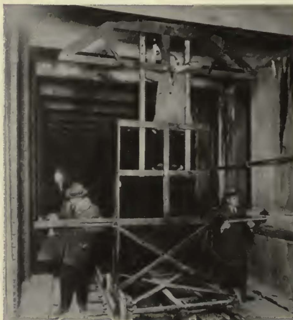
Checking for car clearances with full-sized templet
