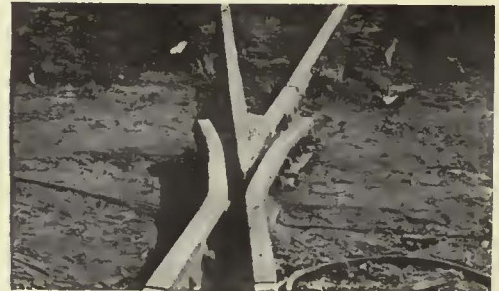
Same frog after being welded with TIMANG Manganese Welding Rod in the track.
