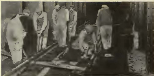
Spading and troweling concrete in the trackways
