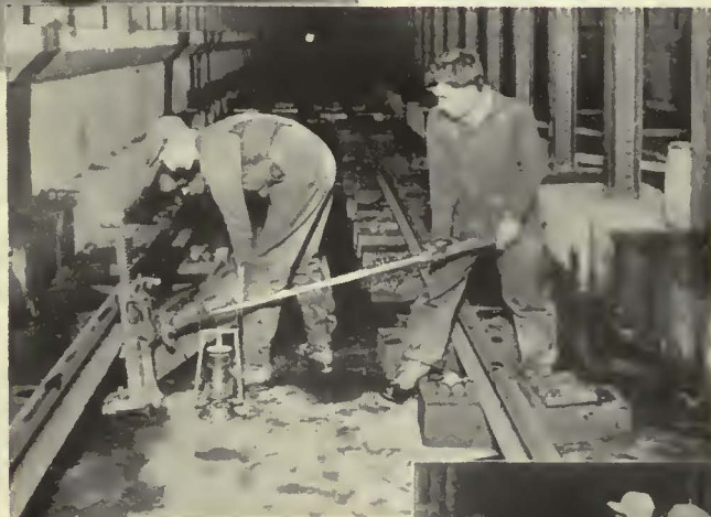
Jacking up the rails for placing ties and tie plates
