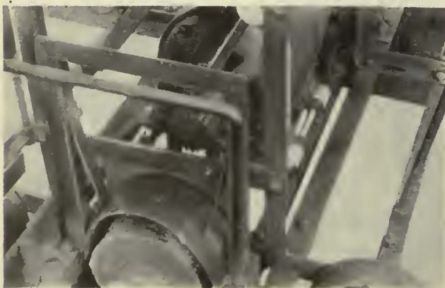
Attachment by hinges facilitates grinding motor alignment
