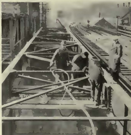
New station under construction for Chicago's rapid transit system
