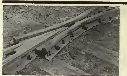
Plain bolted frog which had been worn out; and quickly reclaimed by welding with TIMANG.
