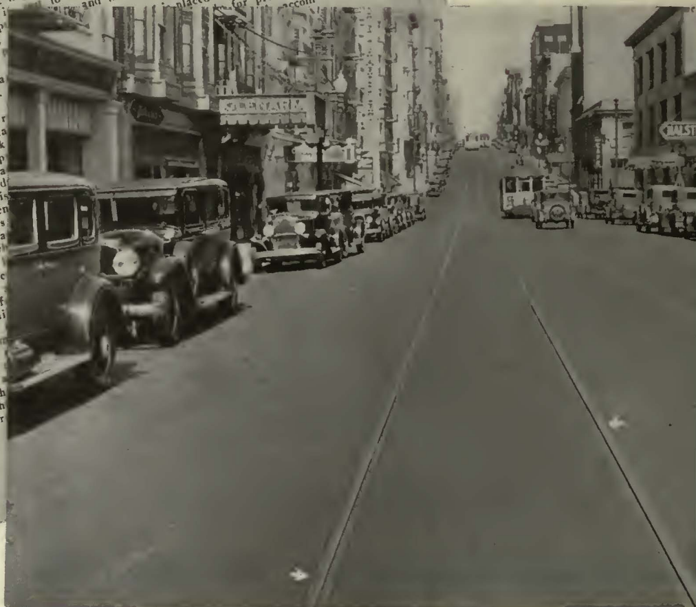
View on Sutter Street, San Francisco, taken May 27, 1931, after reconstruction had been completed. White arrows show location of two Thermit welded rail joints in foreground.
