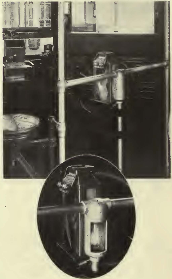
The fare box on cars of the Ottawa Electric Railway is illuminated by a lamp placed in a housing on the supporting stanchion
