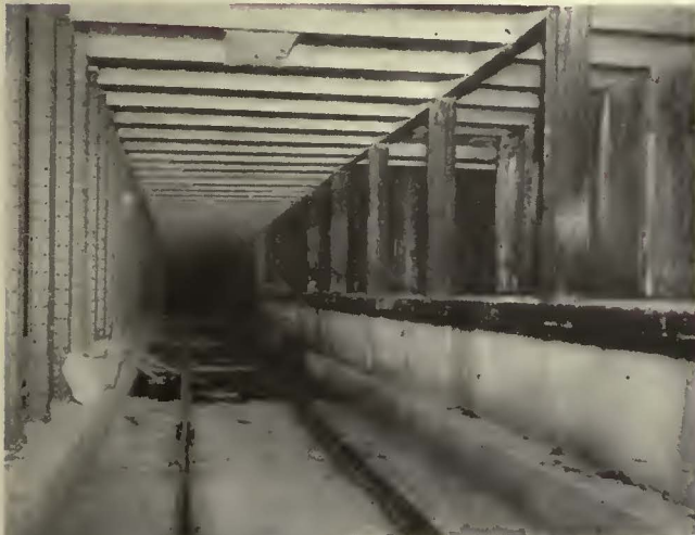
Rails bolted together and laid loosely in the trackway
