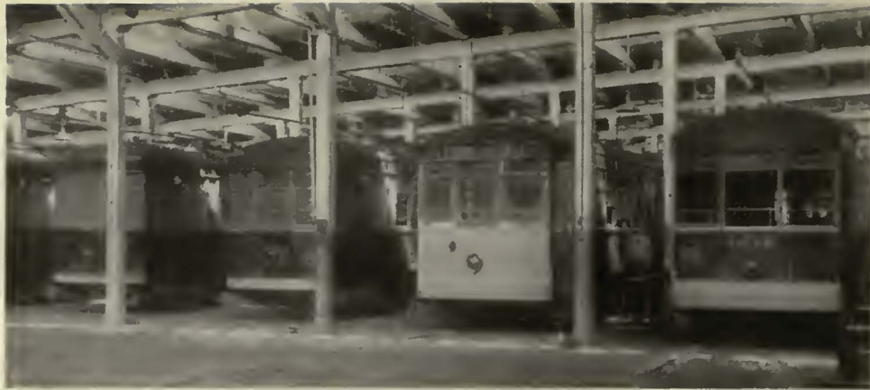
Six tracks with two cars on each track are required for washing, sanding, glazing, painting and trimming operations on a schedule of two cars finished daily
