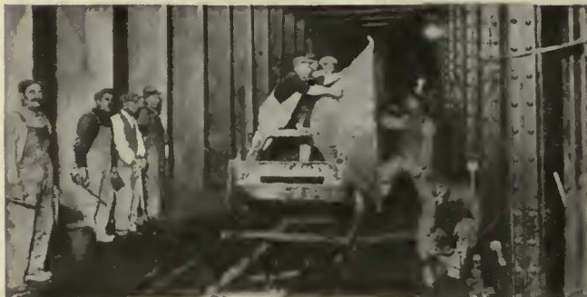
Concreting begins at both ends of section and progresses toward the center
