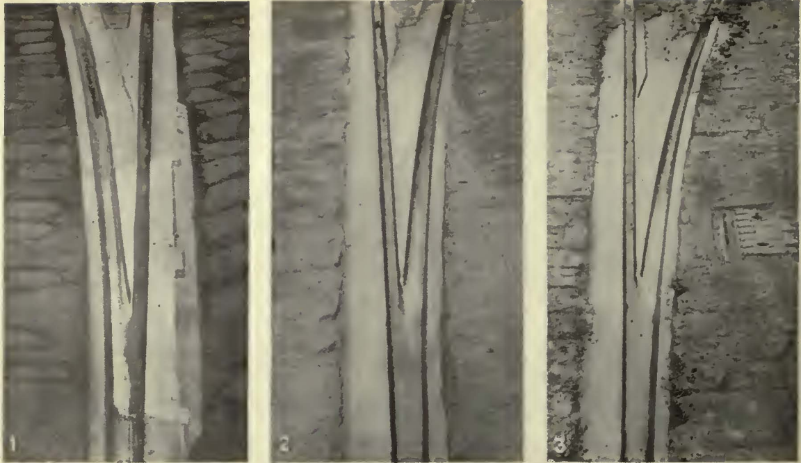
Results of Wear on Open-Point Mates in Cleveland
