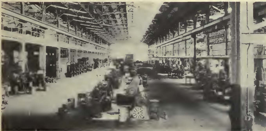
Machine shop for car and bus repairs. On the mezzanine floor is the sheet metal shop
