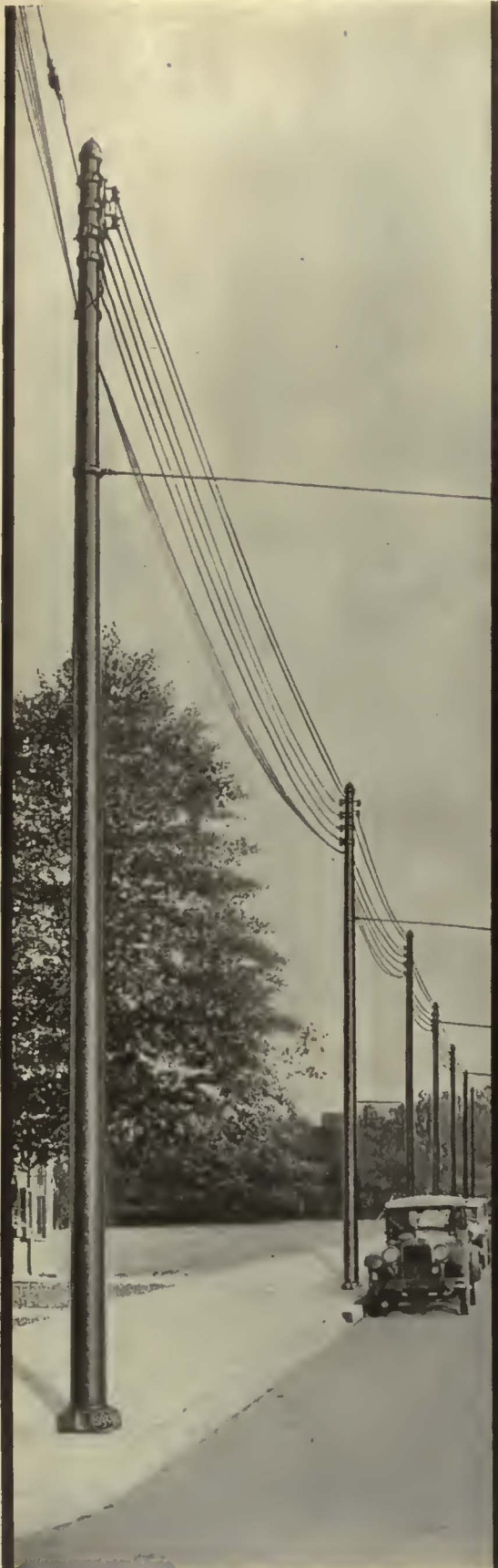
Monotube Pole with ornamental base used for distribution lines and trolley span wire support.
