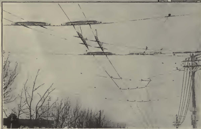
A portion of the overhead trolley bus system at Christchurch showing the wide use of O-B line material. O-B crossovers, insulators, spring-lock hangers, and Marathon Ears figure prominently in the construction.
