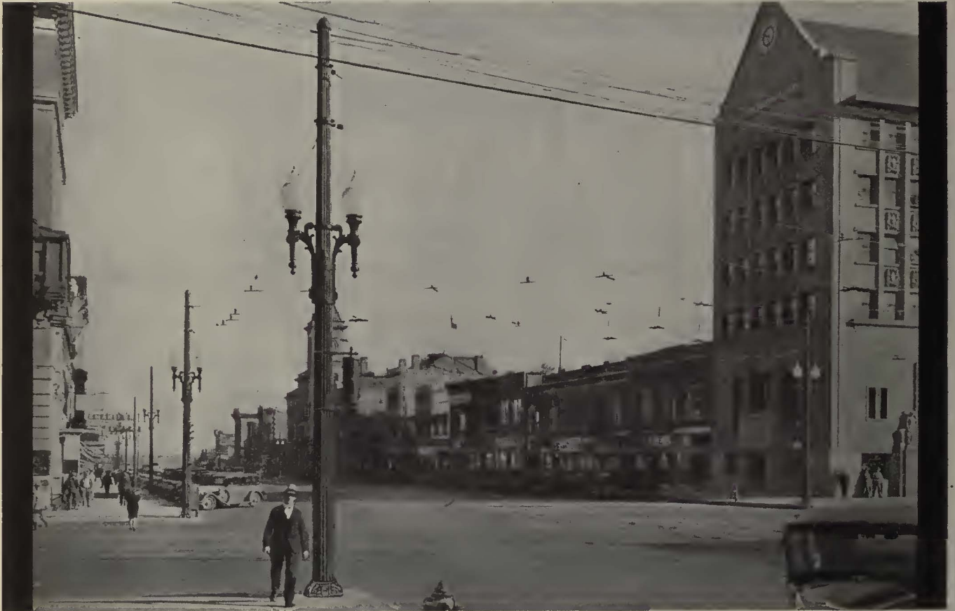
In Topeka, Kas., Union Metal Poles support trolley span wires, street lights and traffic signals. Note absence of guy wires
