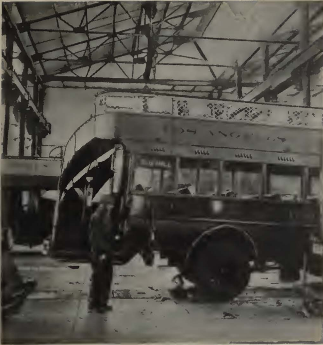
Cranes are employed to raise the rear end of a bus undergoing repairs
