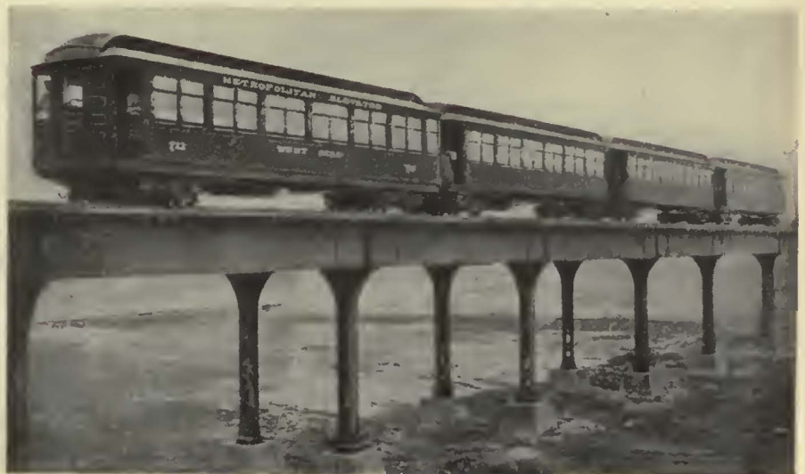
The Metropolitan Elevated in Chicago was the first rapid transit line to adopt electricity. Its advantages were quickly demonstrated and other lines were converted to electric operation
