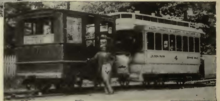
On some of the early installations small electric locomotives were used to draw the passenger cars
