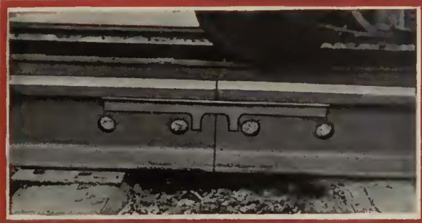
The above shows Joint Shim in position with angle bar removed.
