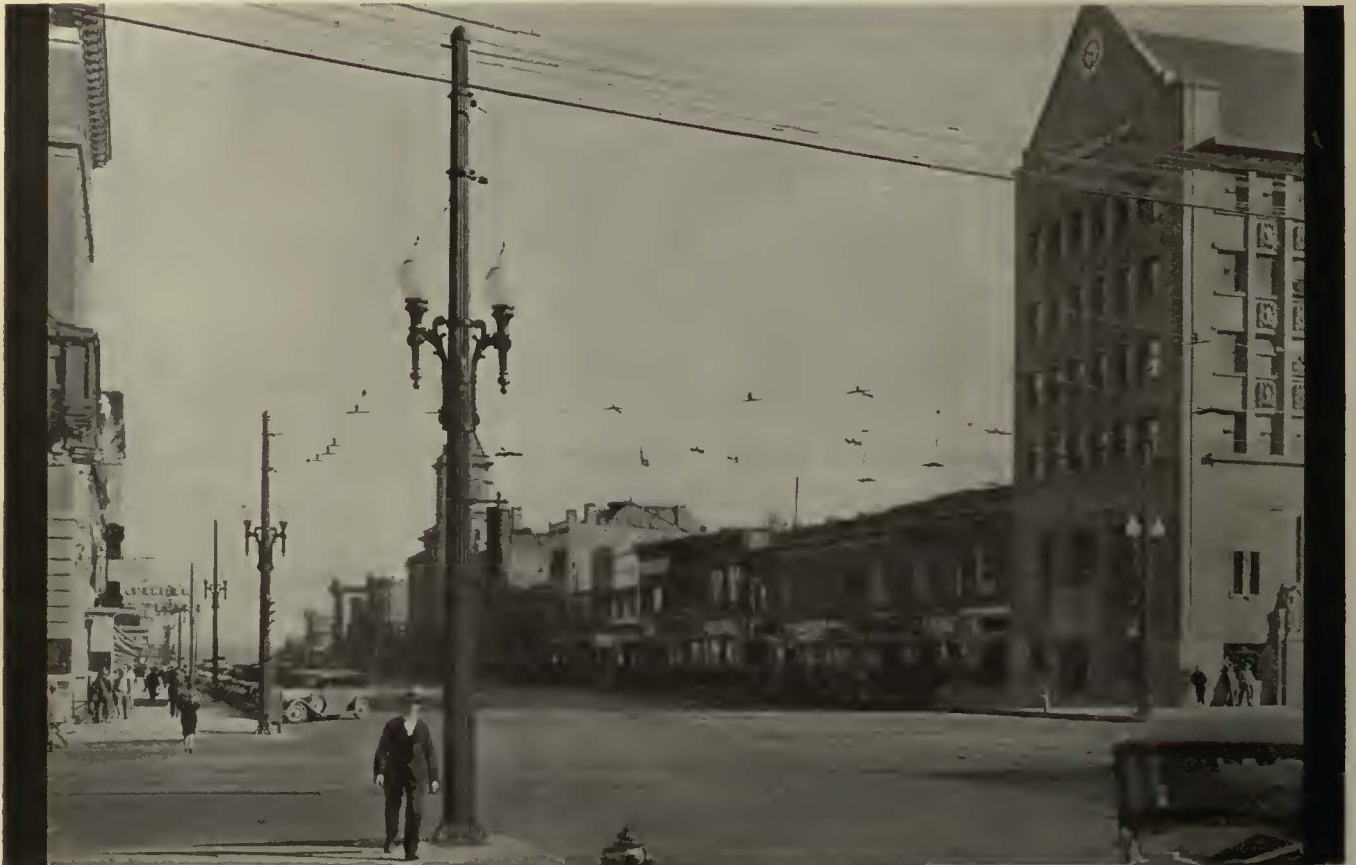
In Topeka, Kos., Union Metal Poles support trolley span wires, street lights and traffic signals. Note absence of guy wires
