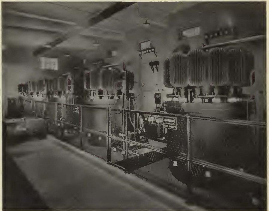
Mercury arc rectifiers are a feature of many modern substations
