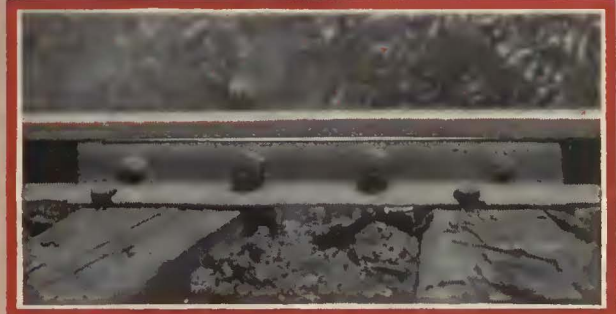
The above shows Joint Shim in position between Bar and Ball of Rail.
