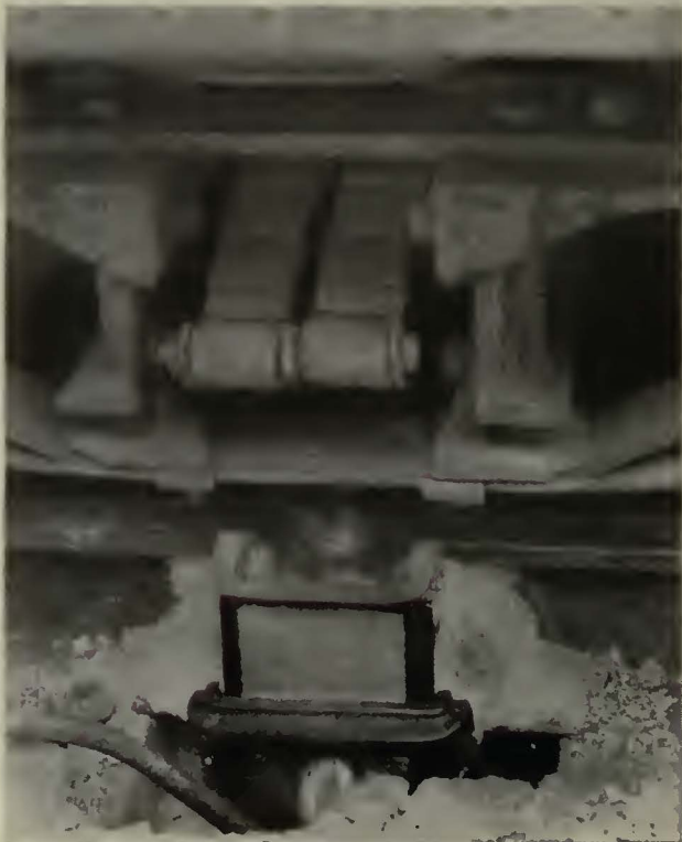
Car operating over joint during preheating
