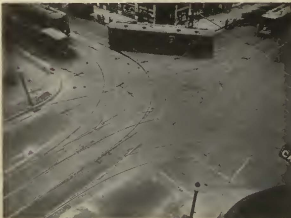
This Bethlehem "Grand Union" has been installed over 10 years at an important traffic intersection in an eastern city.
