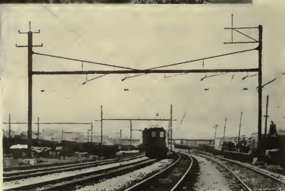
When the Great Northern rebuilt its line through the Cascade Mountains, the electrification was revamped also and extended to cover a greater portion of the route
