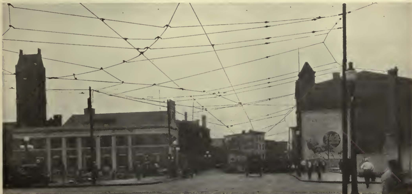
Complicated track layouts require careful treatment of the suspension fittings to produce good appearance of the overhead
