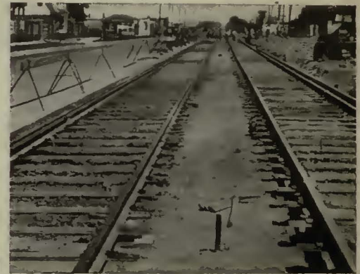
Bethlehem No. 3-A Steel Ties used in double-track construction in a large mid-western city.
