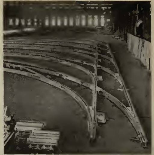
Special car barn layout assembled before shipment in one of Bethlehem's spacious shops.
