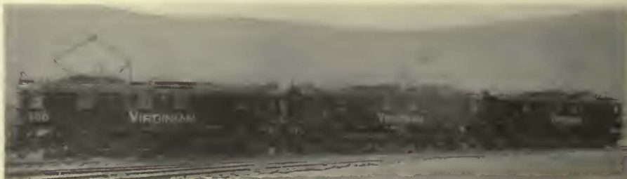
These three-cab locomotives haul 9,000 tons of coal on the Virginian Railway
