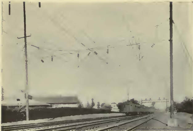
At right—Double catenary construction was a feature of the original New Haven electrification out of New York
