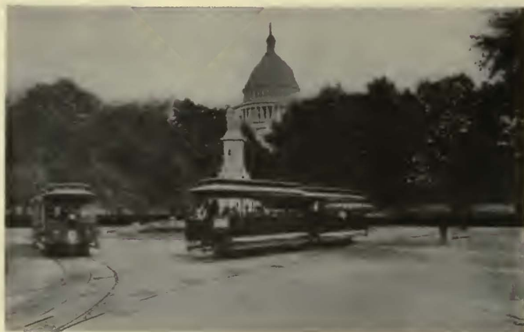
Washington, D. C., in the early nineties, showing the underground conduit system, which is still used there and also in New York City
