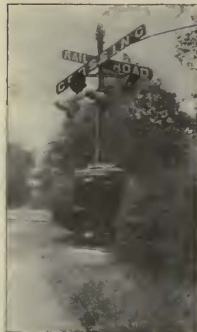
Flashing Lights With Battery Case
