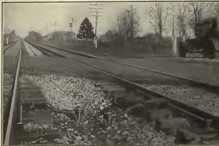
Two Directional Fusticlo Rail Contactors Used as Combination Cut-Outs and Starters. Also Shows Parkway Outlets.
