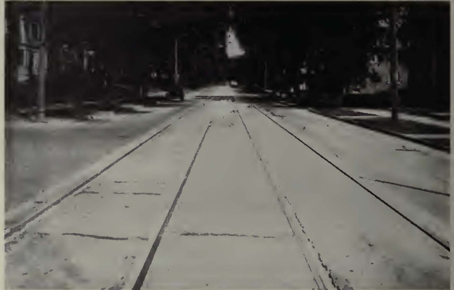
Wells Street, Milwaukee, between 28th Street and 33rd Street. This photograph shows excellent condition of track and pavement six years after laying.
