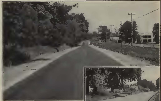
(Above) Completed brick resurfacing of worn concrete by Illinois State Highway Department on Route 4 south of Springfield. This gives the highest type highway at low cost.
