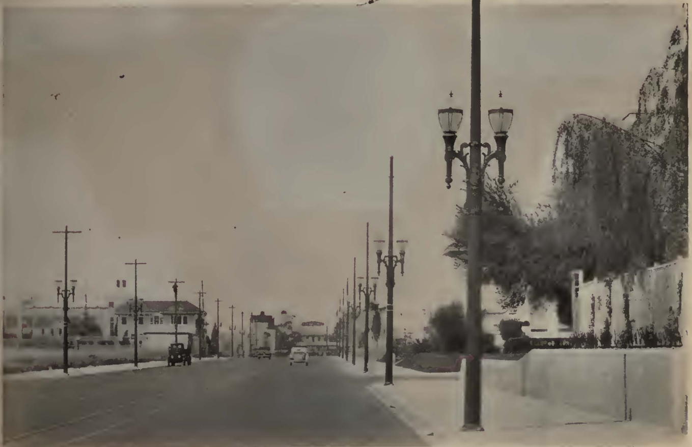
In Los Angeles, Union Metal Poles support trolley span wires, street lights and distribution lines.
