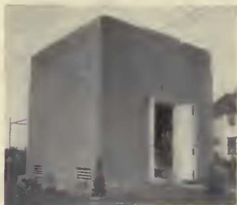
Exterior of one of the substations
