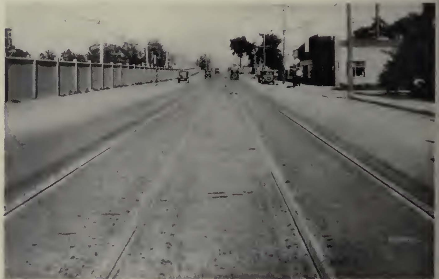
Greenfield Ave., Milwaukee, nine years after laying of track and paving.
