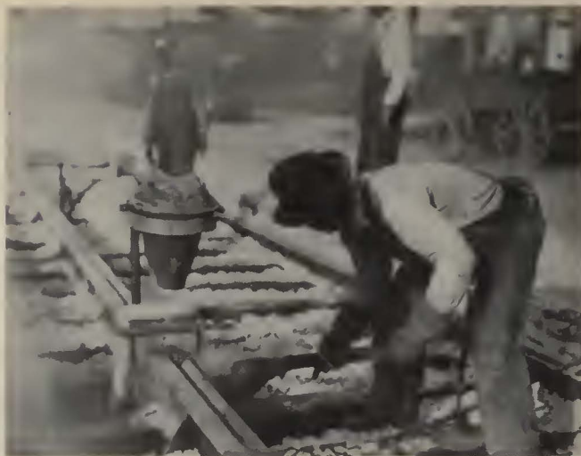
Thermit welded joints are used on all track construction at Atlanta
