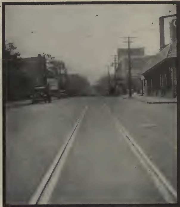
With Thermit welded joints, Atlanta's track is smooth and unbroken by bad joints.
