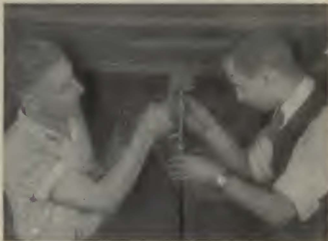
Measuring deflection of car underframe with inside micrometer caliper as the load within the car is varied
