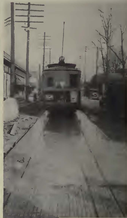
Cars operating over newly laid track, built under service with the aid of a concrete pulsator
