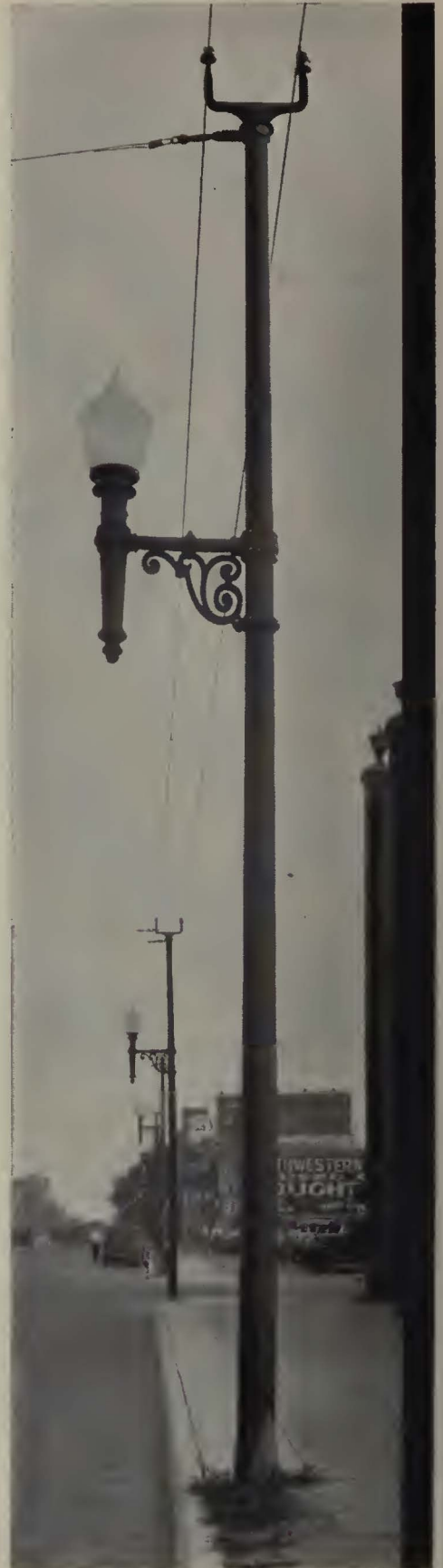
● Monotube Poles Installed in Denver, Colorado
