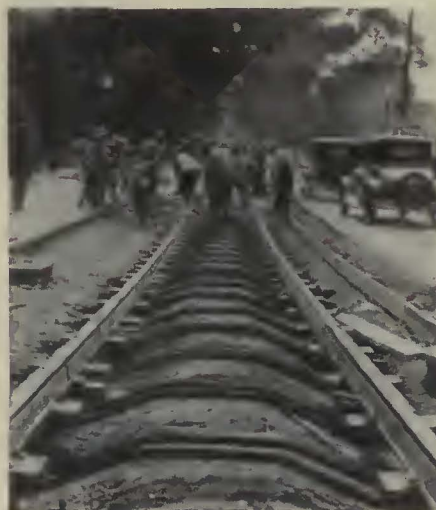
Section of track being rebuilt with Dayton mechanical ties
