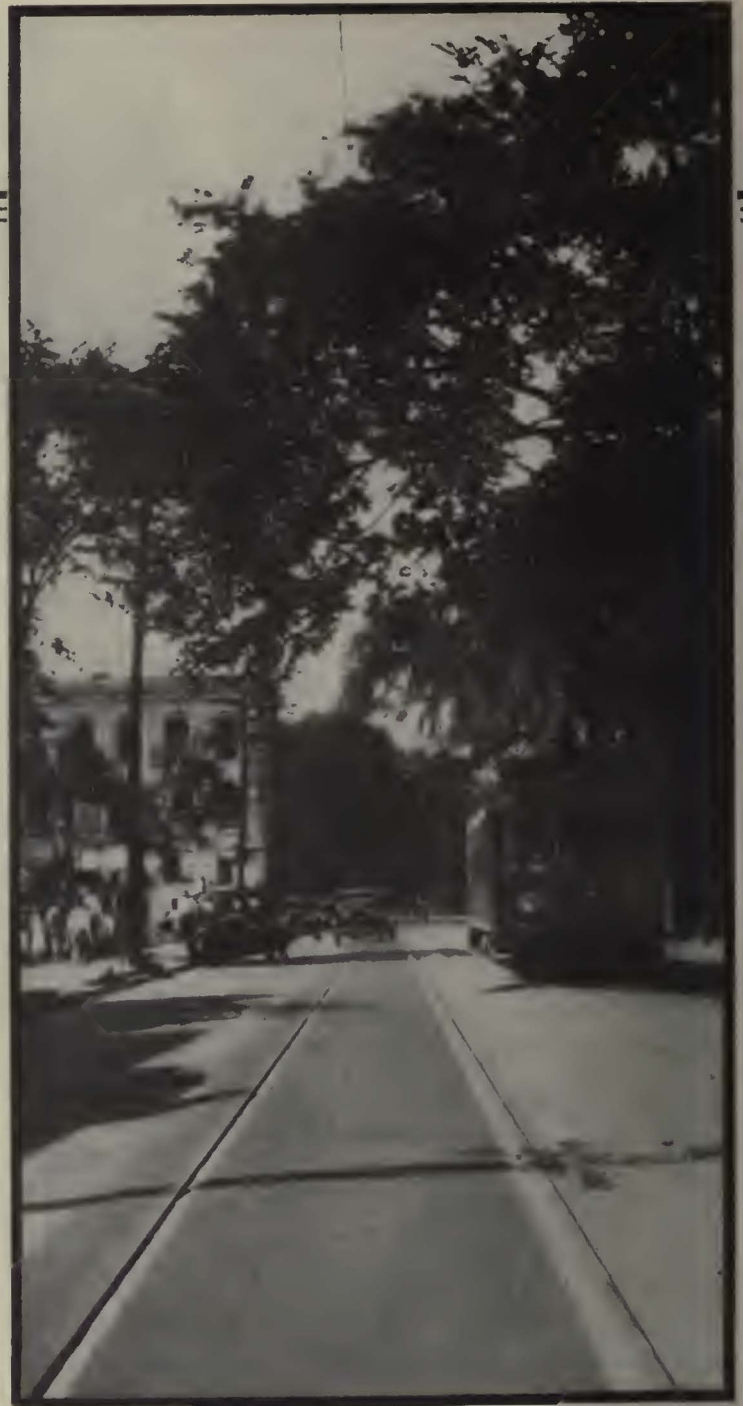
View on Whitehall Street, Atlanta showing standard track construction with Thermit welded rail joints.
