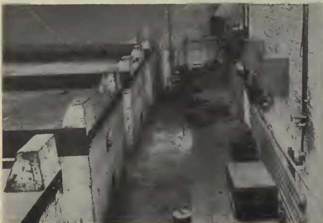
This arrangement of pits in the garage facilitates bus repairs
