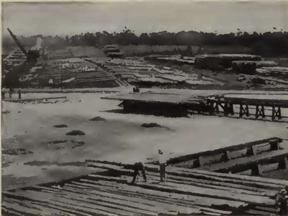
The production of Dixie Poles is an operation of major proportions
