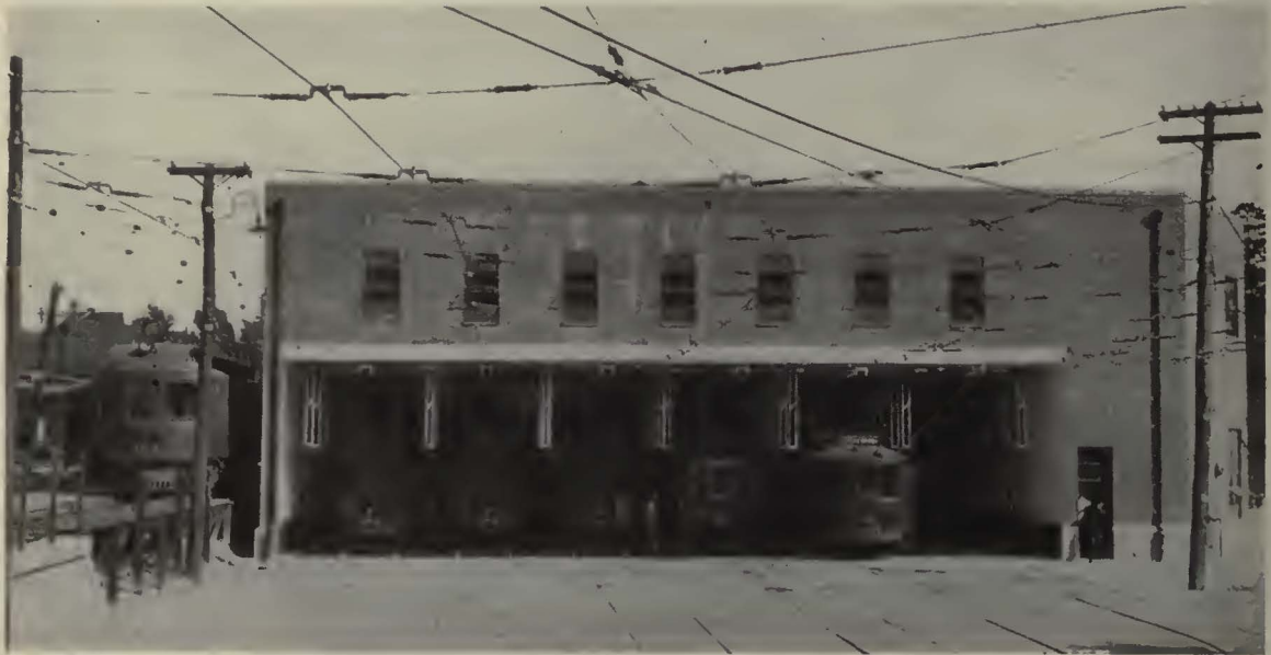
Precision methods are used to align the overhead properly with the track at carhouses, curves and intersections
