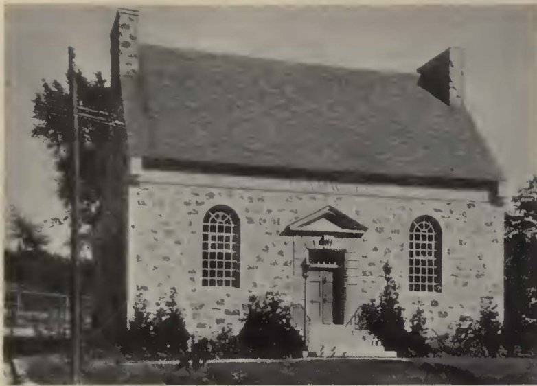
Queen Mary Road substation is built in a style commensurate with its residential surroundings
