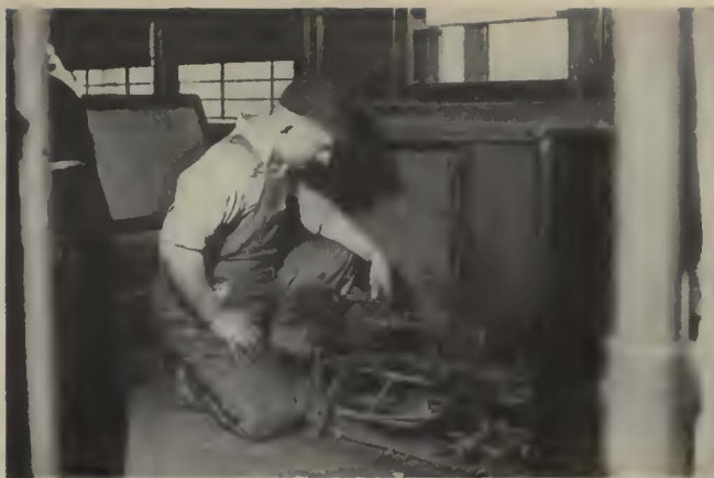
Door engines are removed from the car at the time of overhaul and dismantled for checking
