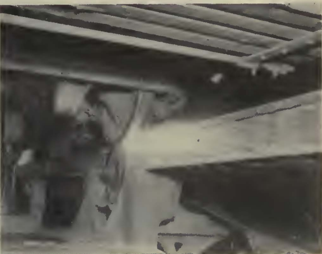
Wheels that show signs of wear on the flanges are ground while under the car
