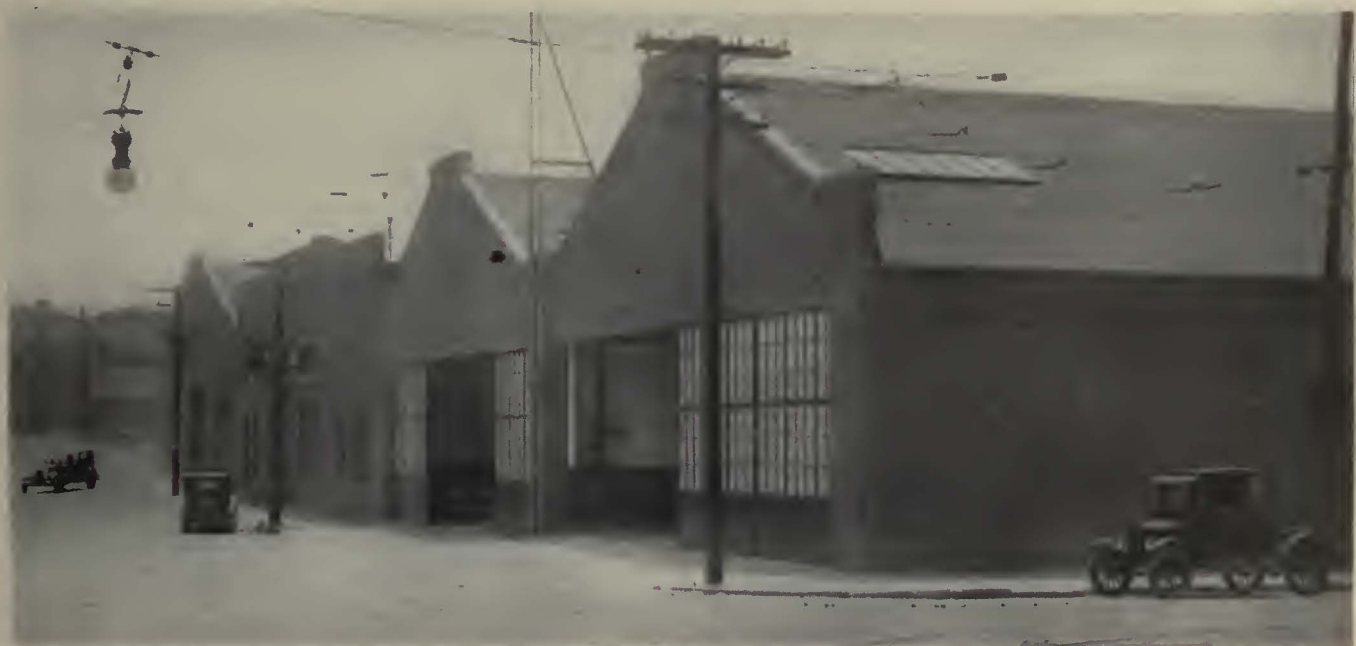
All buses in Atlanta are maintained at this centrally located garage
