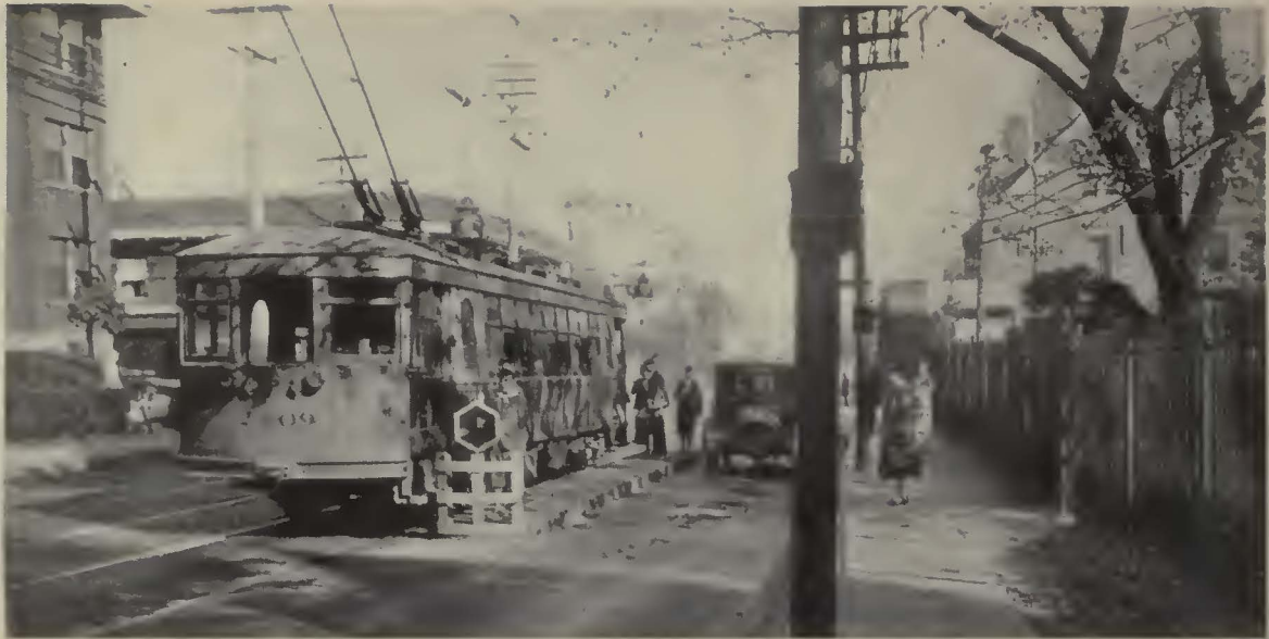
Loading platform in Cincinnati with sidewalk cut back to facilitate passage of vehicular traffic. Illumination is provided by lights suspended from span wires
