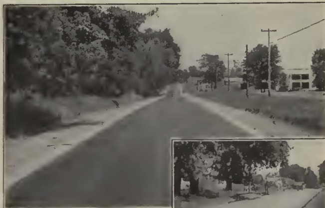
(Above) Completed brick resurfacing of worn concrete by Illinois State Highway Department on Route 4 south of Springfield. This gives the highest type highway at low cost.
