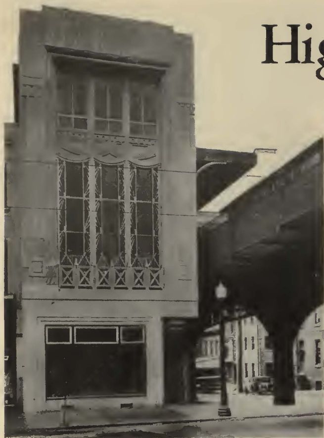
Main Street Façade of the New Norristown Terminal
