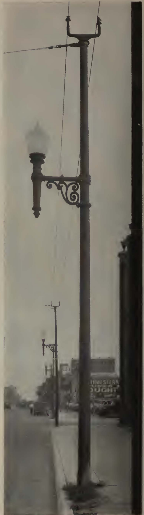
● Monotube Poles Installed in Denver, Colorado
