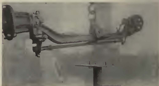
Hoisting axle to stand
