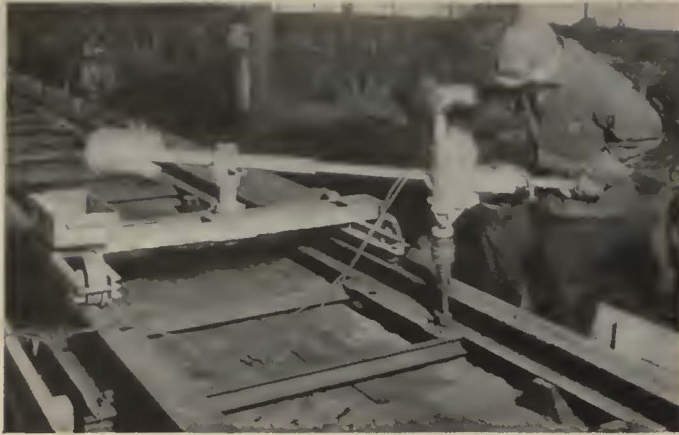
Bolt Tightener which has a special adjustable spring-tension over-running clutch to insure uniform tightness and tension on all rail clips. Only one man is needed to handle this device. Manufacturer: International Steel Tie Company, Cleveland, Ohio.
