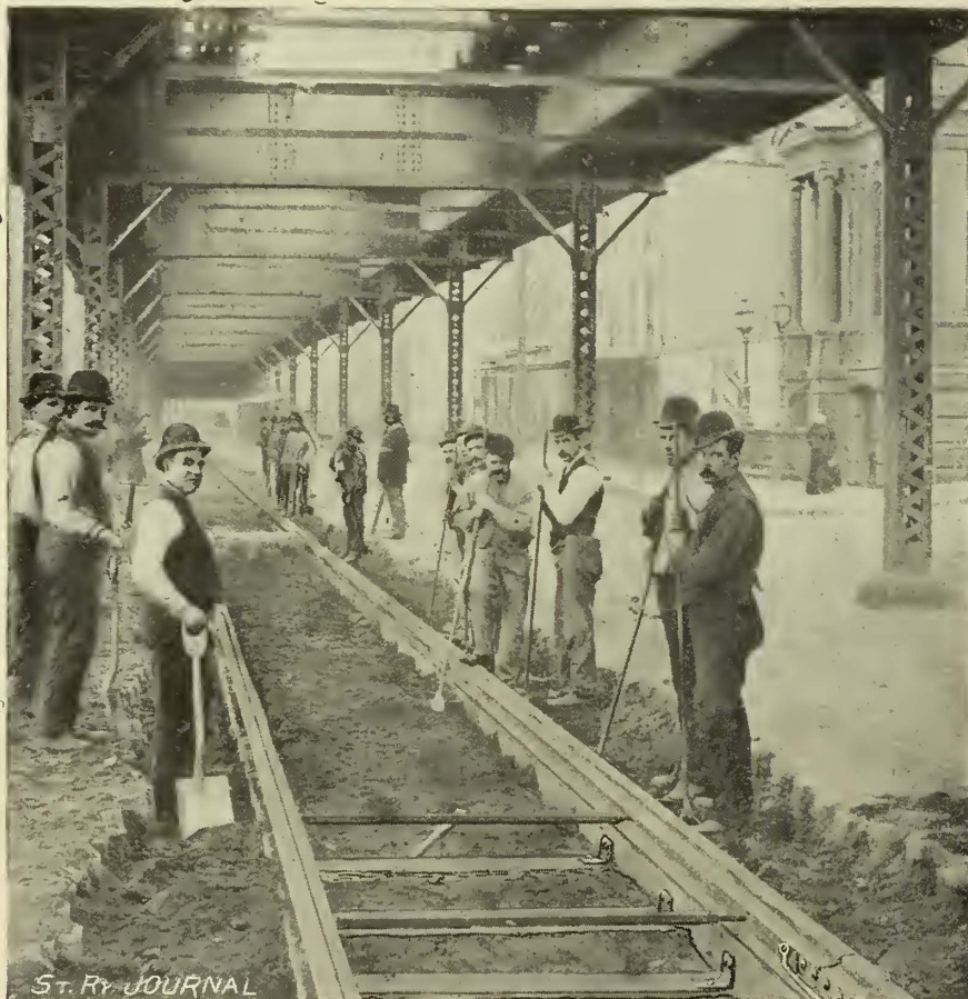
FIRST NEW YORK ELECTRIC ROAD—SECTION SHOWING TRACK CONSTRUCTION.
