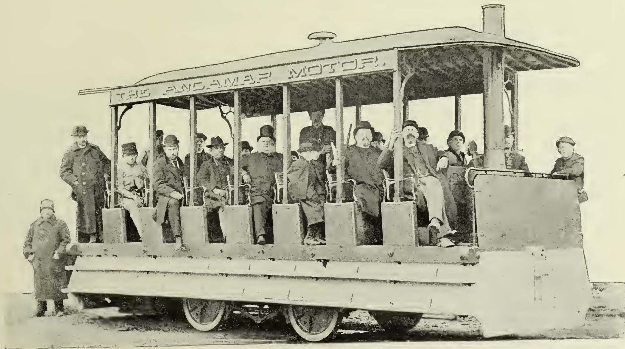
THE KINETIC STEAM MOTOR CAR FOR WEST CHICAGO STREET RAILWAY.
