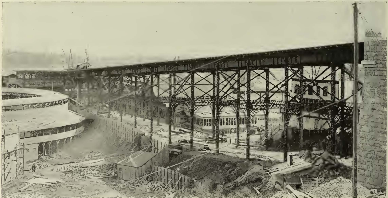
FIG. 3.—155TH STREET VIADUCT, NEW YORK—VIEW FROM WASHINGTON HEIGHTS.
