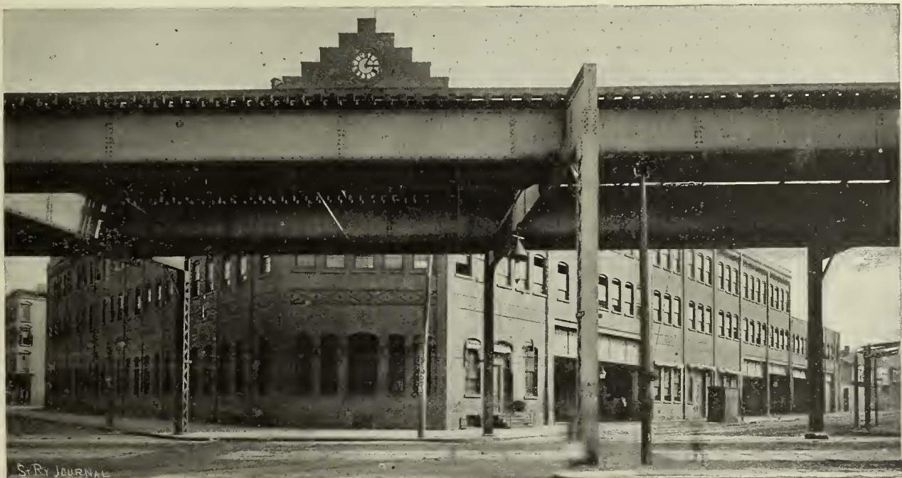
OFFICES AND PRINCIPAL DEPOT OF BROOKLYN CITY & NEWTOWN RAILROAD CO., BROOKLYN, N. Y.
