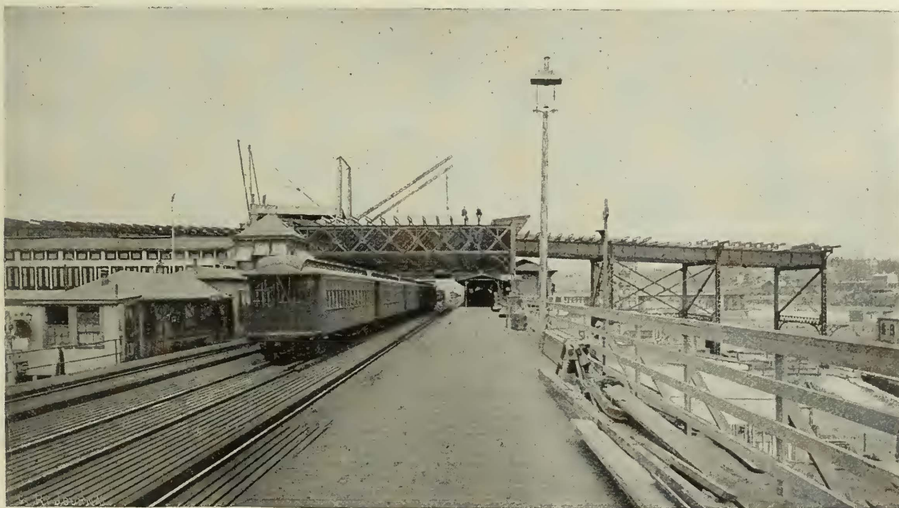
FIG. 1.—155TH STREET VIADUCT CROSSING ELEVATED RAILWAY AT 8TH AVENUE, NEW YORK.
