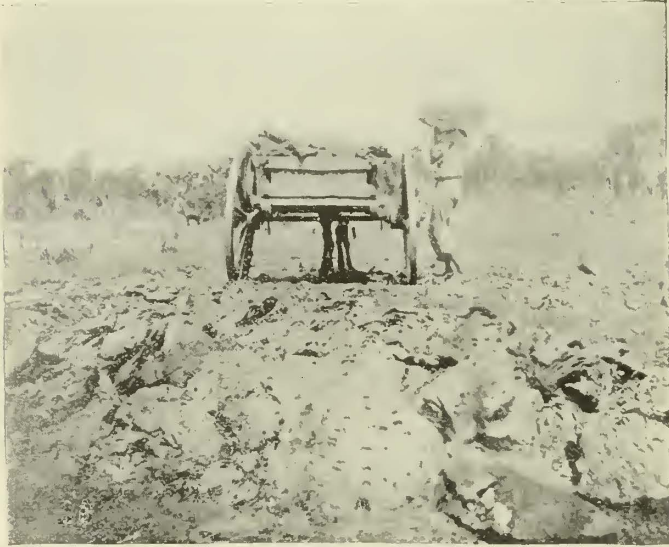
FIG. 2.—DIGGING AND LOADING ASPHALT.
