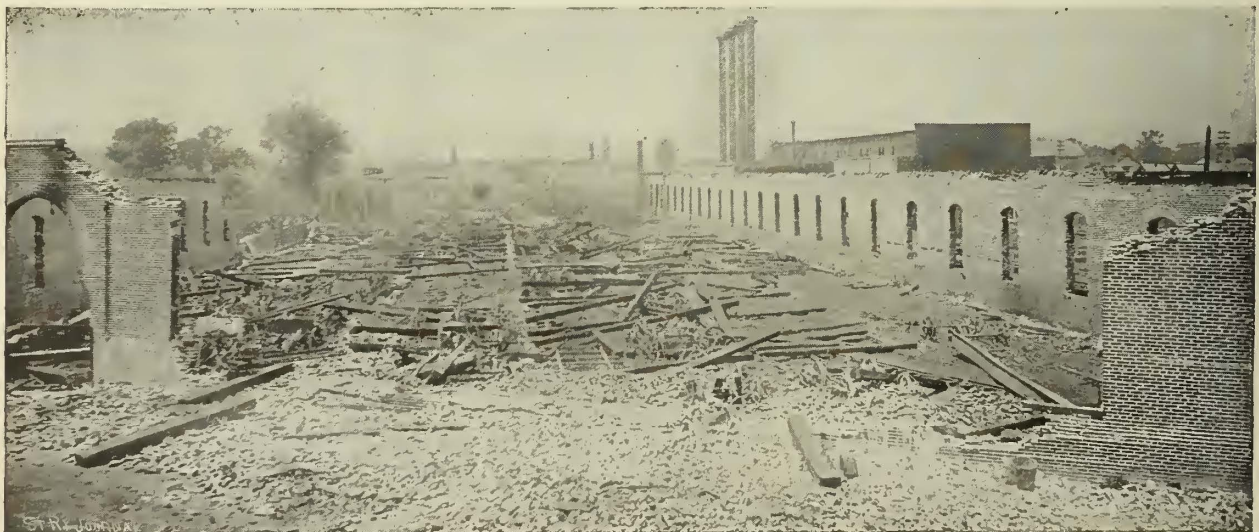
RUINS OF CAR HOUSE—ST. LOUIS & SUBURBAN STREET RAILWAY CO.
