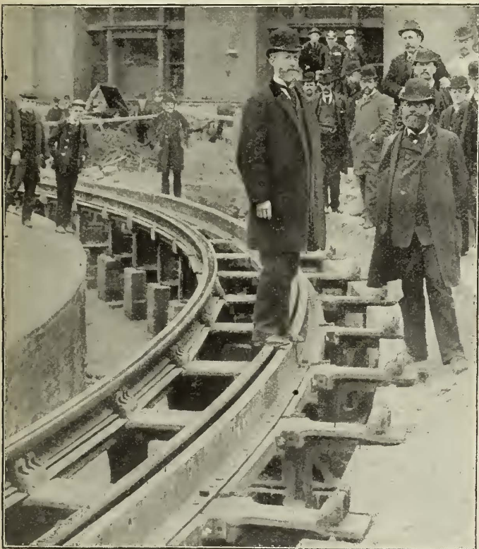
FIG. 2.—BOWLING GREEN LOOP DURING CONSTRUCTION—BROADWAY CABLE RAILWAY.
